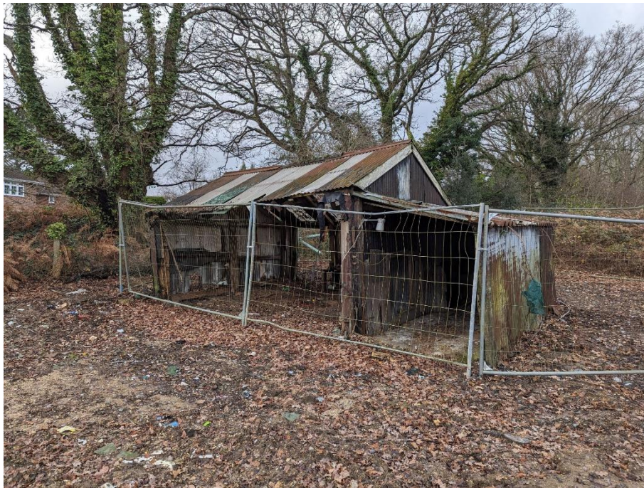
Figure 7. One of the outbuildings on site (taken December 2023).
