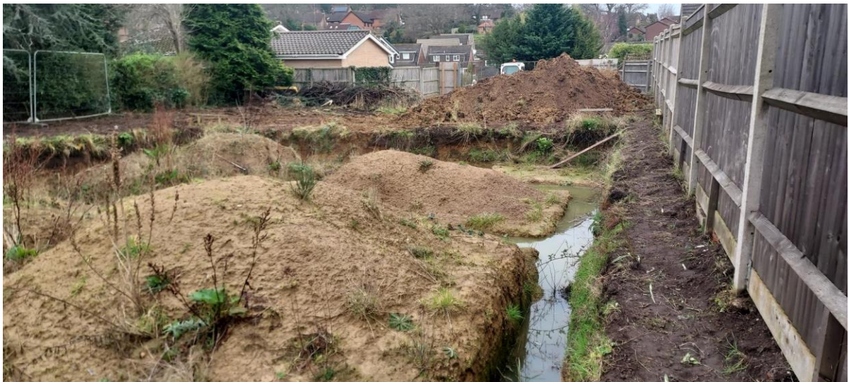
Photo 1: The footings of the new building
