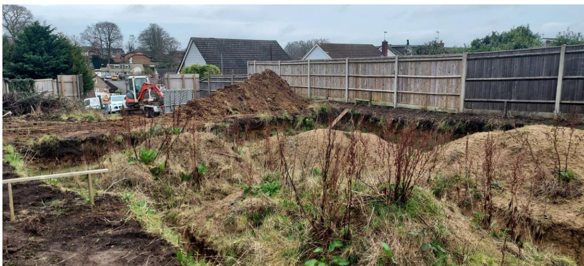
Photo 2: Piles of vegetated earth
