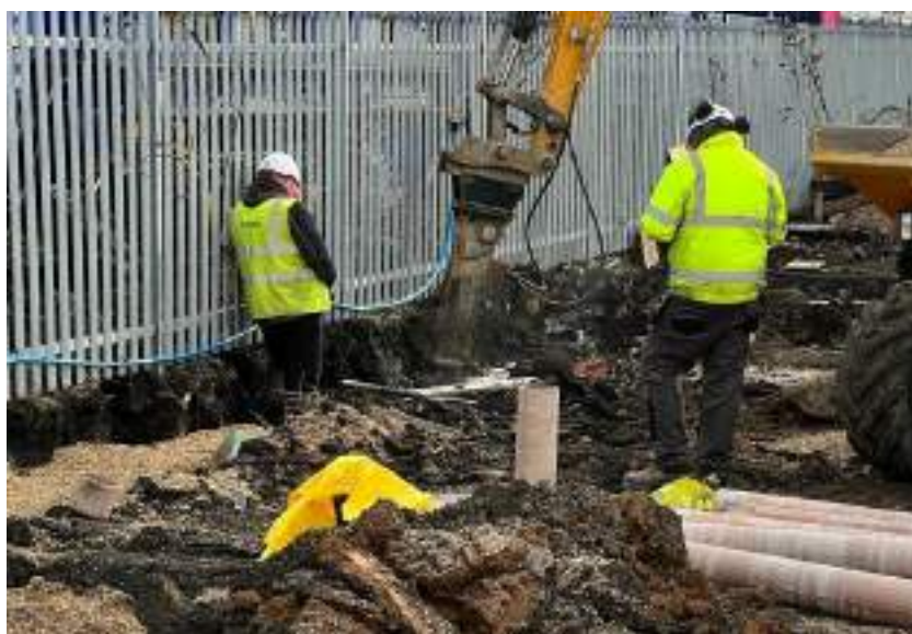
Figure 11 – Watching brief for redundant boreholes.
