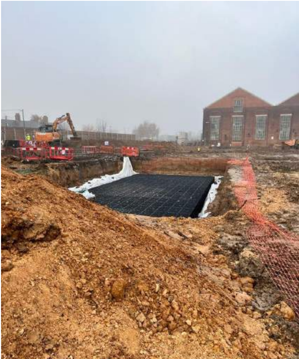
Figure 10 – Watching brief during drainage & service ducts.
