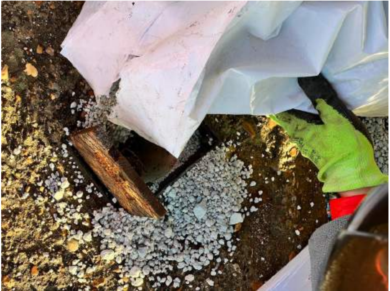
Figure 14 – Decommissioning boreholes.
