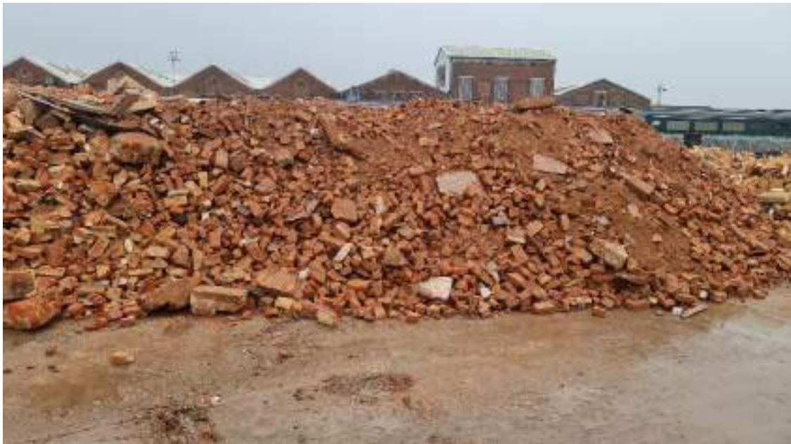
Figure 5 – Demolition Stockpile (prior to crushing).
