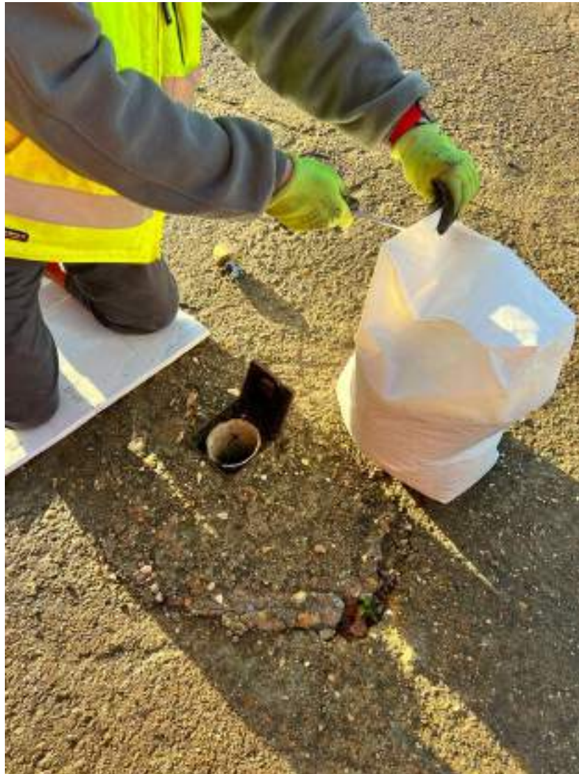
Figure 13 – Decommissioning boreholes.
