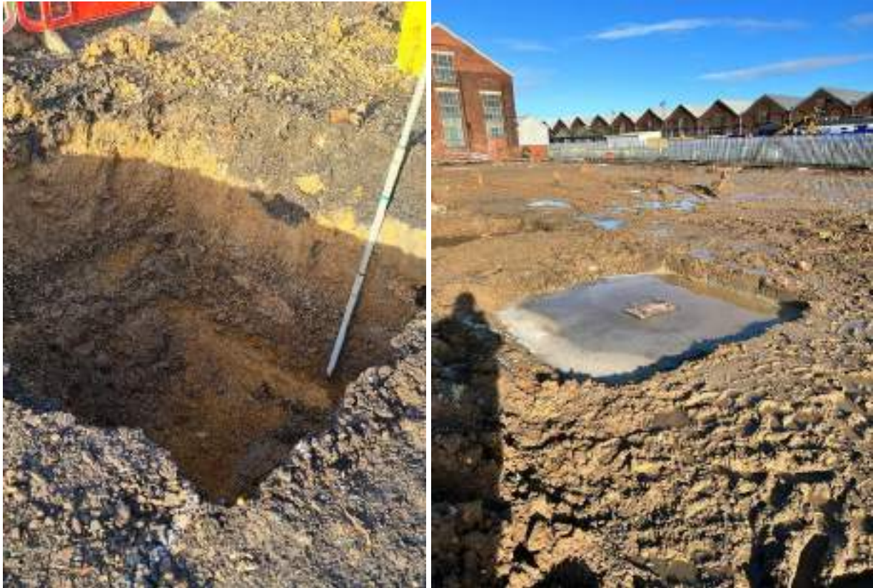
Figure 8 – Watching brief during groundworks.
