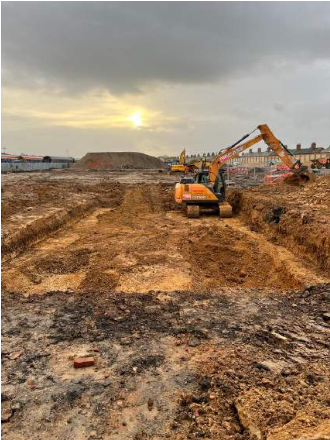
Figure 9 – Watching brief during groundworks.
