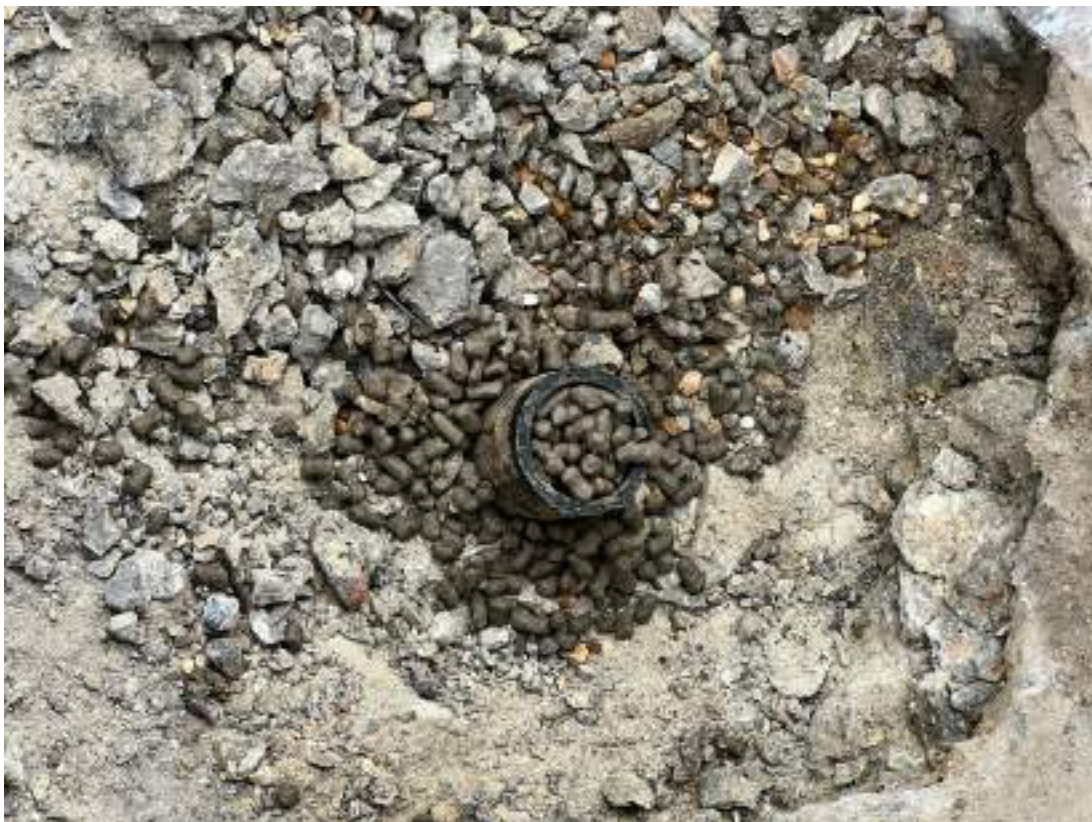
Figure 12 – Decommissioning boreholes.
