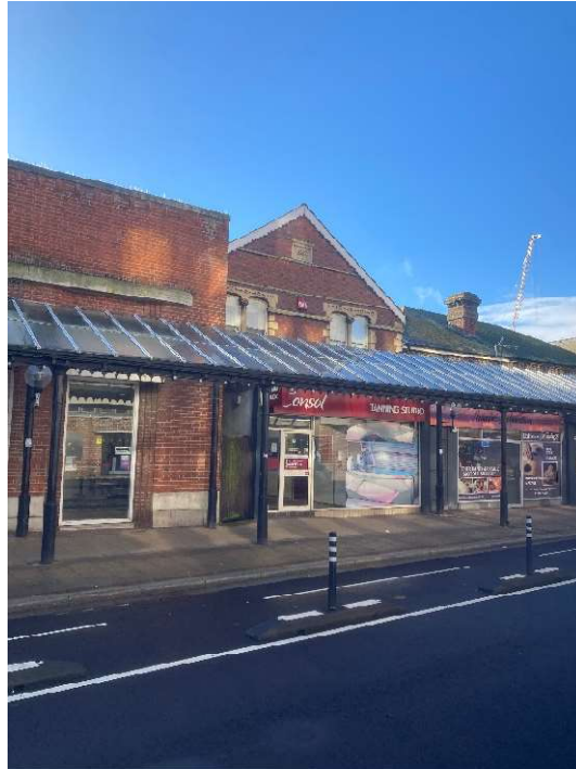
Fig. 1 – Photograph showing the front (north) elevation of 5 Leigh Road (centre).
