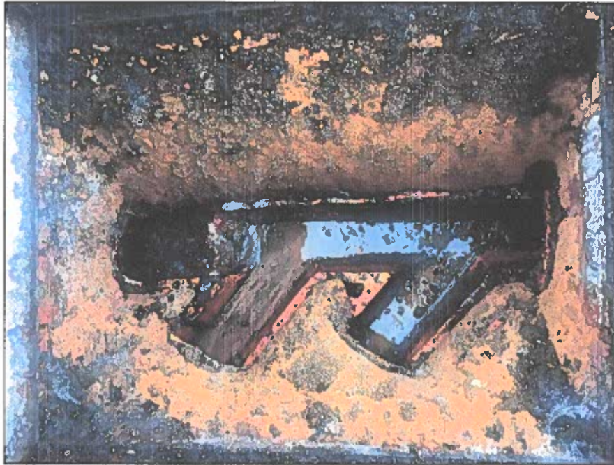
Photo: CABIN MH 1.JPG 18.07m, Finish node type, inspection chamber reference number: CABIN MH1
