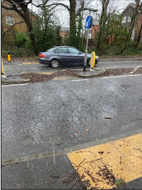
Photograph 3: Existing pedestrian infrastructure along Providence Hill
