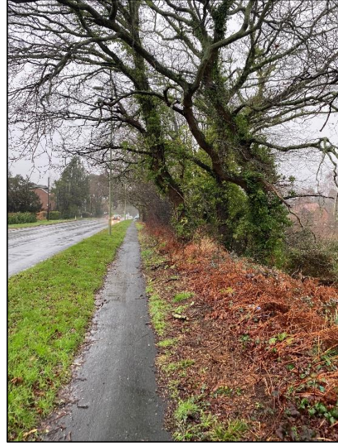
Photograph 4: Existing pedestrian infrastructure along Providence Hill
