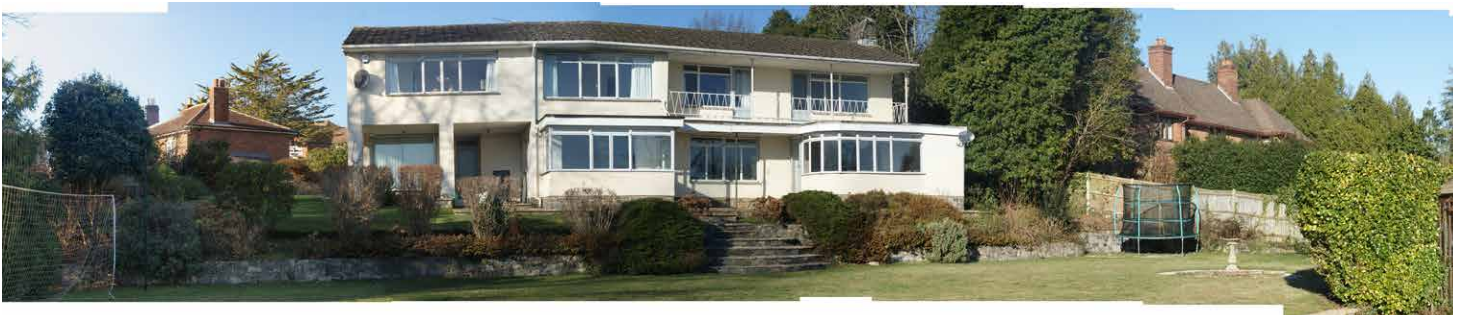
On-site View B - From north of the swimming pool, looking north at the existing dwelling, with the neighbouring dwellings visible to either side
