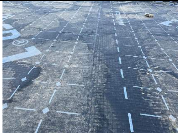
Plot 15. Overview of a hand welded membrane lap joint.
