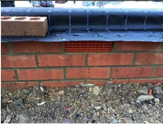
Air brick in place under the membrane at the time of our inspection.
