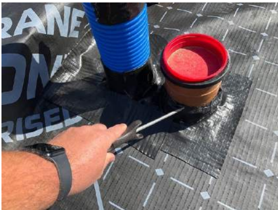
Plot 40. Pick testing to sealed pipe penetration's.
