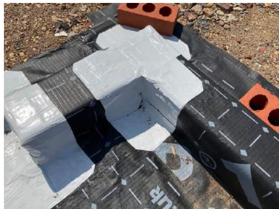
Plot 17. Typical corner detail sealed with SAGM.
