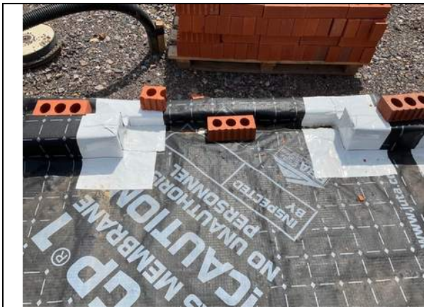
Plot 21. Threshold detail sealed using SAGM.
