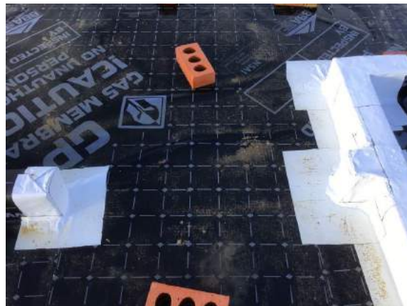
Sealed internal door threshold using SAGM.
