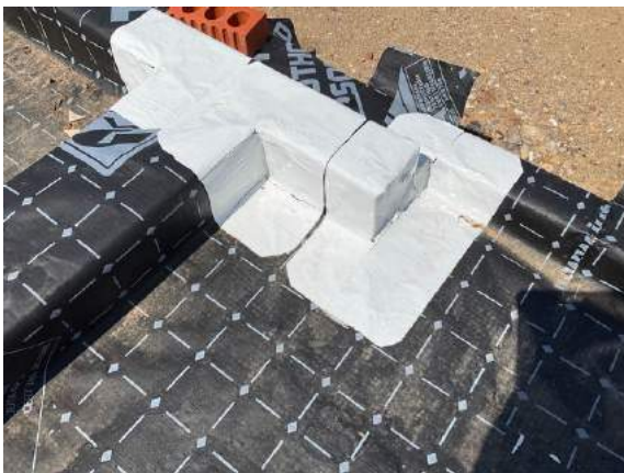
Plot 19. Corner and threshold details sealed with SAGM.
