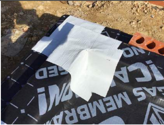
Typical corner seal using SAGM in plot 30.
