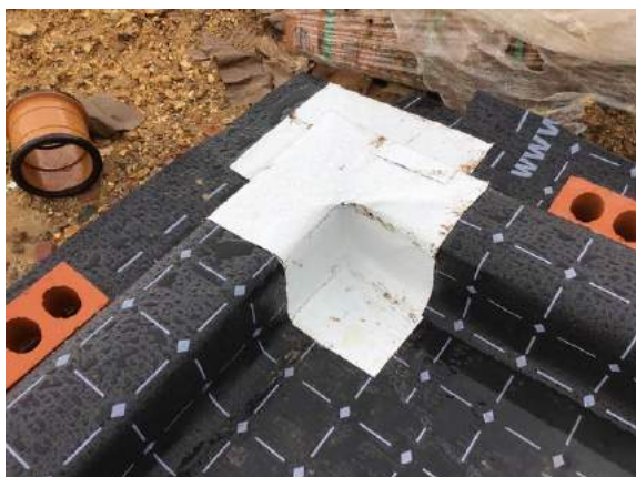
Typical corner seal using SAGM in plot 78.
