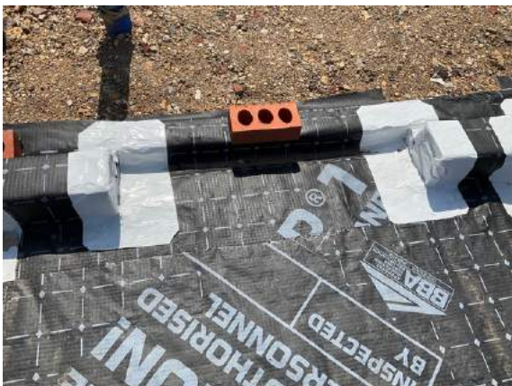
Plot 17. Threshold detail sealed with SAGM.
