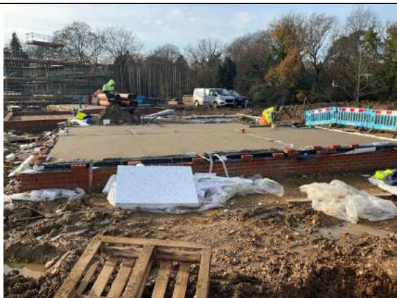
Overview of Plot 35 installed this week, but screeded prior to our visit.
