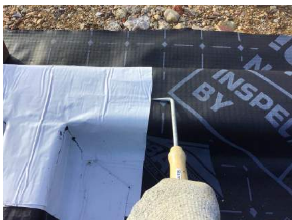
Pick testing all SAGM detailing in plot 57.
