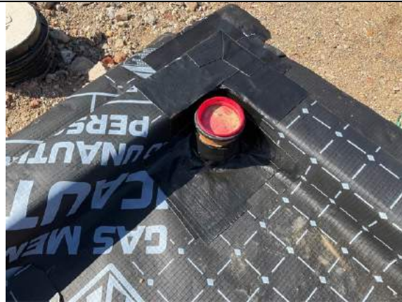
Plot 40. Multiple details corner and pipe entry sealed with SAGM.
