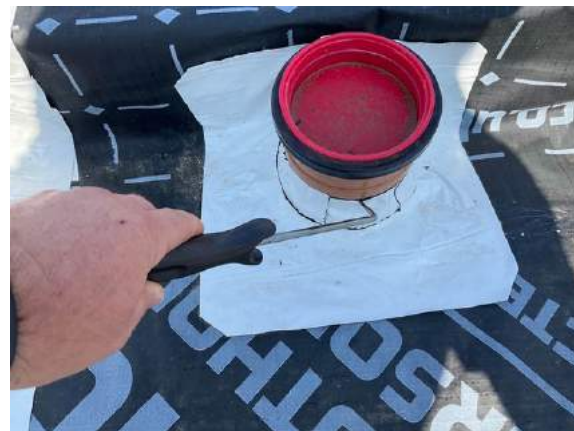
Plot 19. Pick test to sealed pipe entry.
