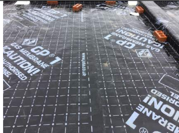
All membrane laps have been hand welded using a hot air gun and rolled using a neoprene roller in plot 68.
