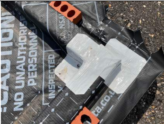
Plot 22. Internal & external corner details sealed with SAGM.
