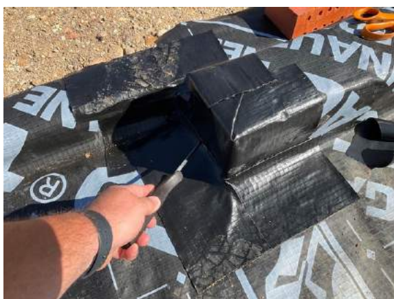
Plot 39. Pick testing to sealed threshold detail.
