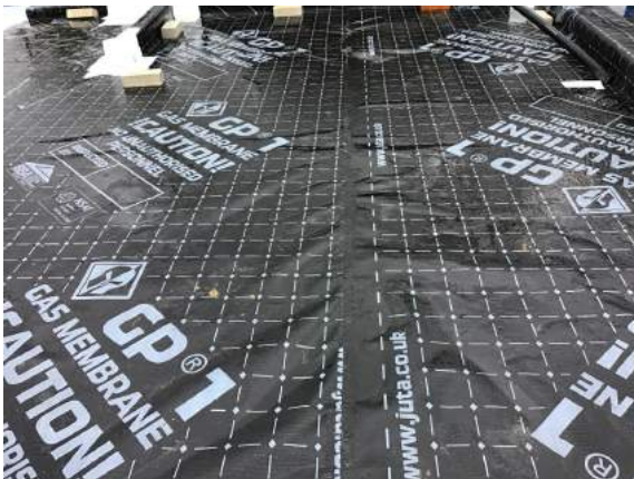
All membrane laps have been hand welded using a hot air gun and rolled using a neoprene roller in plot 72.
