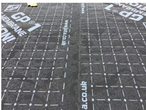
Hand welded membrane lap in plot 31.
