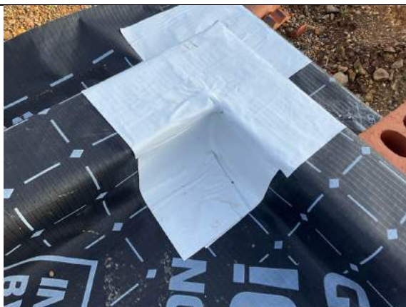
Plot 34. Typical corner details sealed using SAGM.
