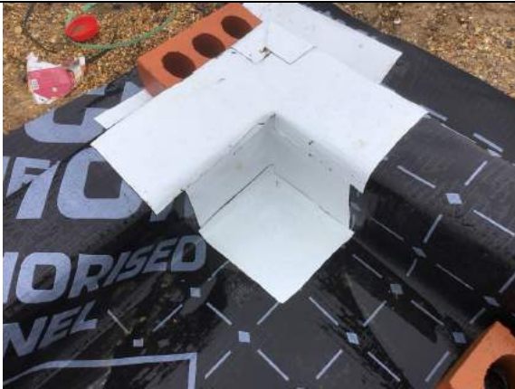
Typical corner seal using SAGM in plots 73-76.
