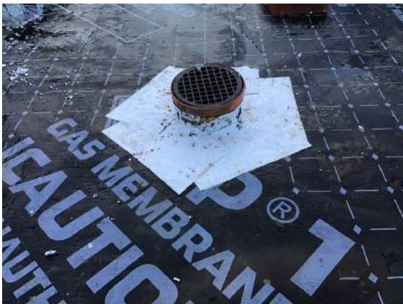
Sealed pipe penetration using SAGM in apartment plots 62-66.
