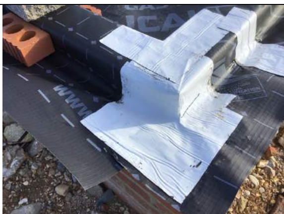
Typical corner seal using SAGM in plot 56.
