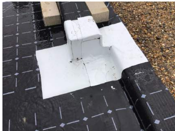
Sealed door threshold detail using SAGM in plot 81.
