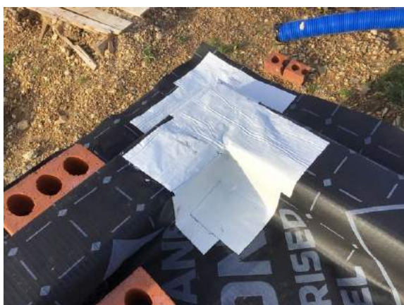
Typical corner seal using SAGM in plot 69.
