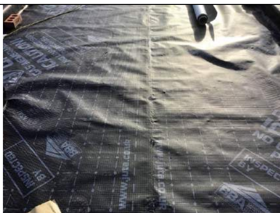
Hand welded membrane lap in plot 69.
