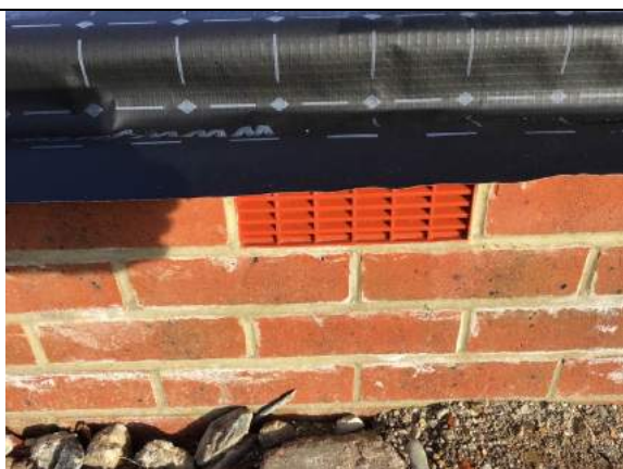
Air brick in place at the time of our inspection under the membrane to plot 60.
