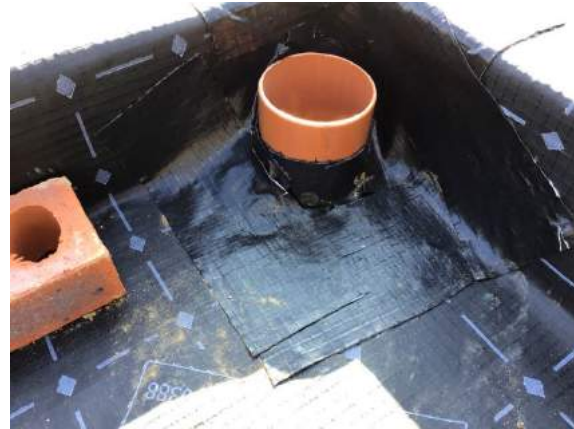
Typical pipe penetration seal using SAGM in plot 29.
