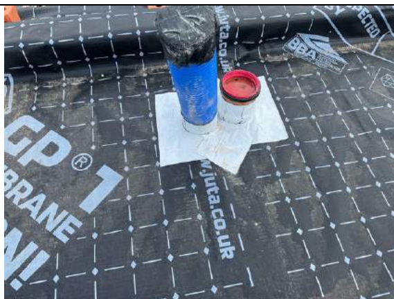
Plot 24. Typical dual pipe penetration's sealed using SAGM.
