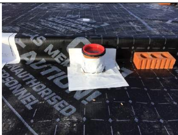
Typical pipe penetration seal using SAGM in plot 60.
