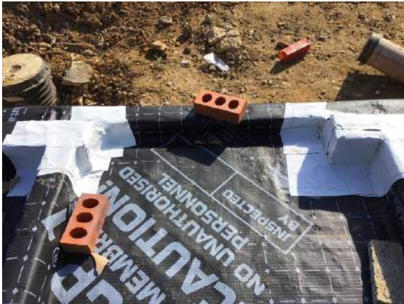
Sealed door threshold detail using SAGM in plot 30.
