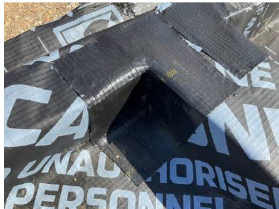
Plot 40. Typical corner detail sealed using SAGM.
