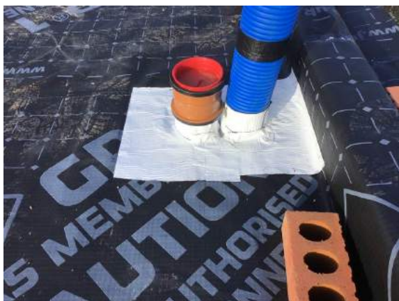
Typical double pipe penetration seal using SAGM in plot 58.
