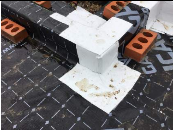
Typical corner seal using SAGM in plot 83.
