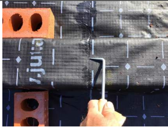
Pick testing all hand welded membrane laps in plot 30.
