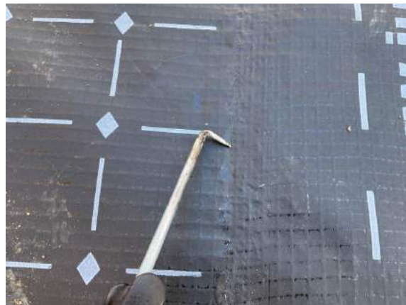
Plot 27. Pick testing along all hand welded membrane lap joints.
