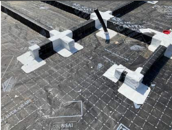
Plot 18. Multiple details sealed using SAGM.
