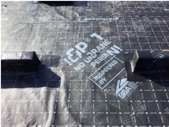
Sealed internal door threshold using SAGM in plot 29.
