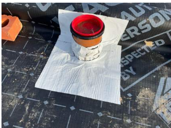
Plot 34. Typical pipe penetration's sealed with SAGM.
