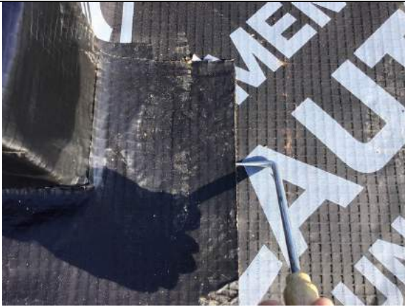
Pick testing all SAGM detailing in plot 28.
