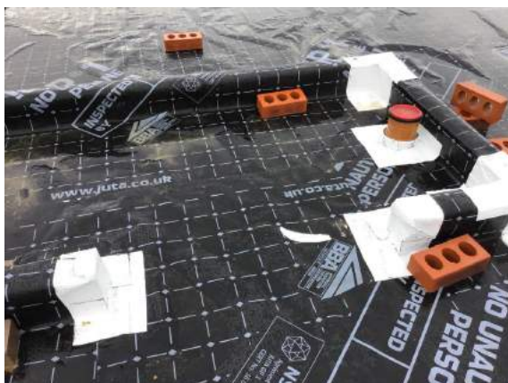
Typical internal door threshold seal using SAGM in plot 36.
