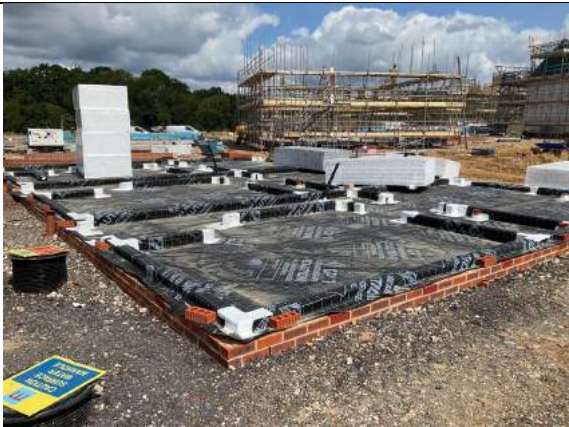
Overview of the full footprint installation to Plots 12-13-14.
