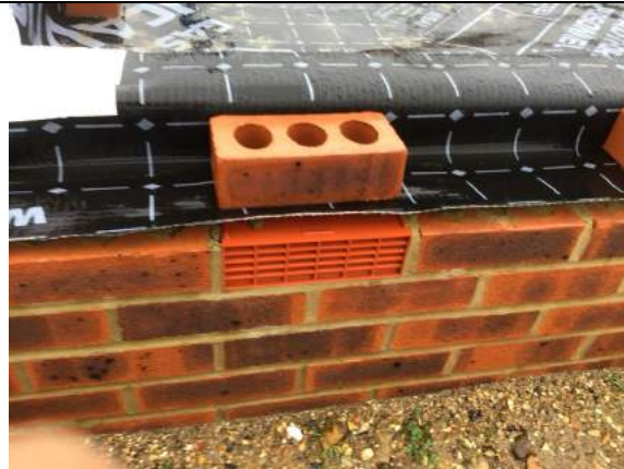
Air brick under the membrane at the time of our inspection to plots 73-76.
