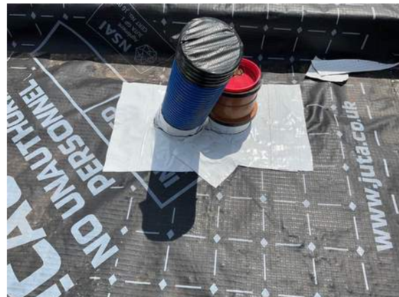
Plot 20. Typical pipe penetration's sealed with SAGM.
