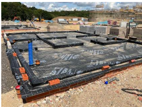
Overview of the full footprint installation to Plot 25.
