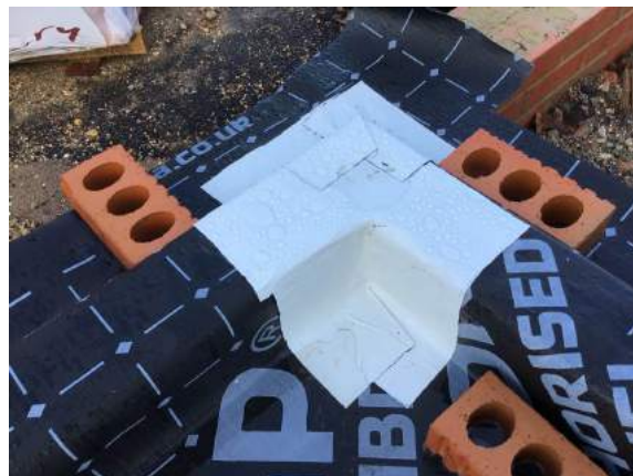
Typical corner seal using SAGM in plot 59.
