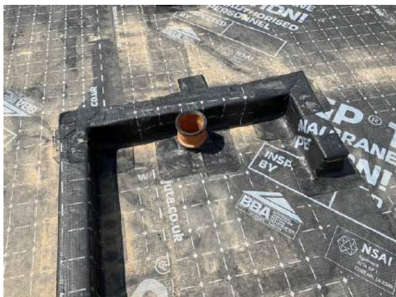
Plot 25. Multiple corner details and pipe entry sealed with SAGM.
