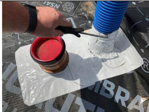
Plot 22. Pick testing upon sealed pipe penetration's.
