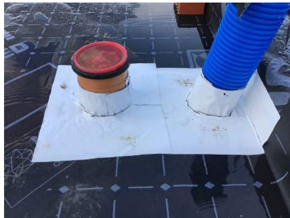
Typical double pipe penetration seal using SAGM in plot 59.
