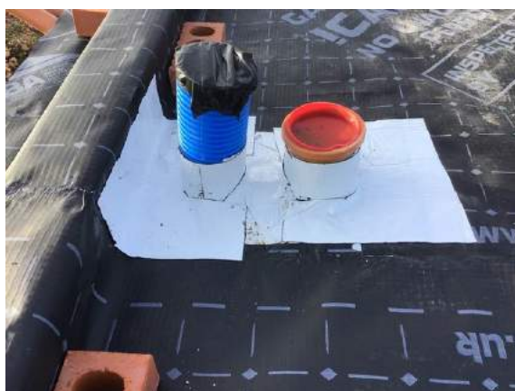
Typical double pipe penetration seal using SAGM in plot 69.
