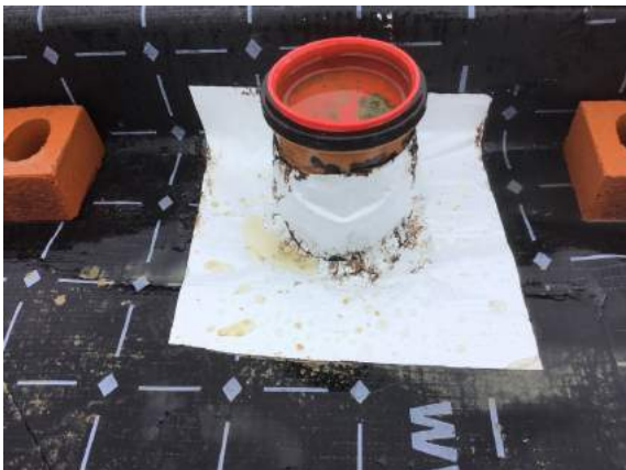
Typical pipe penetration seal using SAGM in plot 67.
