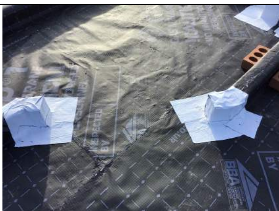
Sealed internal door threshold seal using SAGM in plot 56.
