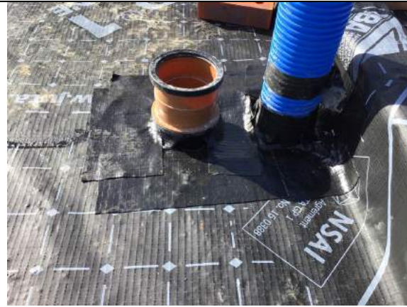
Typical double pipe penetration seal using SAGM in plot 28.
