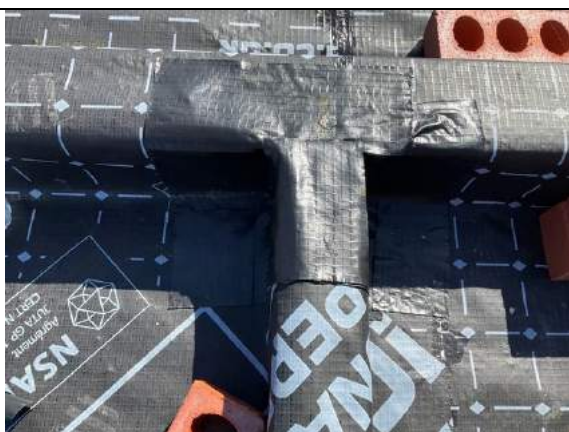
Plot 38. Typical corner details sealed using SAGM.
