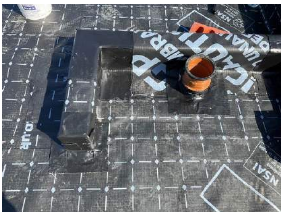
Plot 39. Multiple details sealed using SAGM.
