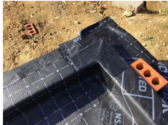
Sealed corner detail using SAGM in plot 29.
