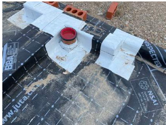
Plot 16. Corner, threshold & pipe entry sealed with SAGM.
