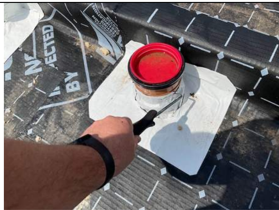
Plot 21. Pick testing to sealed pipe entry.
