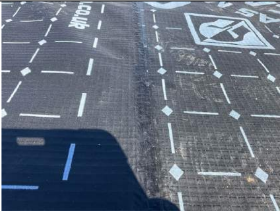
Plot 40. Overview of a hand welded membrane lap joint.
