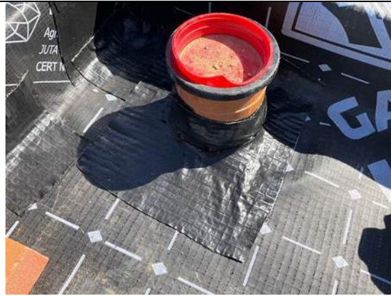
Plot 41. Typical pipe penetration sealed with SAGM.
