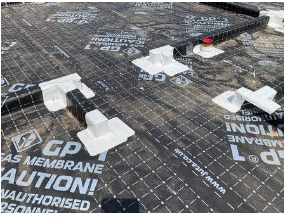
Plot 20. Multiple corner details sealed with SAGM.
