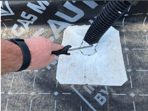
Plot 15. Pick test to sealed pipe entry.
