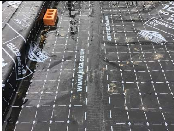
All membrane laps have been hand welded using a hot air gun and rolled using a neoprene roller in plot 83.
