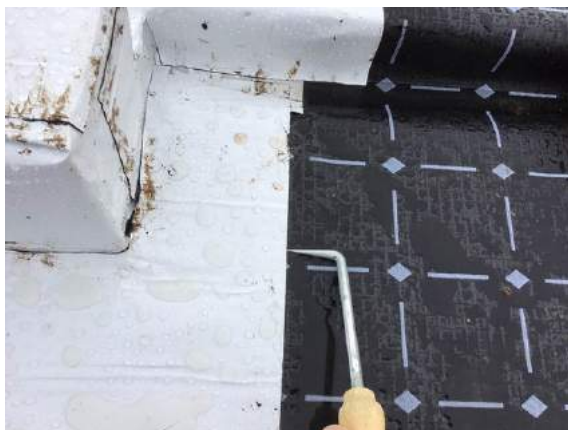
Pick testing all SAGM in plot 78.
