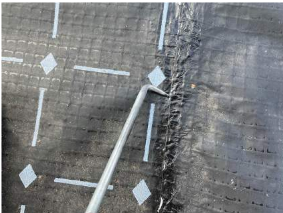
Plot 23. Pick test to hand welded membrane lap joint.
