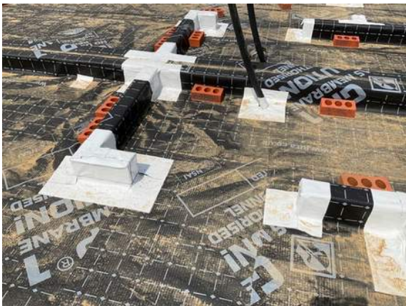
Plot 52. Multiple corner details & pipe entry sealed using SAGM.
