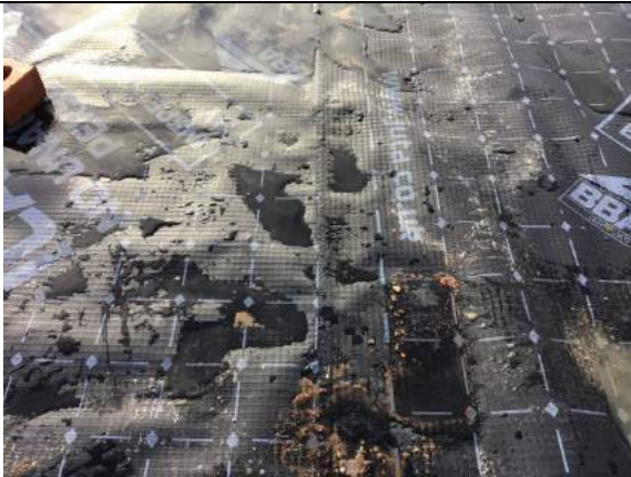
Typical hand welded membrane lap.
