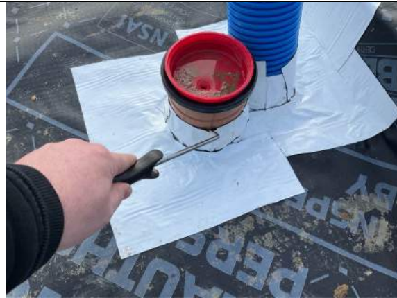
Plot 34. Pick testing upon sealed pipe penetration's.
