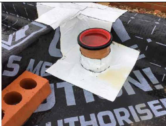
Typical pipe penetration and corner seal using SAGM in plot 77.
