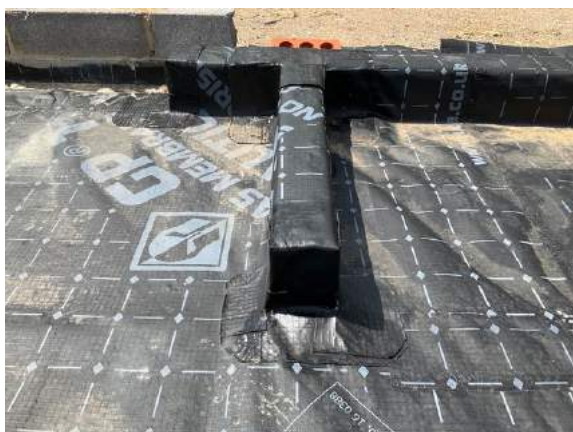
Plot 26. Corner details sealed with SAGM.
