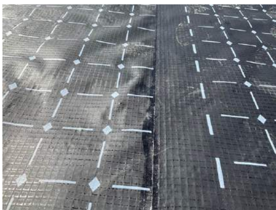
Plot 39. Overview of a hand welded membrane lap joint.
