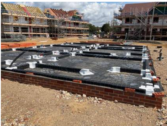
Overview of the full footprint installation to Plots 17-18-19.
