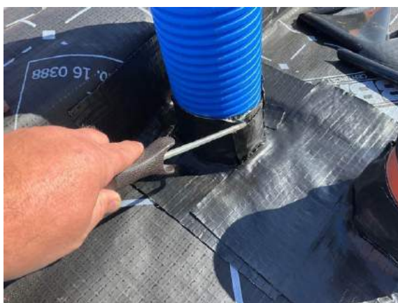
Plot 39. Pick testing to sealed pipe penetration's.
