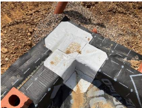
Plot 51. Internal & external corner details sealed with SAGM.
