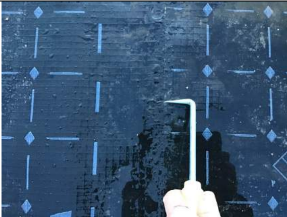
Pick testing all hand welded membrane laps in apartment plots 62-66.
