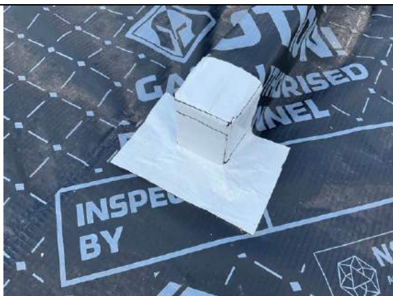
Plot 24. Internal wall corners sealed with SAGM.
