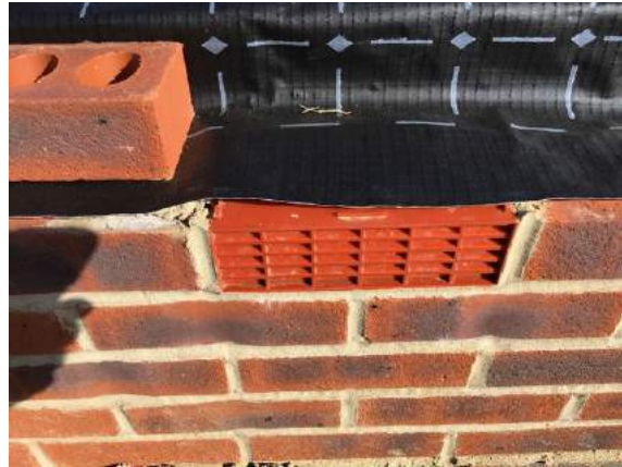
Air brick in place under the membrane to plots 28,29 & 30.
