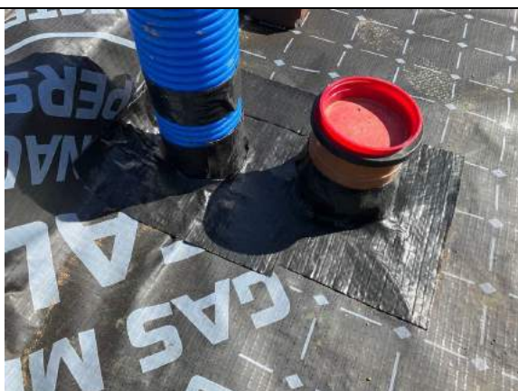
Plot 38. Typical pipe penetration's sealed using SAGM.
