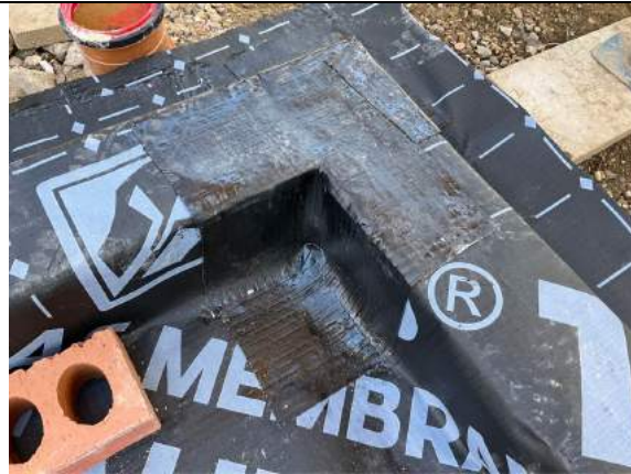
Plot 27. Typical corner detail sealed using SAGM.
