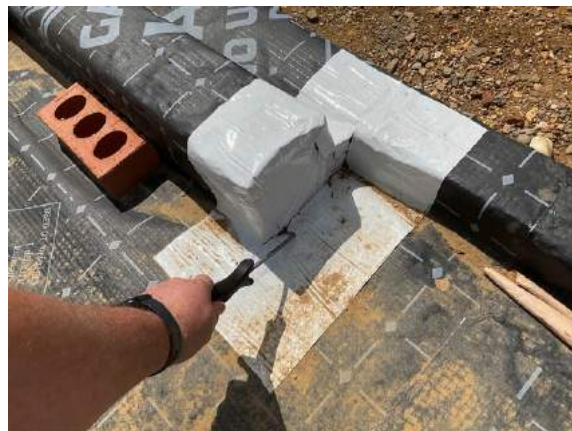
Plot 51. Pick test to sealed threshold detail.
