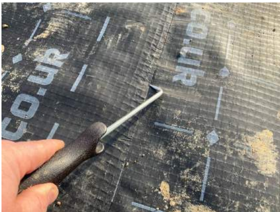
Plot 34. Pick & Probe testing along all hand welded lap joints.
