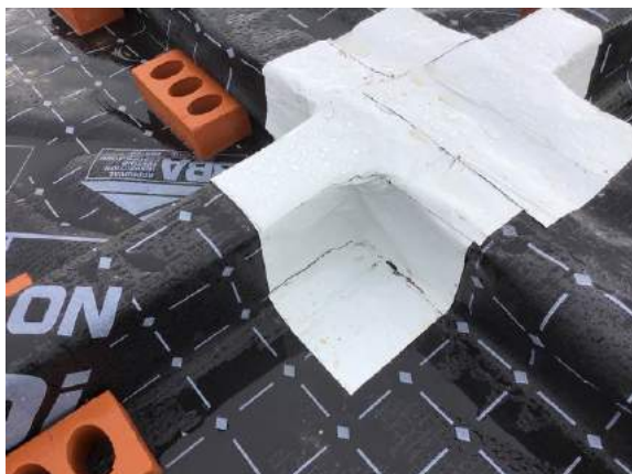
Typical corner seal using SAGM in plot 77.
