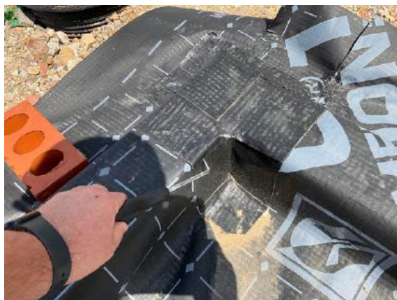
Plot 25. Pick testing to sealed corner detail.
