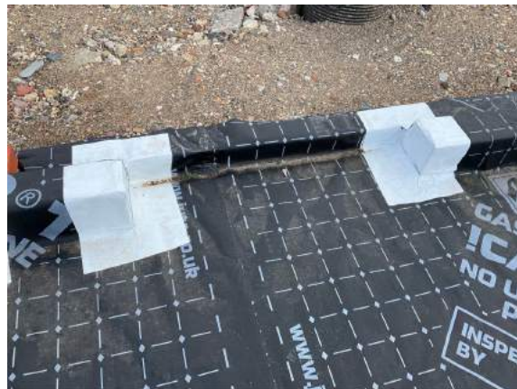
Plot 23. Threshold detail sealed with SAGM.
