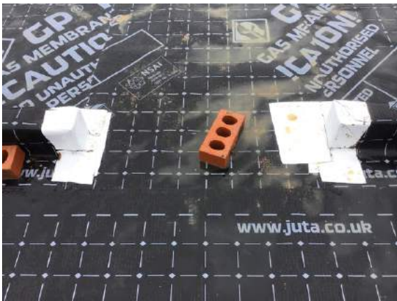
Sealed internal door threshold using SAGM in plot 68.
