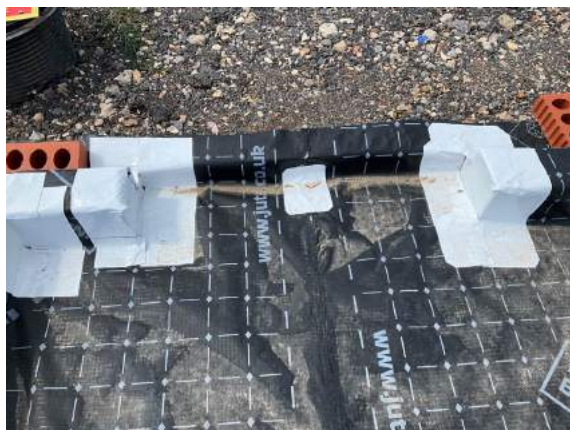
Plot 14. Threshold detail sealed with SAGM.
