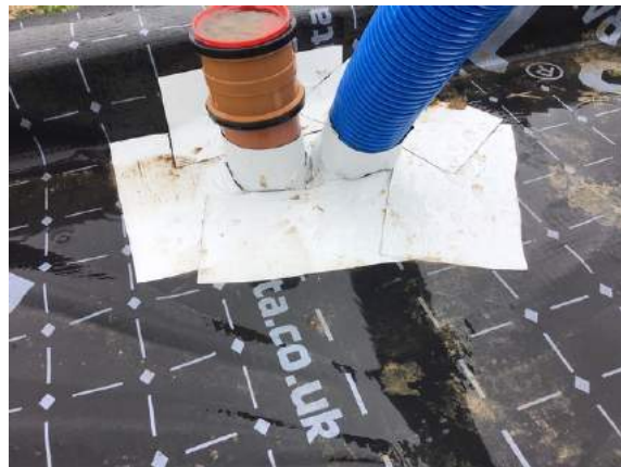
Typical double pipe penetration seal using SAGM in plot 84.
