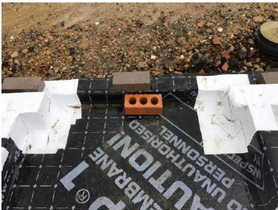
Sealed door threshold detail using SAGM in plot 84.
