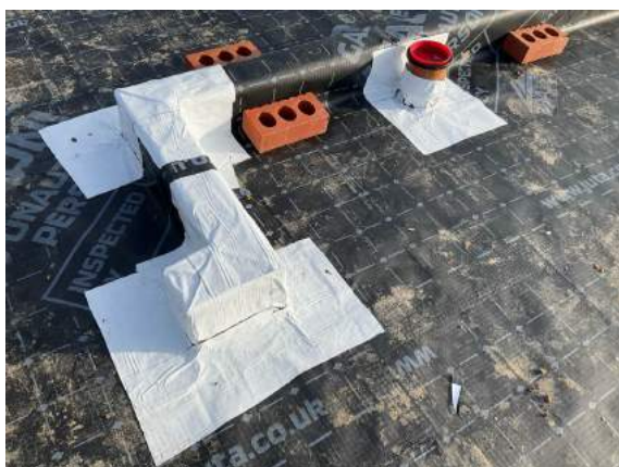
Plot 34. Multiple corner and pipe entry details sealed using SAGM.
