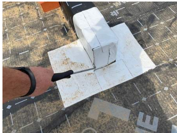
Plot 52. Pick test to internal wall corner details.
