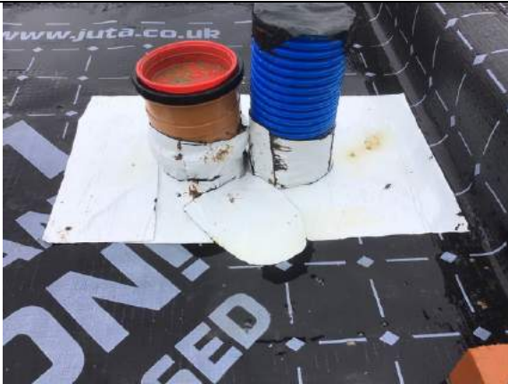
Typical double pipe penetration seal using SAGM in plot 68.
