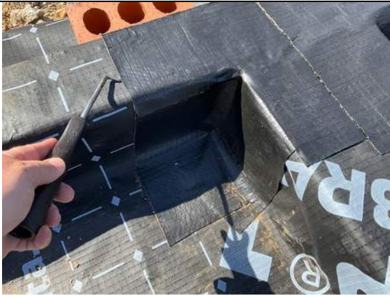
Plot 41. Pick testing upon sealed corner detail.
