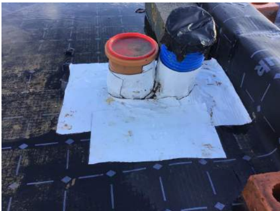
Typical double pipe penetration seal using SAGM.
