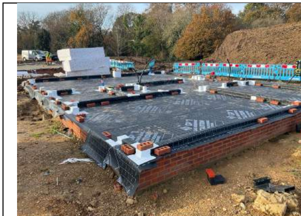
Overview of the installation of Juta GP1 Gas Barrier to Plot 34.
