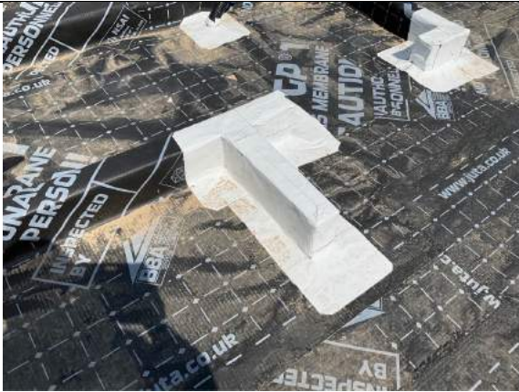
Plot 12. Corner details sealed with SAGM.
