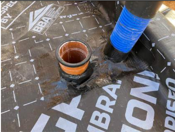
Plot 27. Typical pipe penetration's sealed with SAGM.
