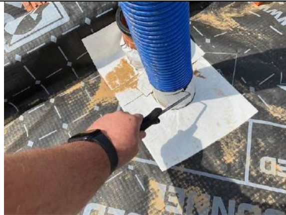
Plot 50. Pick test to sealed pipe entry's.
