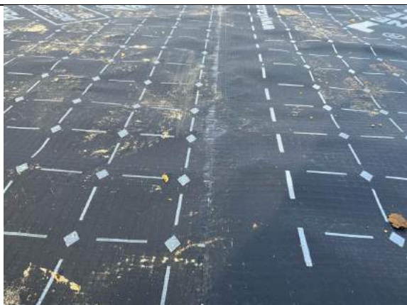
Plot 34. Overview along a hand welded membrane lap joint.
