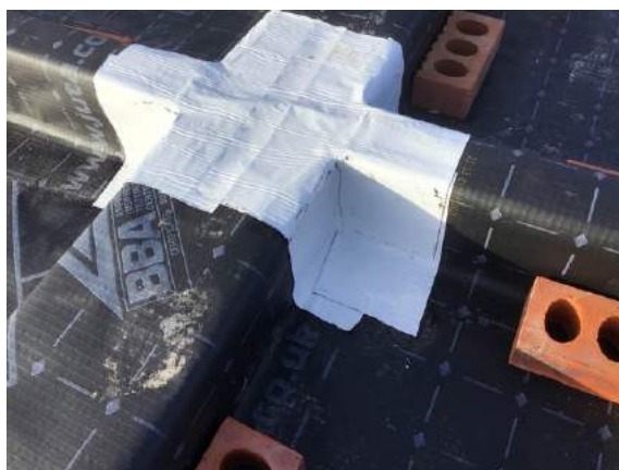
Typical corner seal using SAGM in plot 61.
