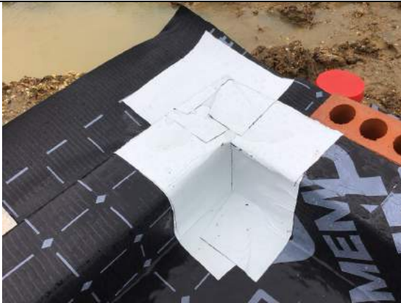
Typical corner seal using SAGM in plot 70.
