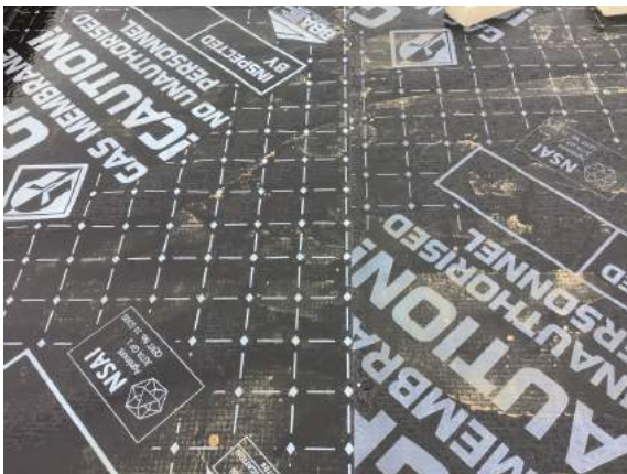
All membrane laps have been hand welded using a hot air gun and rolled using a neoprene roller in plots 73-76.
