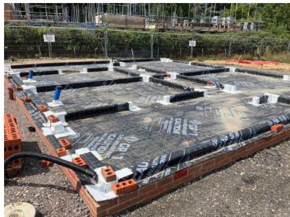
Overview of the full footprint installation to Plots 20-21.
