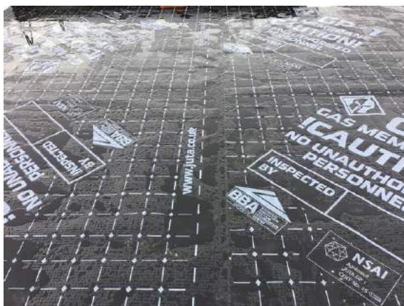
Typical hand welded membrane lap in plot 78.
