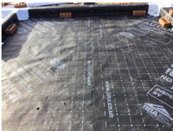
All membrane laps have been hand welded using a hot air gun and rolled using a neoprene roller in plot 58.
