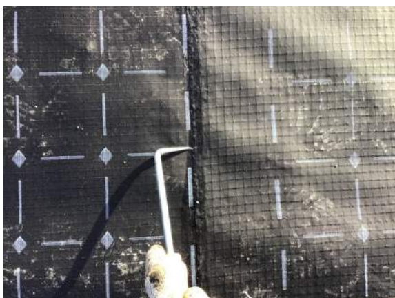
Pick testing all hand welded membrane laps in plot 61.
