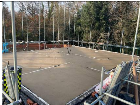
Overview of Plot 32 installed this week, but screeded prior to our visit.
