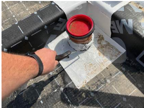
Plot 13. Pick testing to sealed pipe entry.
