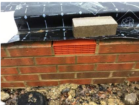
Air brick in place under the membrane to all inspected plots during our visit.
