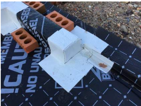
Typical door threshold detail, sealed using SAGM in plot 59.
