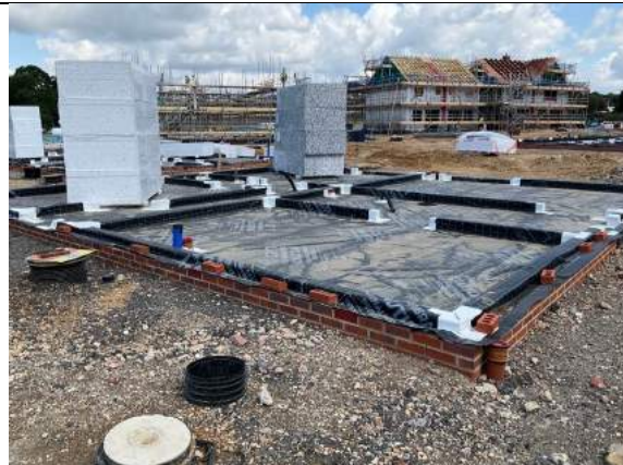
Overview of the full footprint installation to Plots 15-16.
