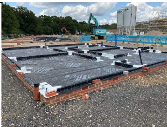
Overview of the full footprint installation to Plots 23-24.
