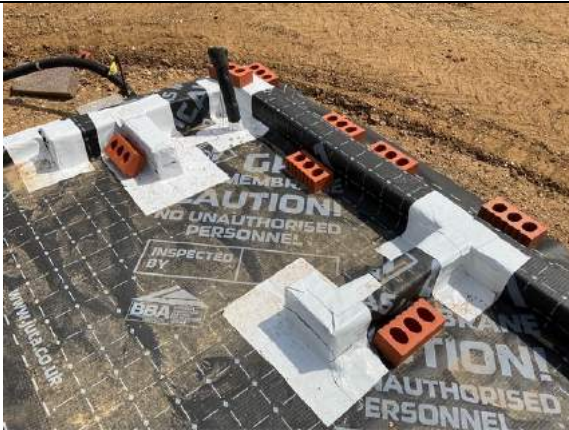
Plot 50. Multiple corner and pipe entry sealed using.
