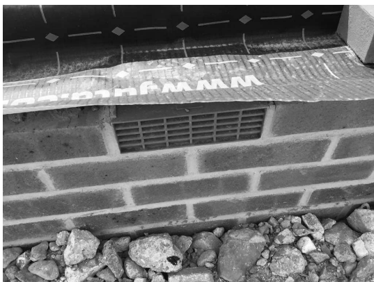
Air brick in place under the membrane during our inspection to plot 26.
