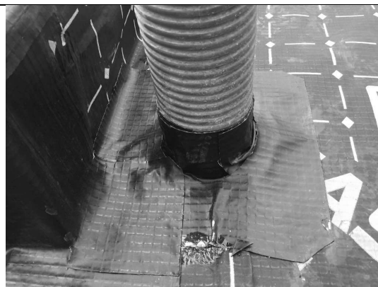
Typical pipe penetration seal using SAGM to plot 7.
