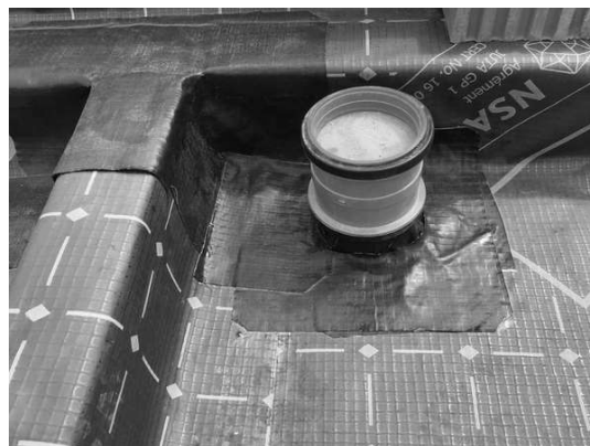
Typical pipe penetration seal using SAGM to plot 43.
