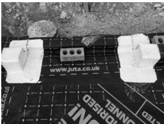
Typical door threshold seal using SAGM to plot 4.
