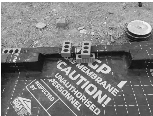
Typical door threshold seal using SAGM to plot 44.
