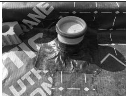
Typical pipe penetration seal using SAGM to plot 6.
