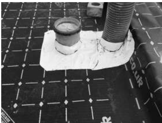
Typical double pipe penetration seal using SAGM to plot 3.
