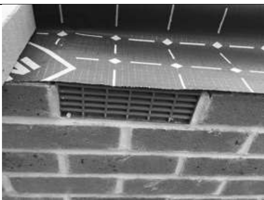
Air brick in place on plot 2.
