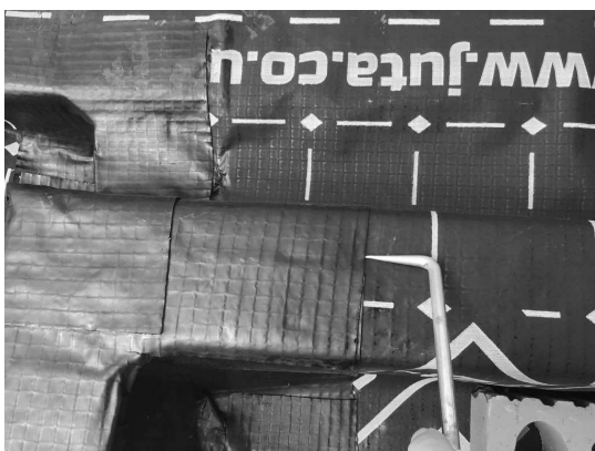
Pick testing all SAGM detailing to plot 7.
