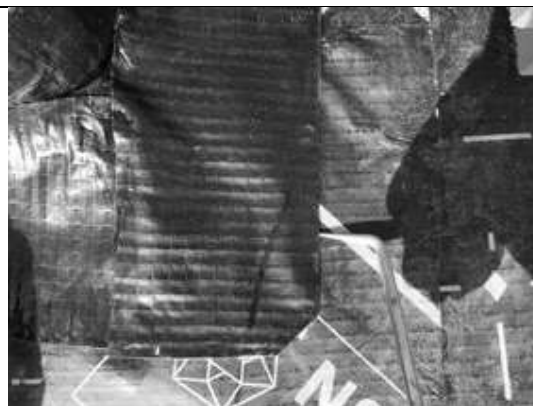
Pick testing all SAGM detailing to plot 5.
