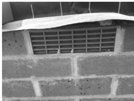
Air brick in place under the membrane at the time of our inspection to plot 9.
