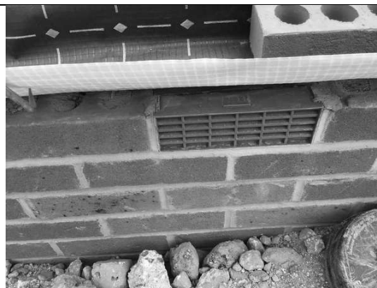
Air brick in place under the membrane to all plots.
