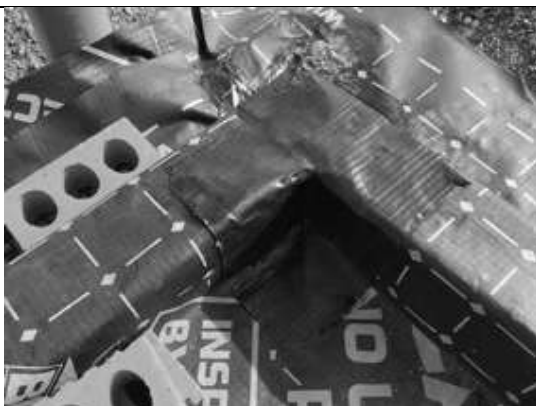
Typical corner seal using SAGM to plot 5.
