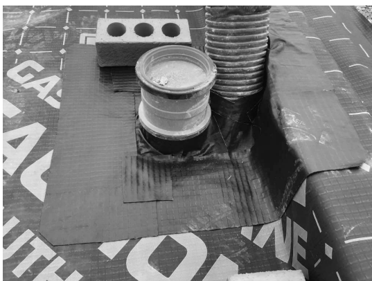
Typical double pipe penetration seal using SAGM to plot 10.
