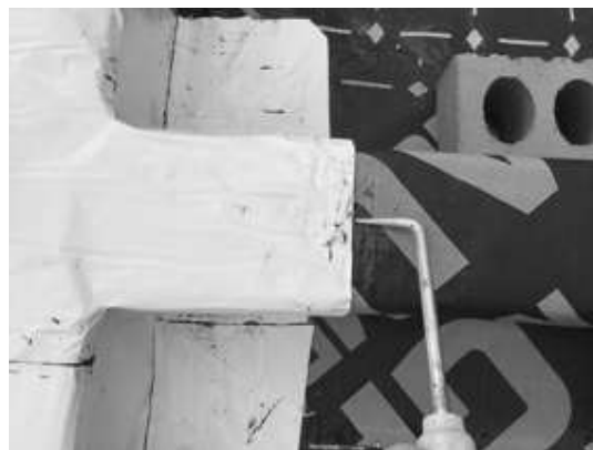
Pick testing all SAGM detailing to plot 3.
