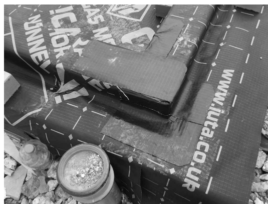
Typical corner seal using SAGM to plot 10.
