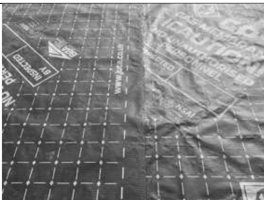
Hand welded membrane lap to plot 6.
