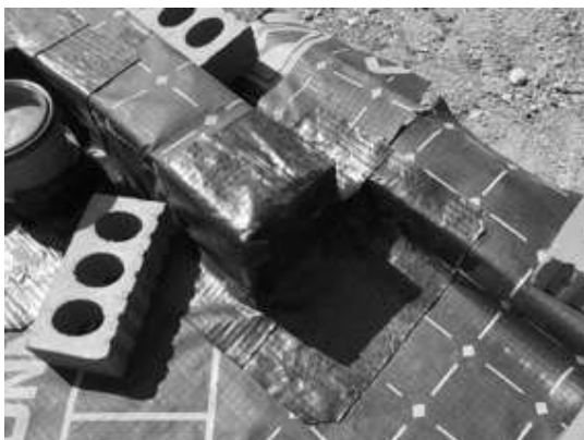
Typical door threshold seal using SAGM to plot 49.
