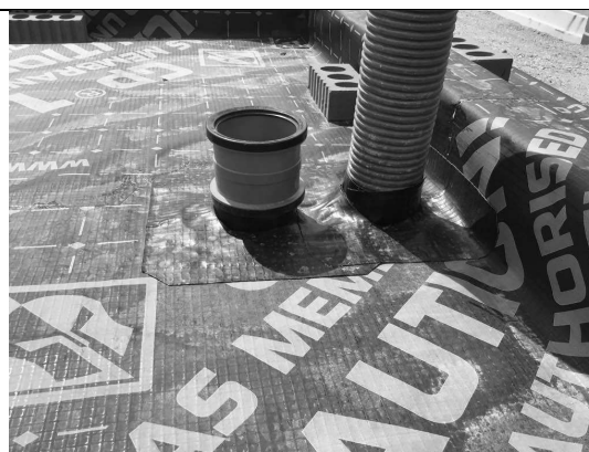
Typical double pipe penetration seal using SAGM to plot 25.
