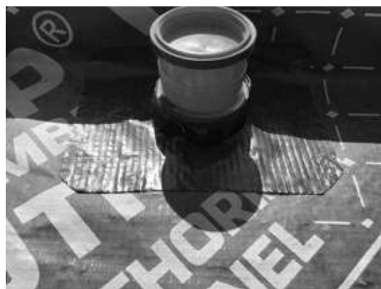
Typical pipe penetration seal using SAGM in plot 49.
