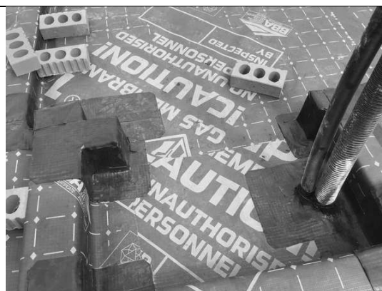
Sealed internal door thresholds using SAGM to plot 42.
