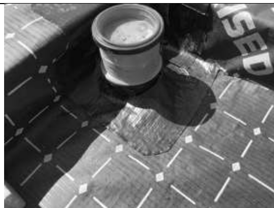
Typical corner seal using SAGM to plot 48.
