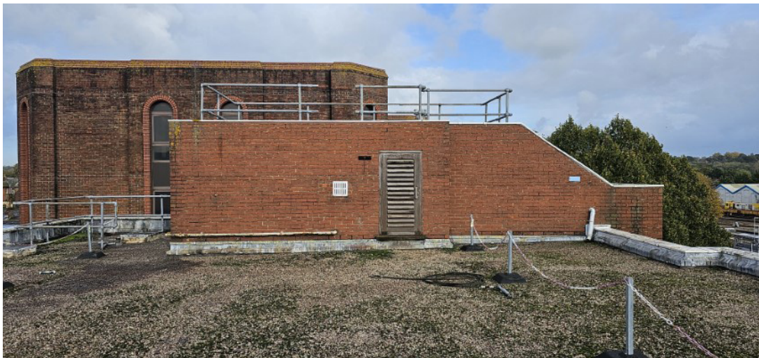
ROOFTOP VIEW OF CAPITAL HOUSE - EXISTING PLANTROOM AND ROOF ACCESS
