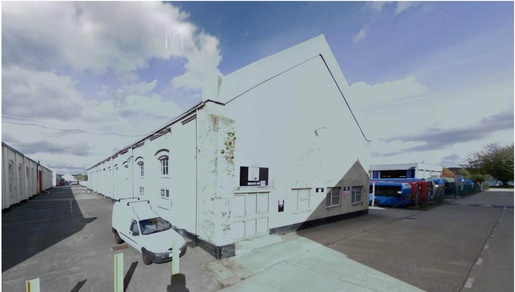
Figure 6 Unit 10 Existing South and West Elevation (Area where the future service yard will be placed)
