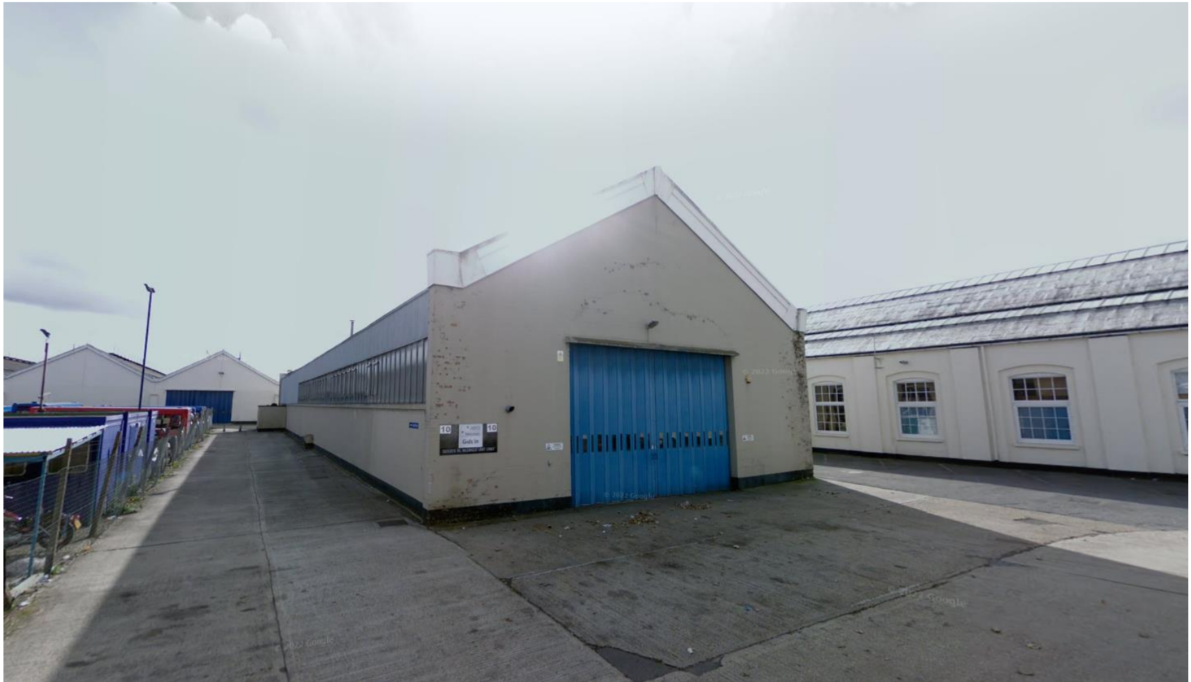
Figure 5 Unit 10 Existing North and East Elevation (Area where the future service yard will be placed)
