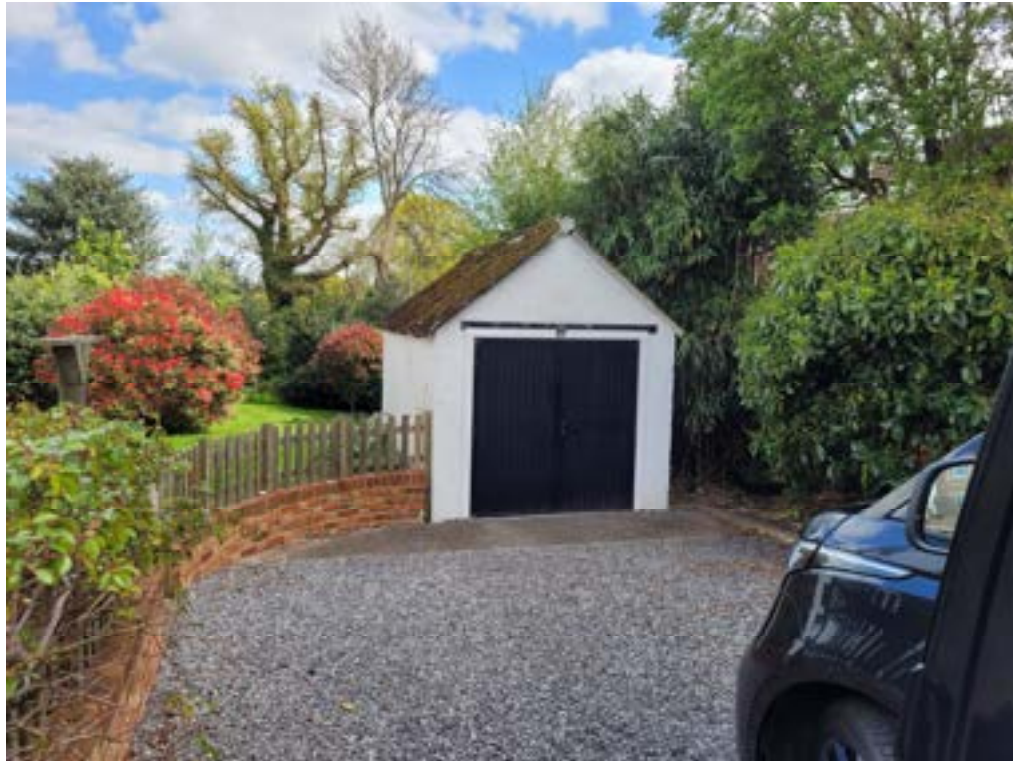
Existing garage to be demolished
