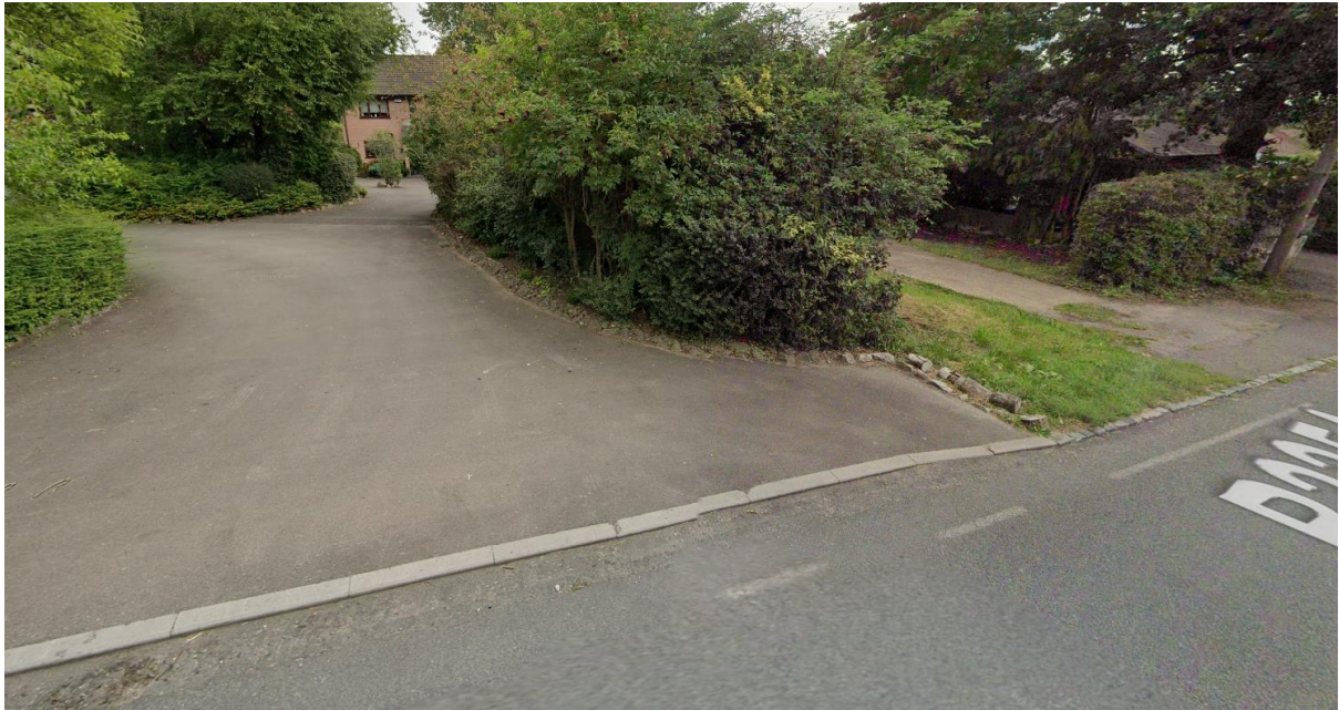
View of recently built shared accesses along Botley Road with no pavement
