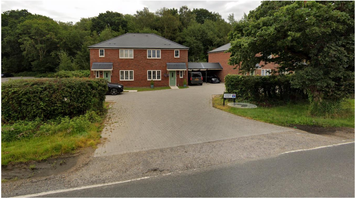
View of existing access to appeal site
