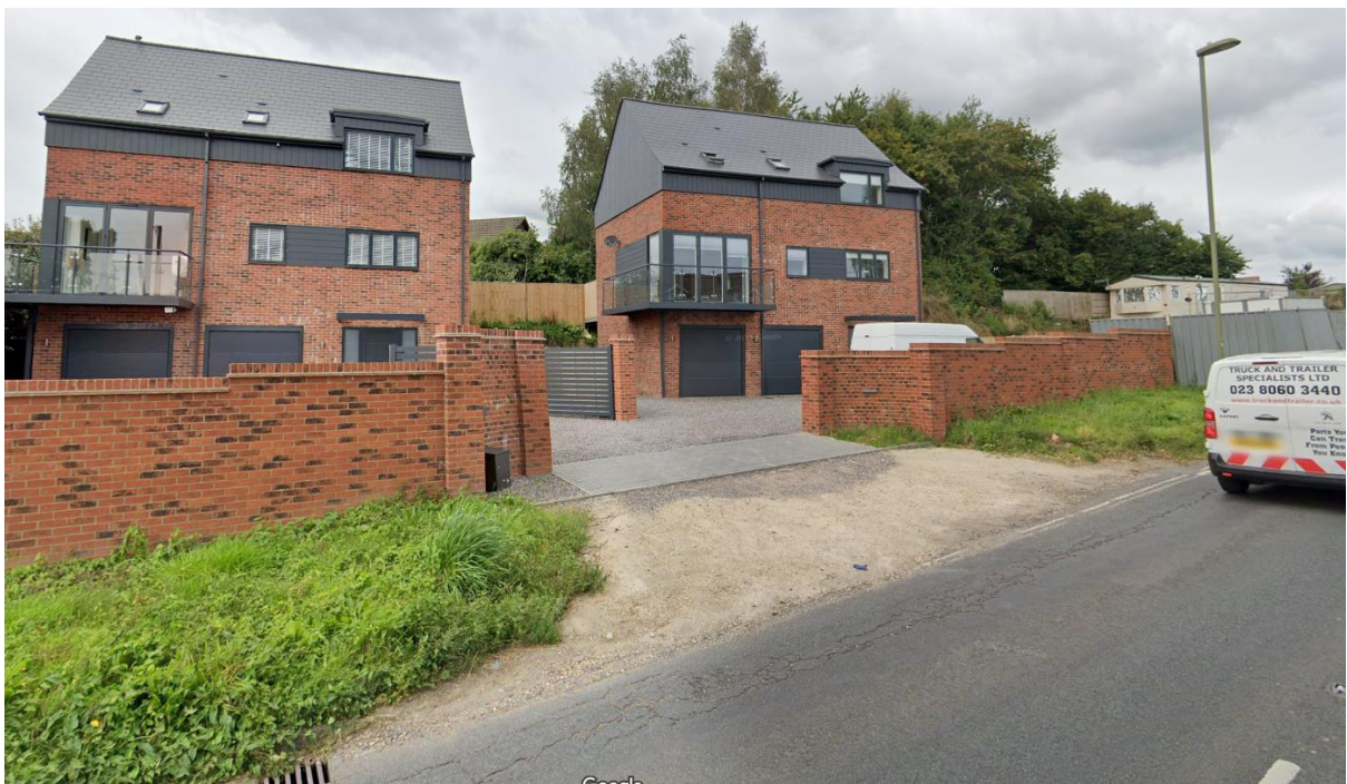
View of recently built shared accesses along Botley Road with no pavement
