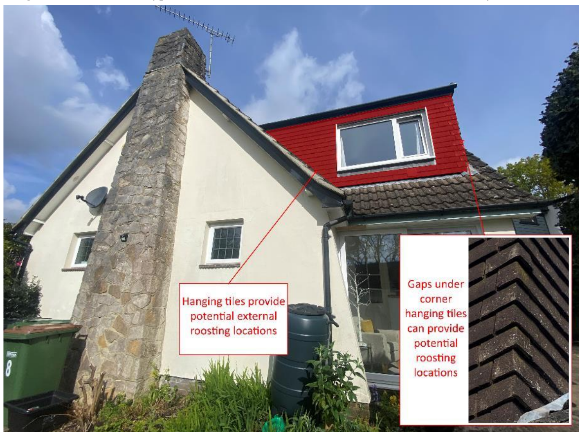
Image 4.3.1.1. Location of potential external roost locations on the east elevation of the house.
