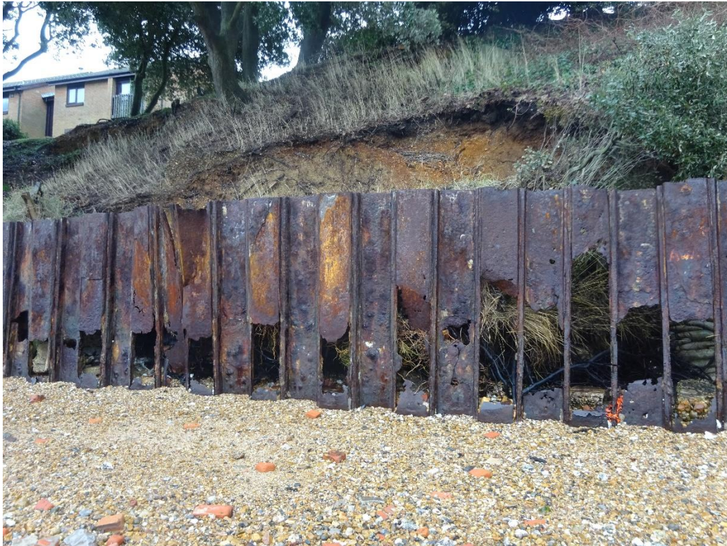
Figure 3 - Photo of the existing sheet pile wall from 2024
