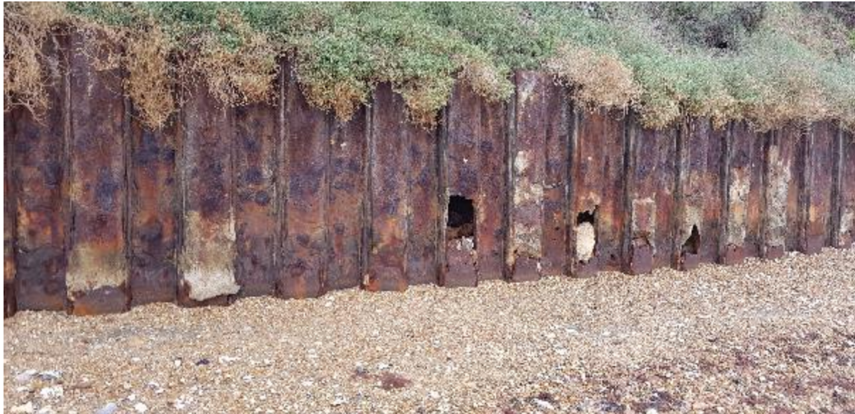
Figure 2 - Photo of the existing sheet pile wall from 2020
