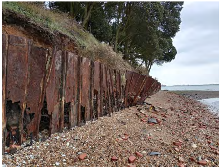
Figure 2: View looking south along the current sheet piling
