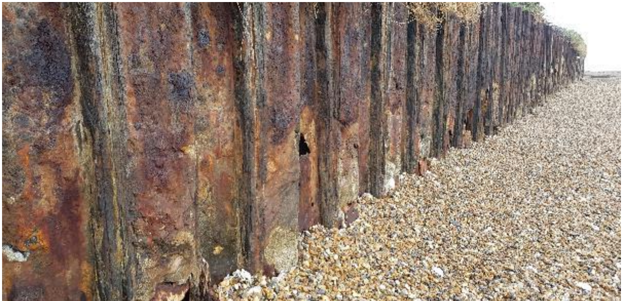
Figure 4-1 Photograph of Existing Sheet Pile Wall
