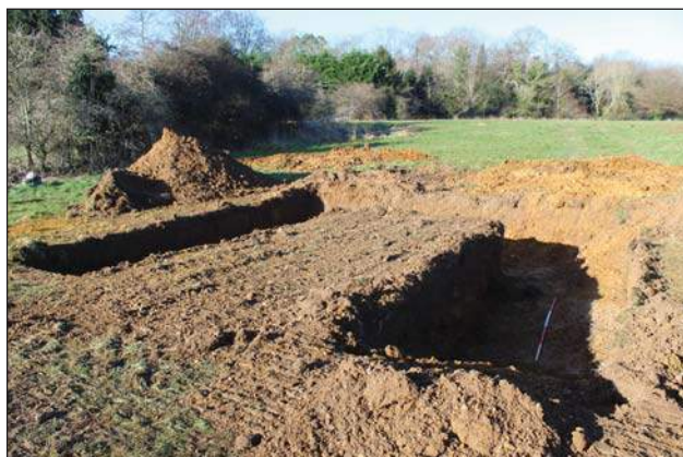
Plate 11, Area strip around backfilled Test Pit 2, looking Northwest. Scale: 2m
