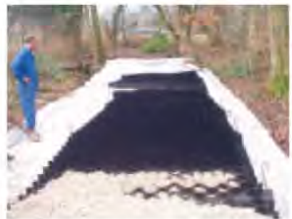
Installation of the CellWeb™ system.
