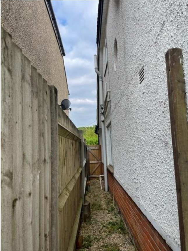
Boundary between 107 and 109 taken from rear of properties. Downstairs bedroom in 107 is rt of frame. N.B. there is only 1.90m between 107 and 109
