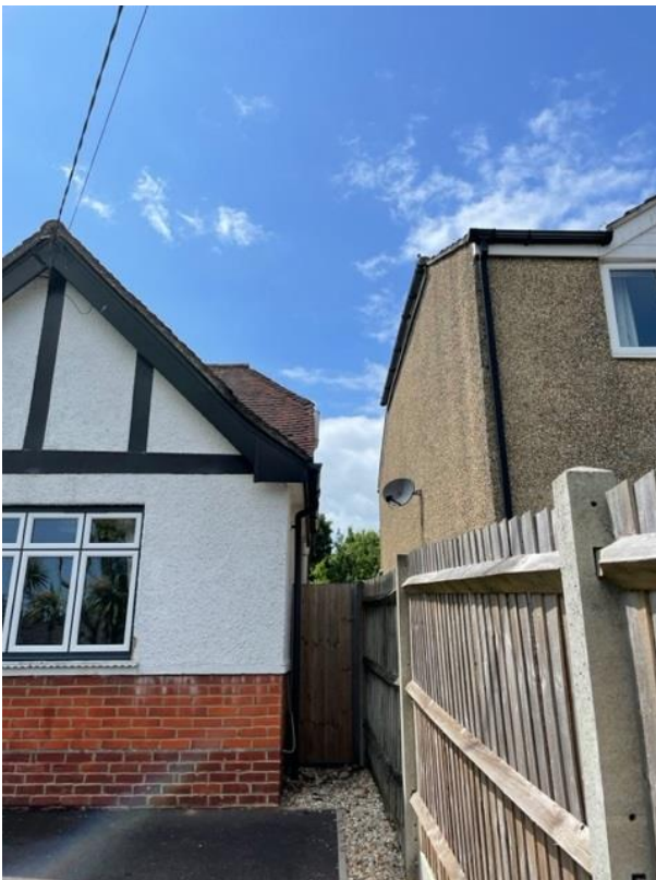
Pic showing current overbearing mass of 109 with Existing cropped gables. It is proposed that height of gable end be raised by 2.87m
