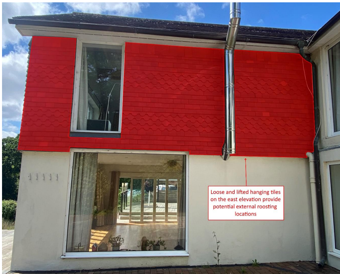
Image 4.3.2. Location of and potential external roost locations on the east elevation of the house.
