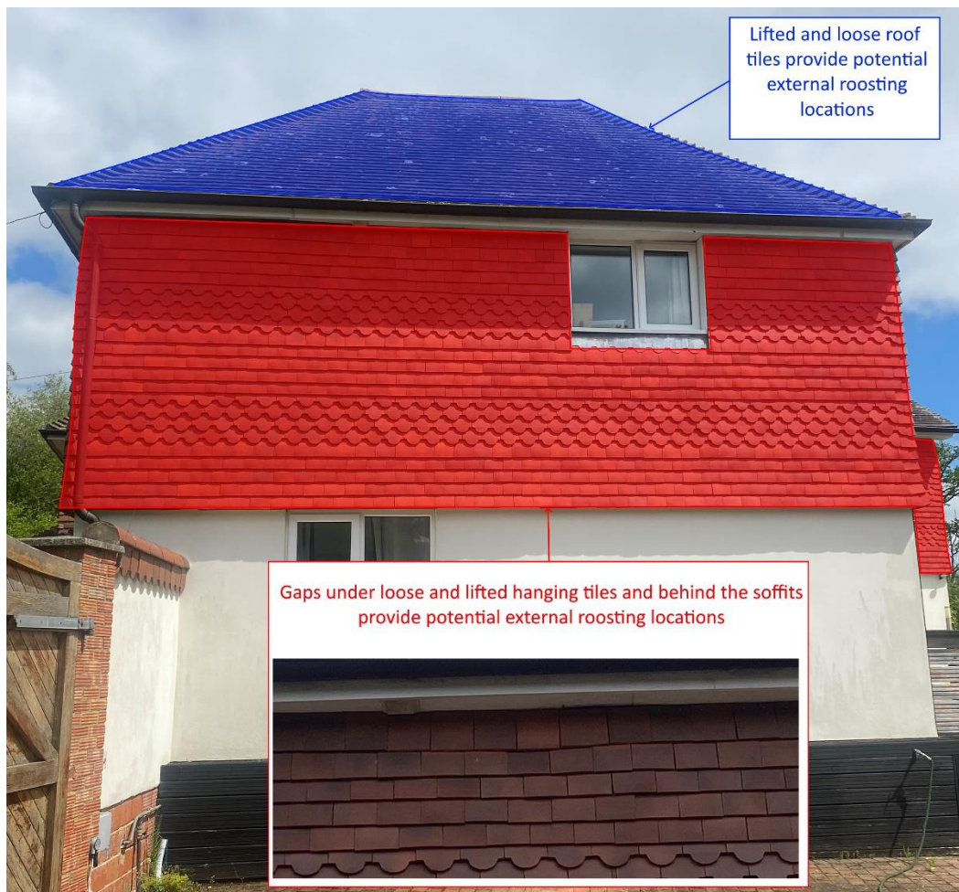
Image 4.3.4. Location of potential external roost locations on the west elevation of the house.
