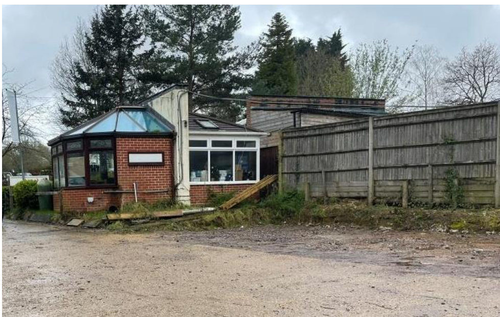
View of existing conservatories to the east looking south from site to the north
