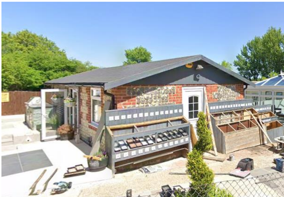
View of existing brick built office building
