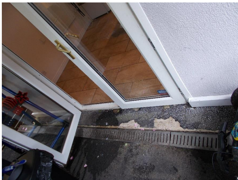
Existing Eco Drain to the north of the kitchen, laundry building.
