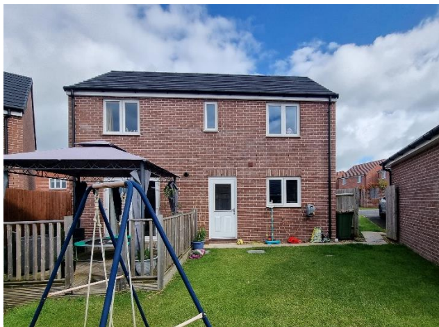
Rear Façade facing South.
