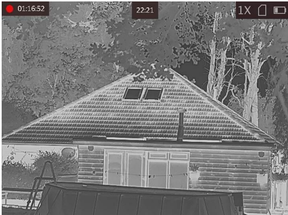
Thermal on Rear of Main dwelling
