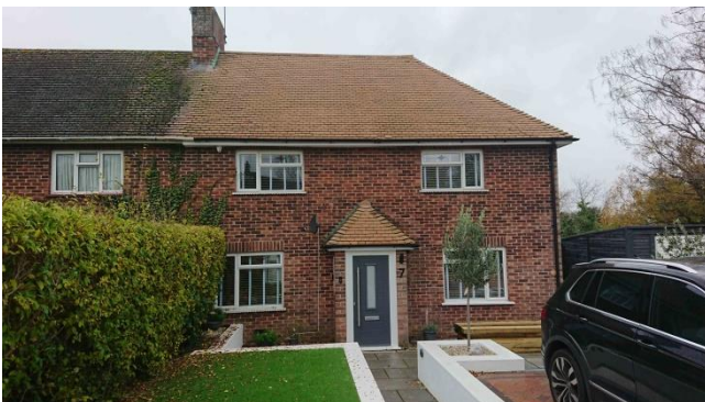
View from Scotland Close of the front (East) elevation and neighbouring house.
