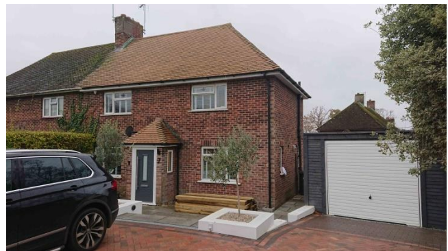
View from Scotland Close of the front (East) elevation and neighbouring house showing the existing garage.
