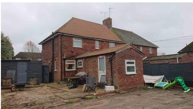
View from the back garden showing the existing extension, party boundary and the neighbouring house.
