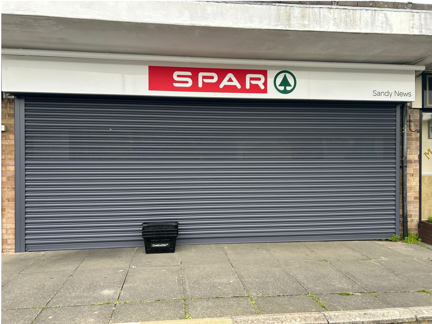
Site Photograph Showing Shutters Closed (NTS)
