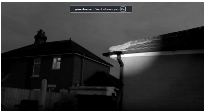
Figure 5. Field of view of 2 nd survey NVA (infra-red camera) on east corner of building. Image taken at darkest point of survey.
