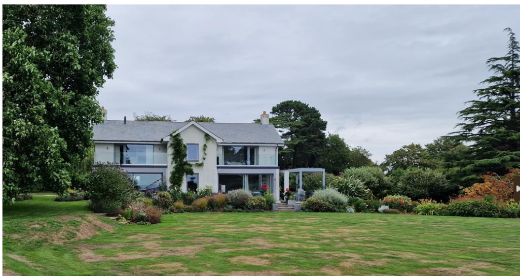
Existing rear elevation of the dwelling
