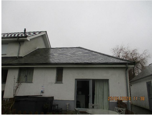
Photo 2: Rear elevation – single-storey extension.
