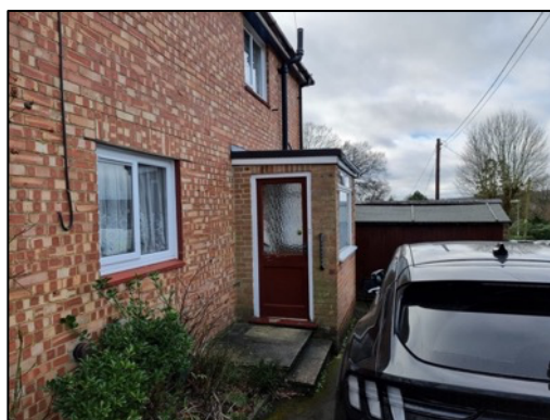
Figure 3 – western elevation with single extension
