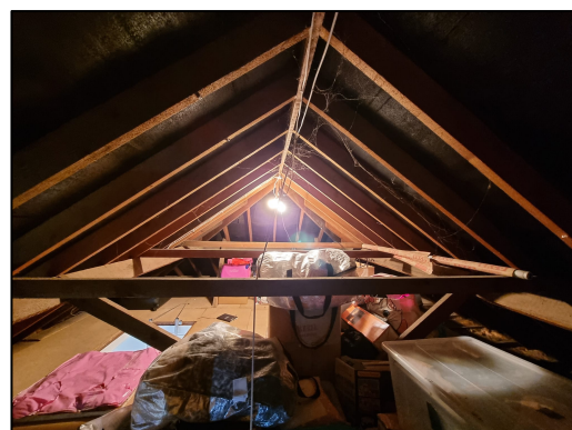
Figure 4 – interior roof void of the house
