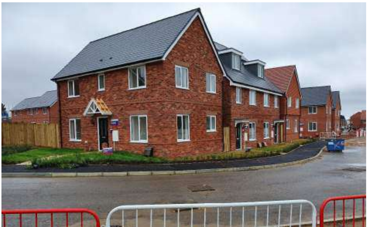
Photograph 6: Nearly completed residential properties in the north west of the site
