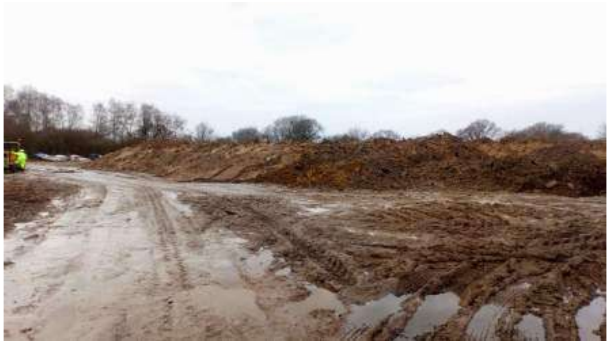
Photograph 5: Burrage Green soil stockpile, facing south.
