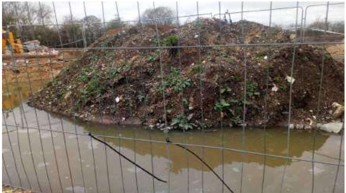
Photograph 6: asbestos impacted soils remain on site following completion of knotweed remediation
