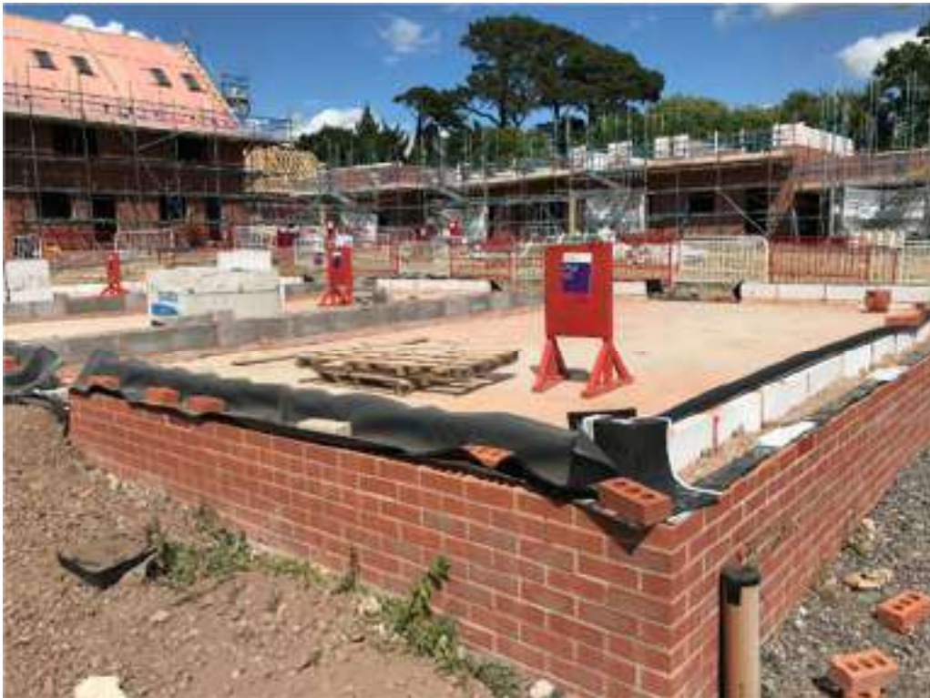
Photograph 6: Re-inspection of gas membranes P61 – P62
