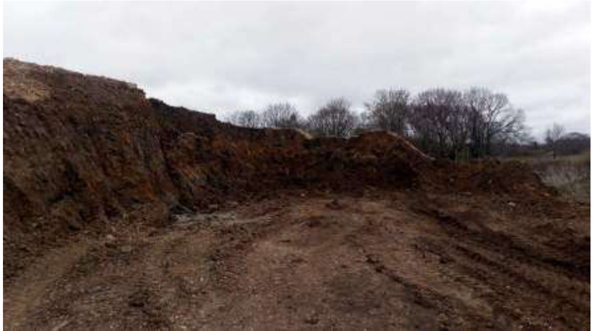
Photograph 3: Topsoil stockpile being reused for capping
