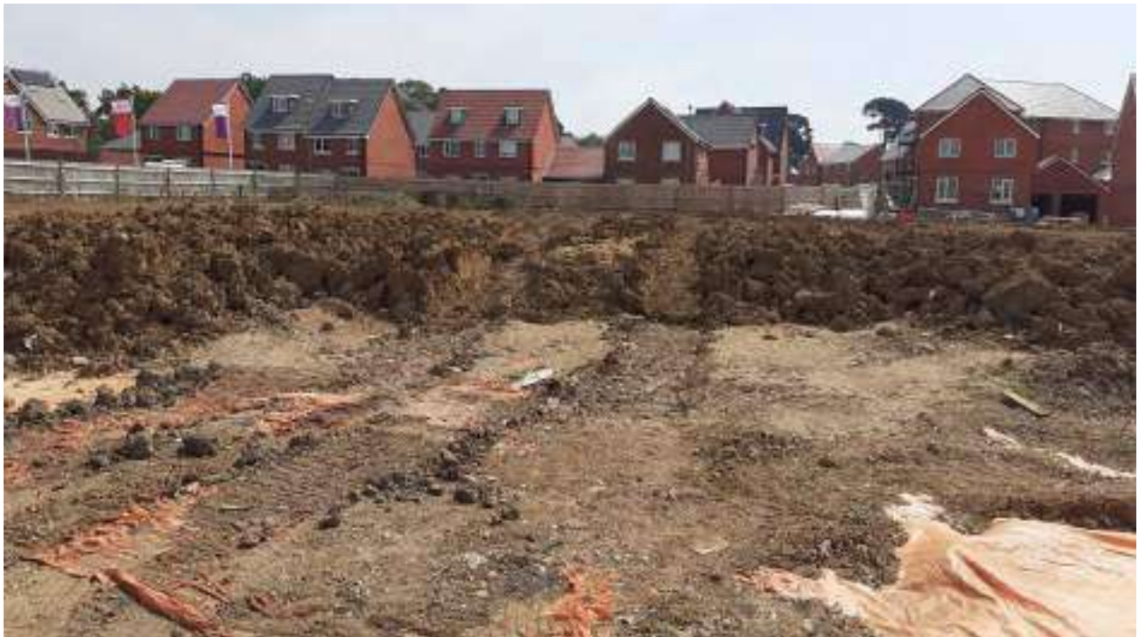
Photograph 2: Recently placed soils to the north of site compound
