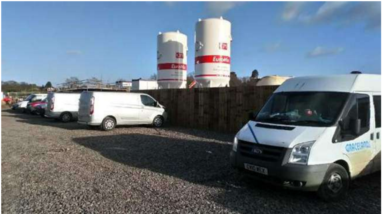
Photograph 6: View of Taylor Wimpey compound, parking in foreground and batching plant present.
