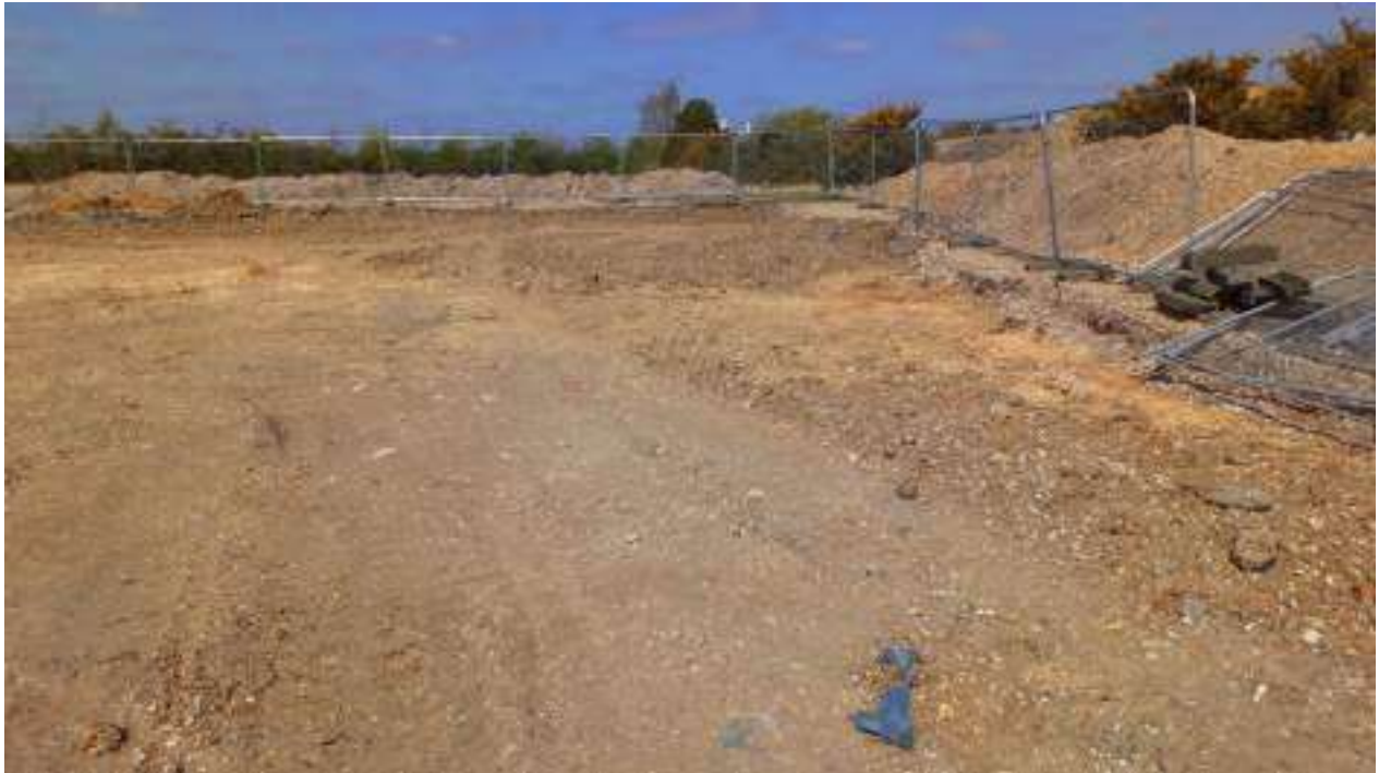
Photograph 5: View looking west across Japanese Knotweed burial cell.
