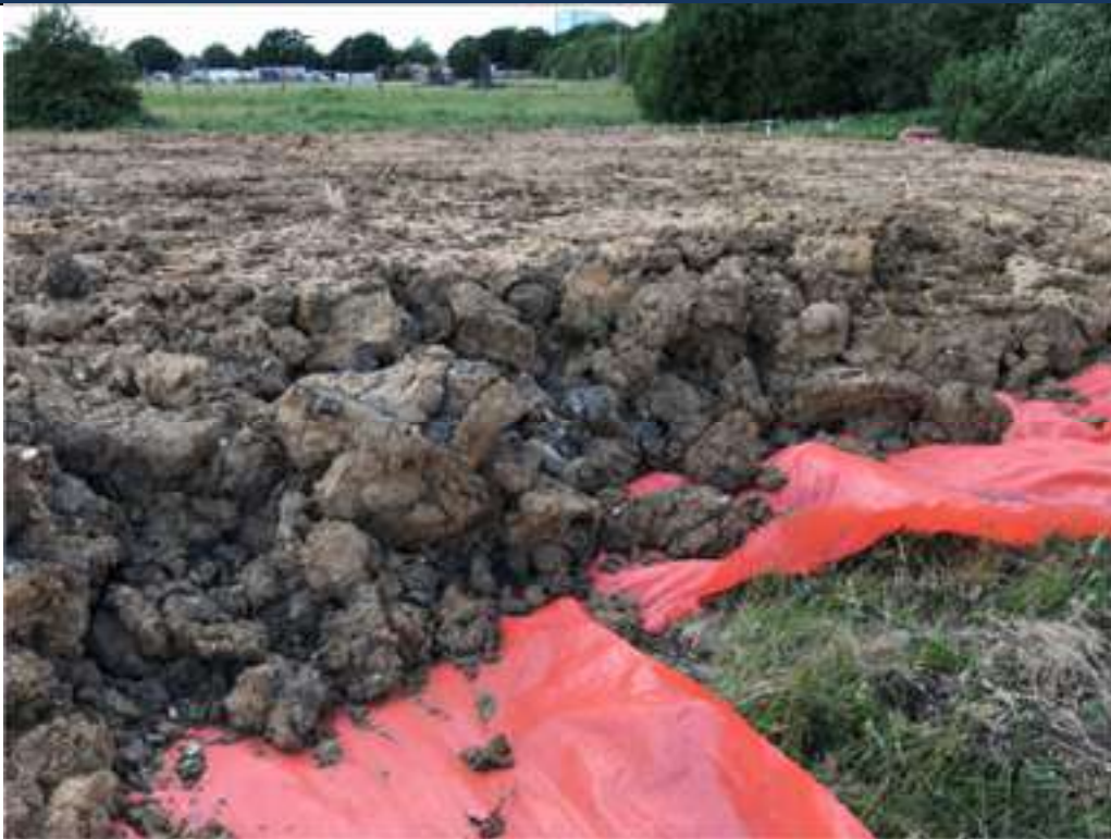
Photograph 1: Cover system in former landfill area
