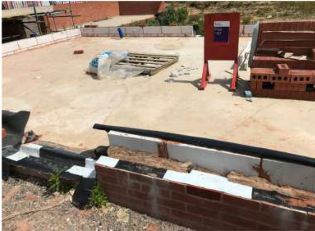
Photograph 3: Re-inspection of gas membranes P182
