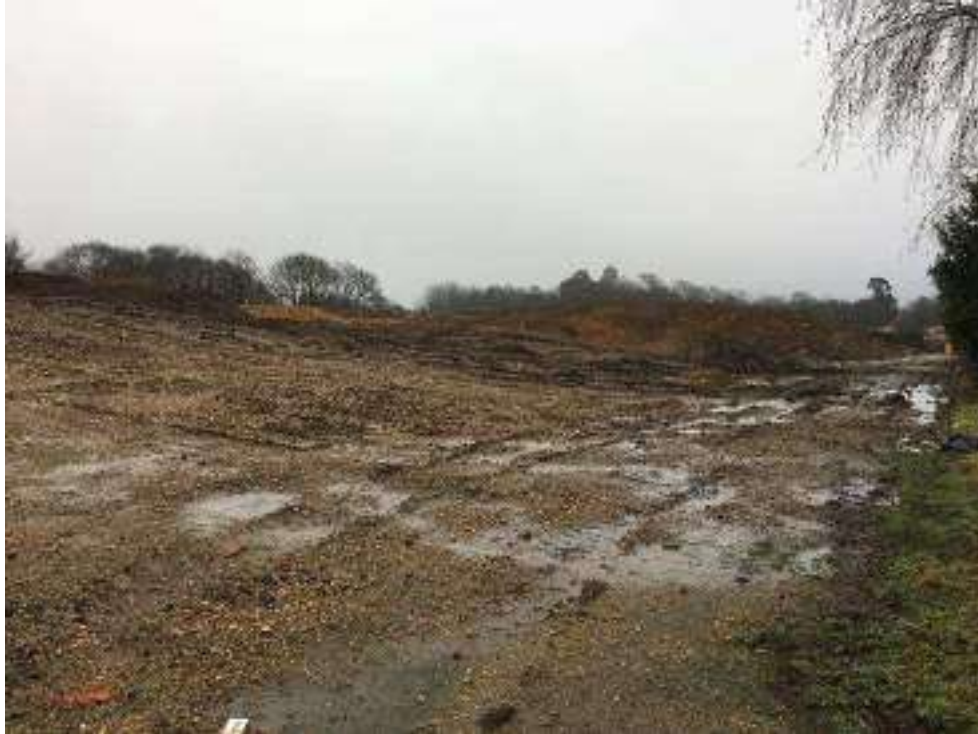
Photograph 3: view looking north across stockpile area (left)
