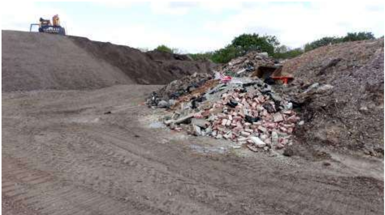
Photograph 4: Construction waste materials placed to the south of the topsoil stockpile
