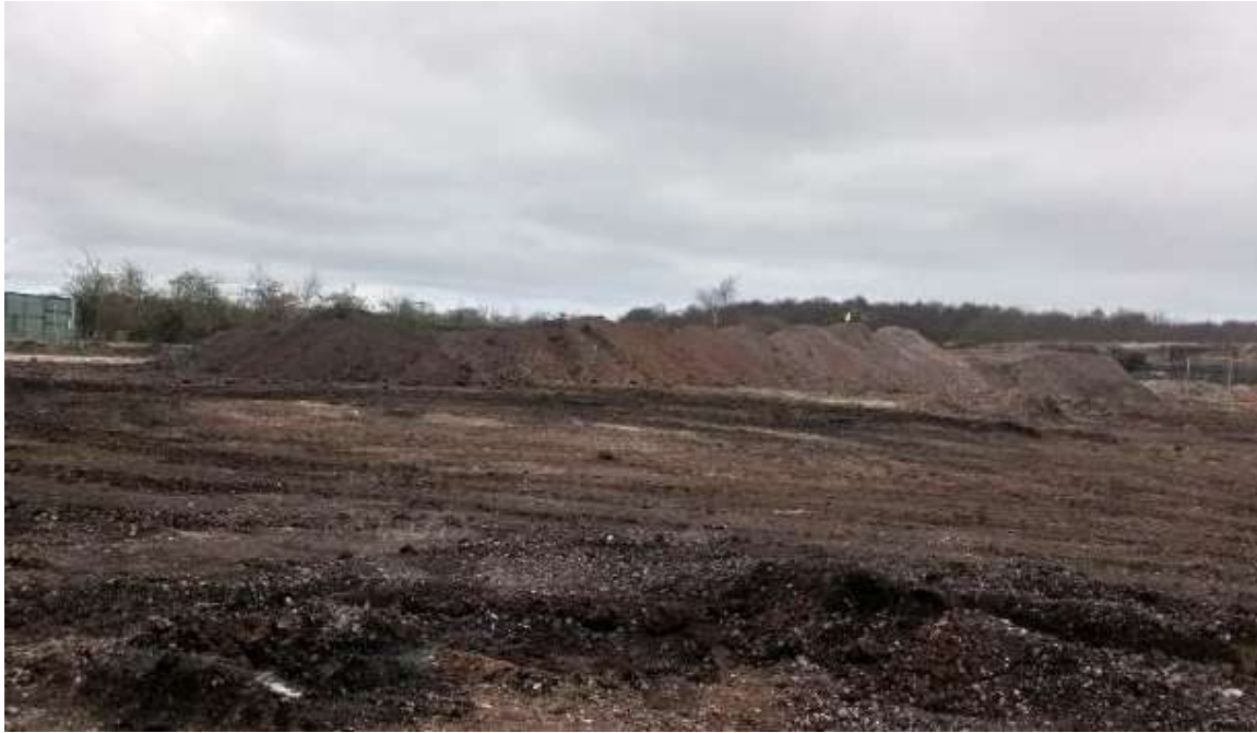
Photograph 1: New stockpiles behind TW compound looking northwest
