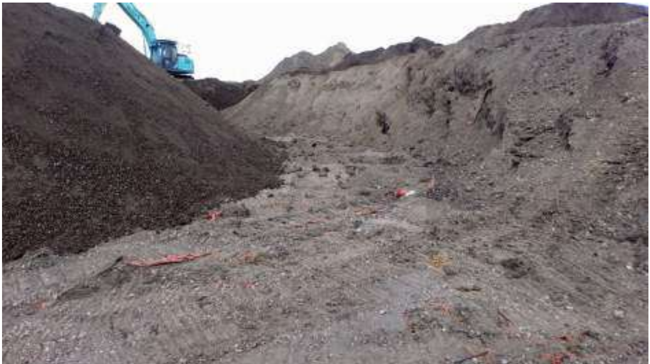
Photograph 2: Membrane evident beneath stockpile and screened Topsoil
