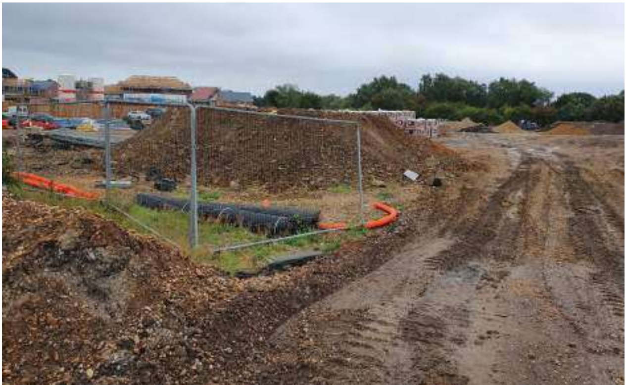
Photograph 2: Soil and brick waste stockpile to west of TW compound
