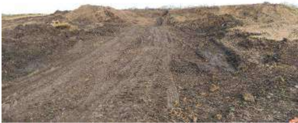
Photograph 1: View looking north towards topsoil stockpile
