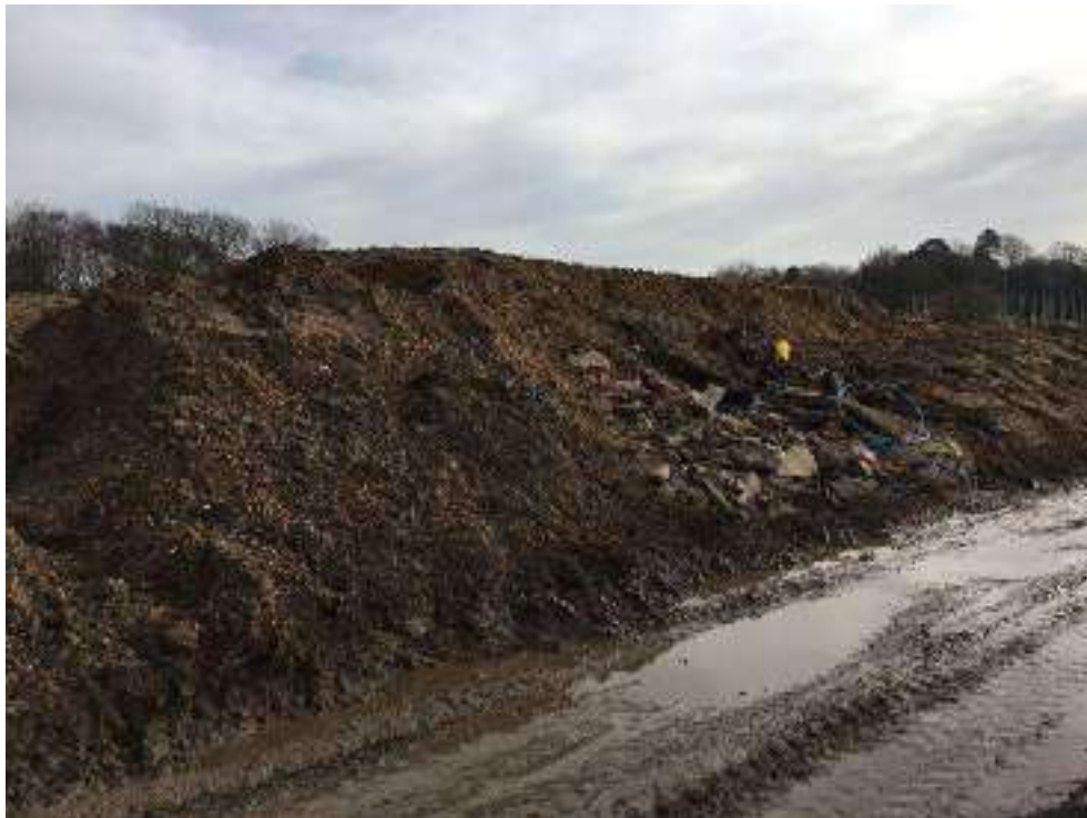
Photograph 4: anthropogenic waste materials placed on mixed stockpile
