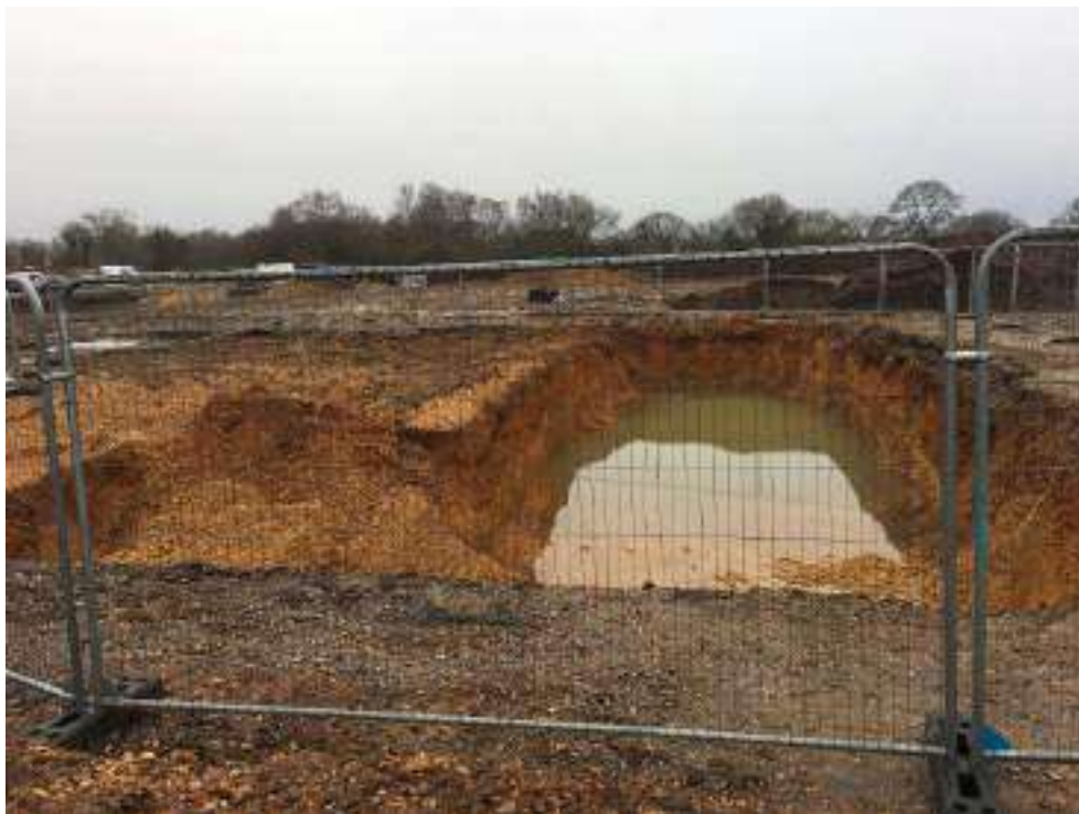
Photograph 6: new borrow pit excavation
