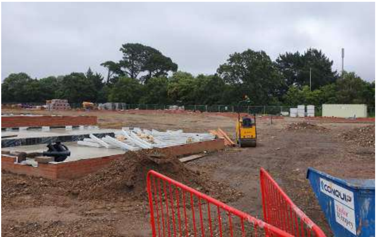
Photograph 8: Preparation of eastern parts of the site for construction
