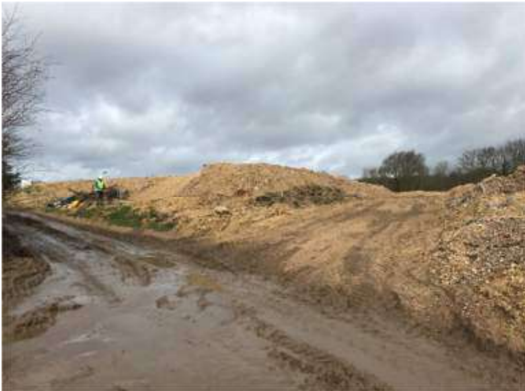
Photograph 4: SP-MM01: Mixed materials stockpile.
