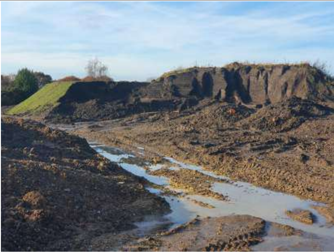
Photograph 3: Remainder of topsoil stockpile. Facing southwest.
