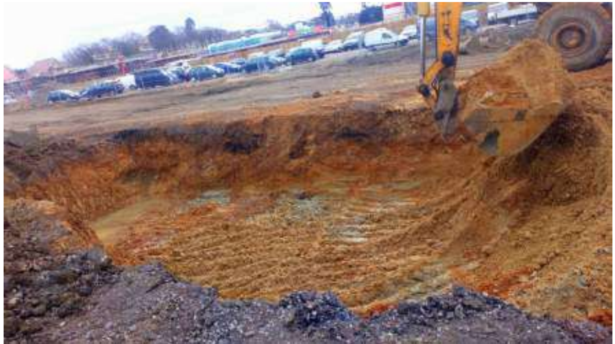
Photograph 5: "borrow pit" excavation
