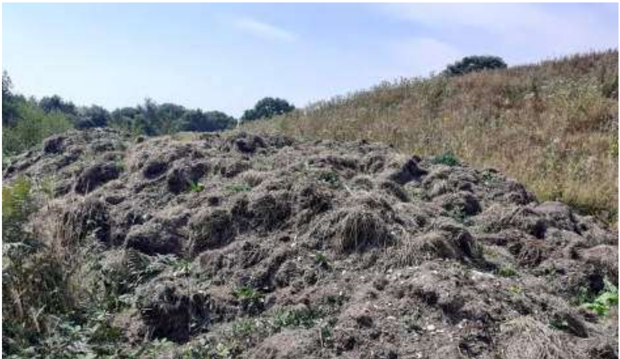
Photograph 5: Recently placed organic soils to east of bund in the south of the country park area.
