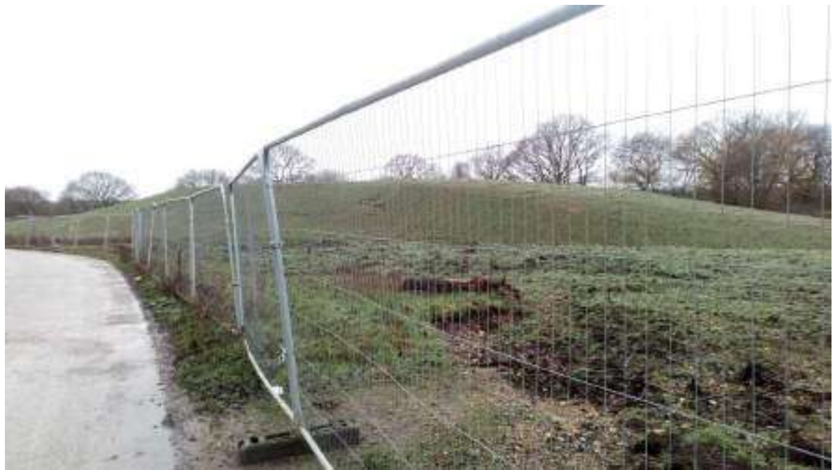
Photograph 6: Overview of the bund to the west of the haul road, looking south. (No access possible).
