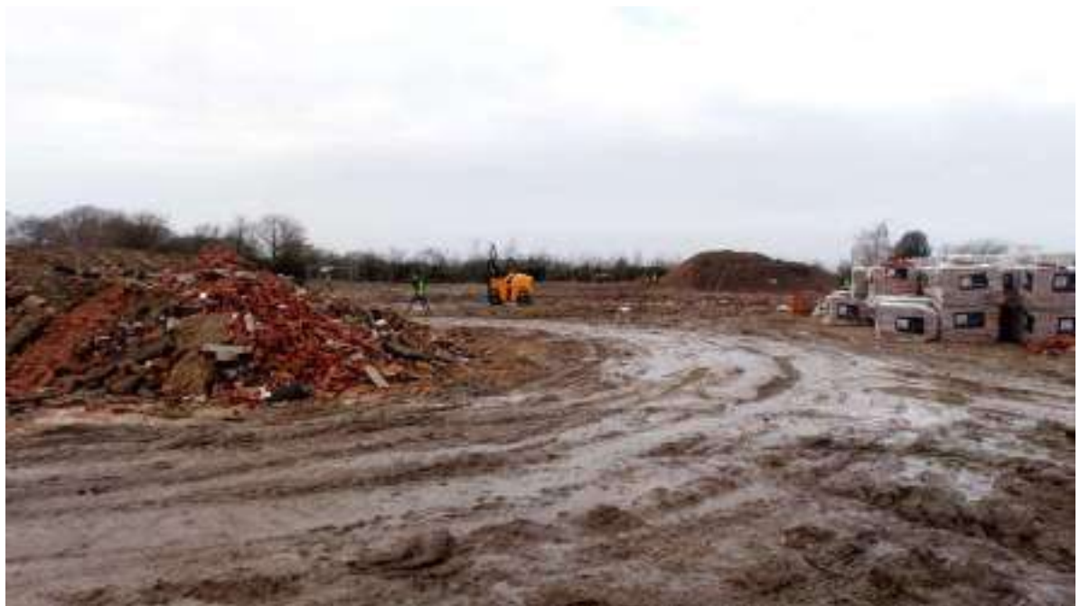
Photograph 4: Area of materials storage (right) and construction waste (left), facing west.
