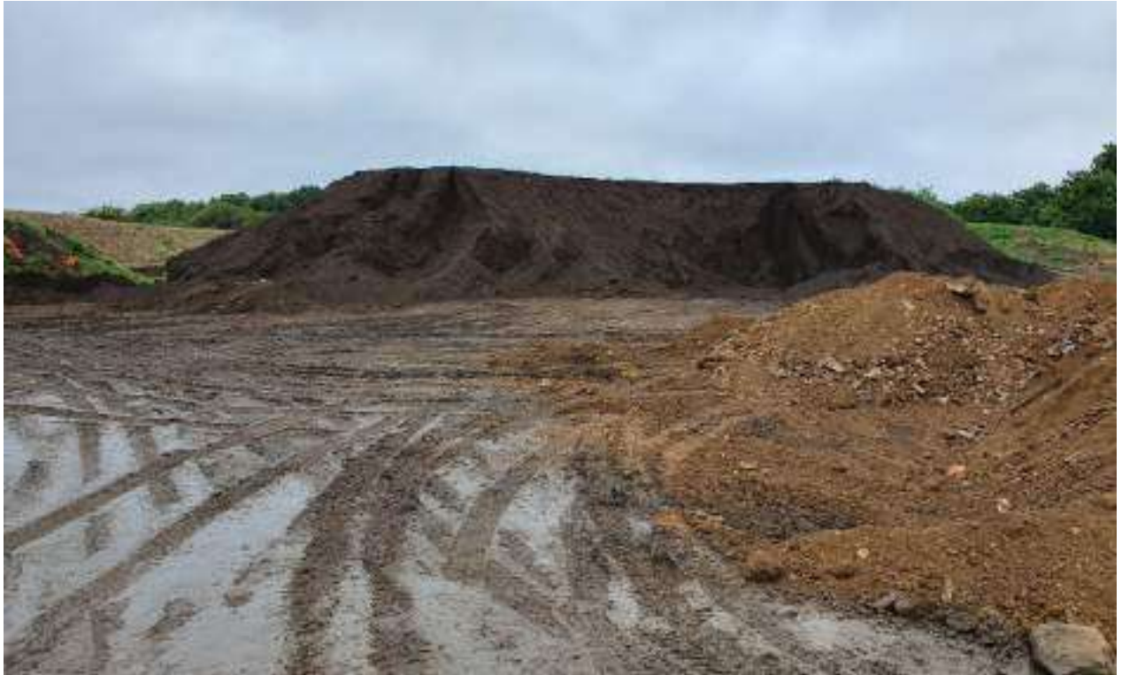
Photograph 3: Screened Topsoil stockpile in north west of site
