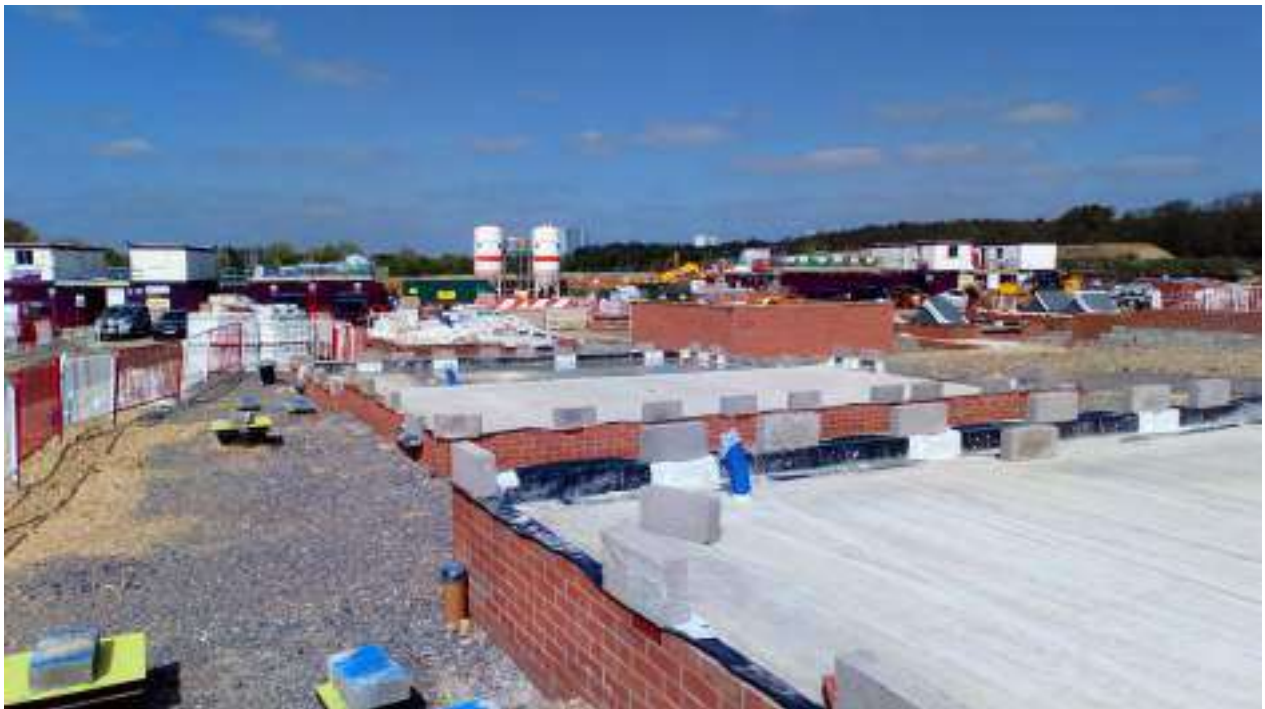
Photograph 2: View across site towards TW compound. Services are clearly identified
