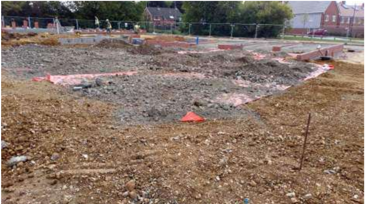
Photograph 8: Placement of crush material on top of membrane in the south east of the site
