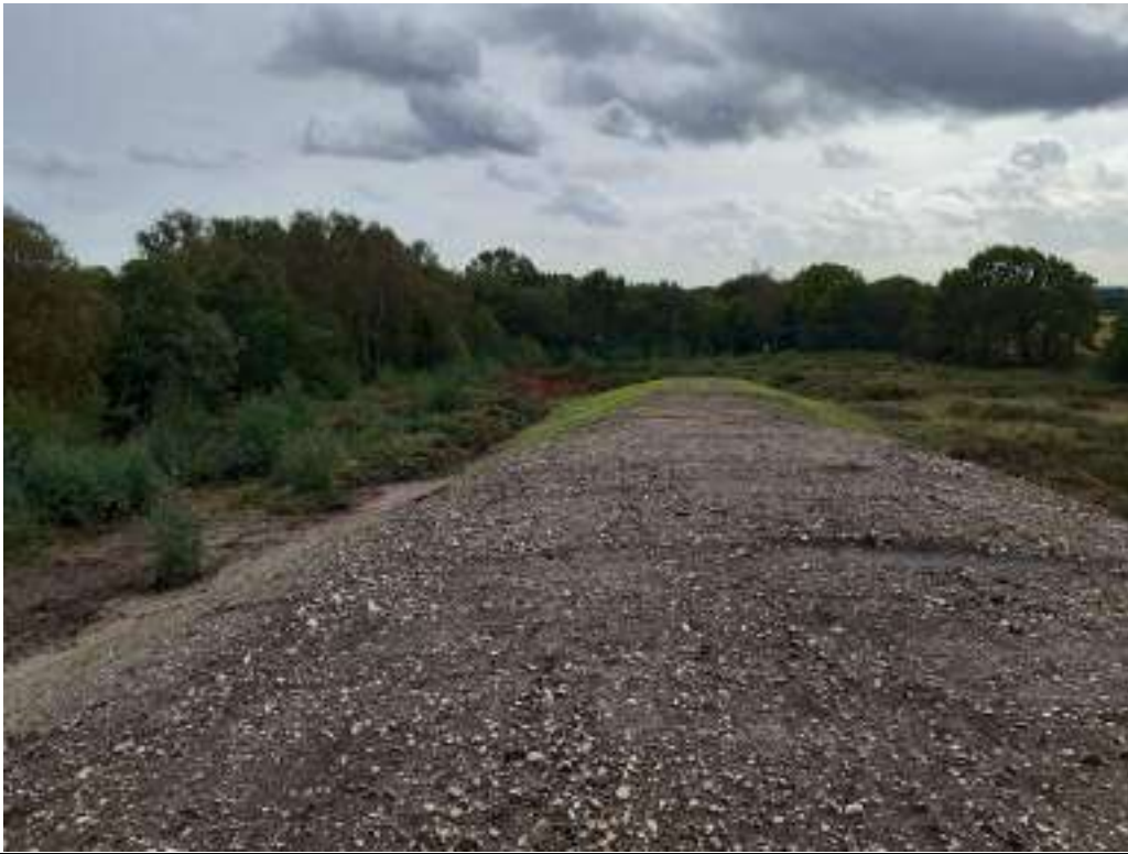
Photograph 1: Looking across the top of the bund, facing southeast.
