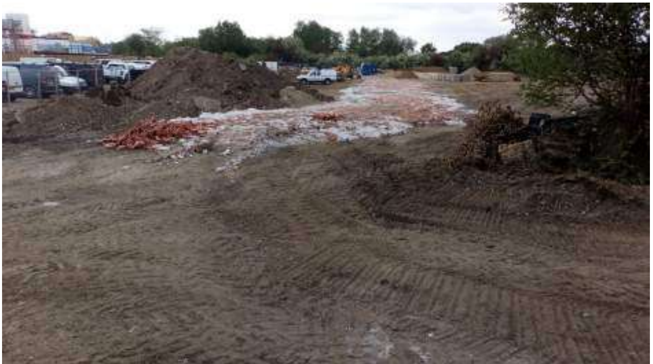
Photograph 6: Looking south toward the constructed access track
