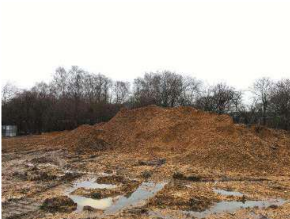
Photograph 4: surplus arisings from knotweed burial cell excavation
