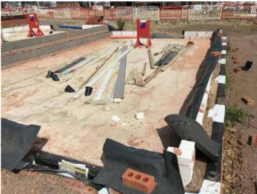
Photograph 2: Re-inspection of gas membranes P63 – P64
