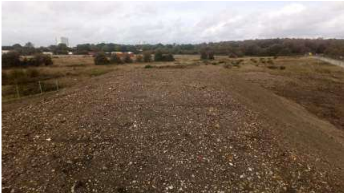
Photograph 2: Looking across the top of the bund, facing northwest.
