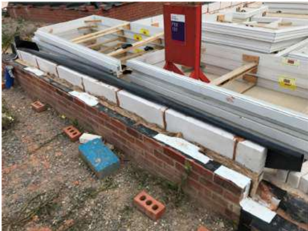
Photograph 4: Re-inspection of gas membranes P181
