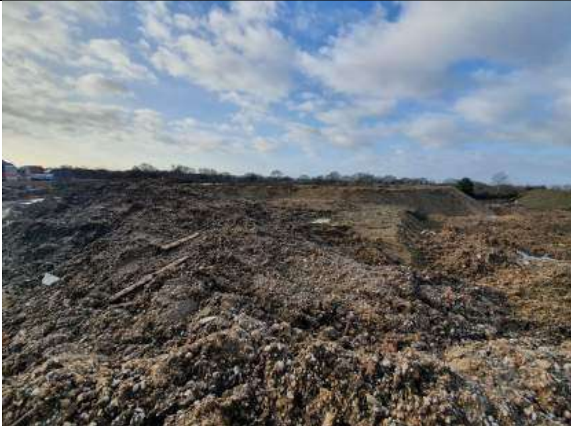
Photograph 4: Remaining mixed subsoil stockpile.
