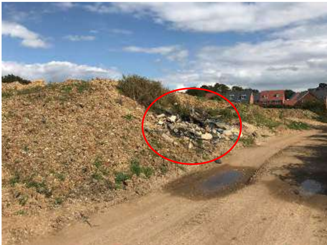
Photograph 4: Mixed soils stockpile – unsuitable materials circled
