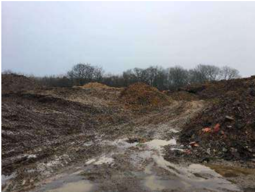
Photograph 2: Stockpile area showing no clear segregation between topsoil (left), sand/gravel arisings (centre) or "muckaway" (right).
