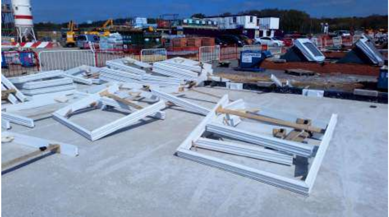
Photograph 3: Materials stored on plots where screed has been placed near site compound.
