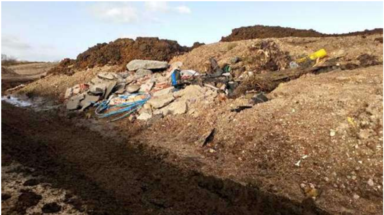
Photograph 8: Various materials within large stockpile area
