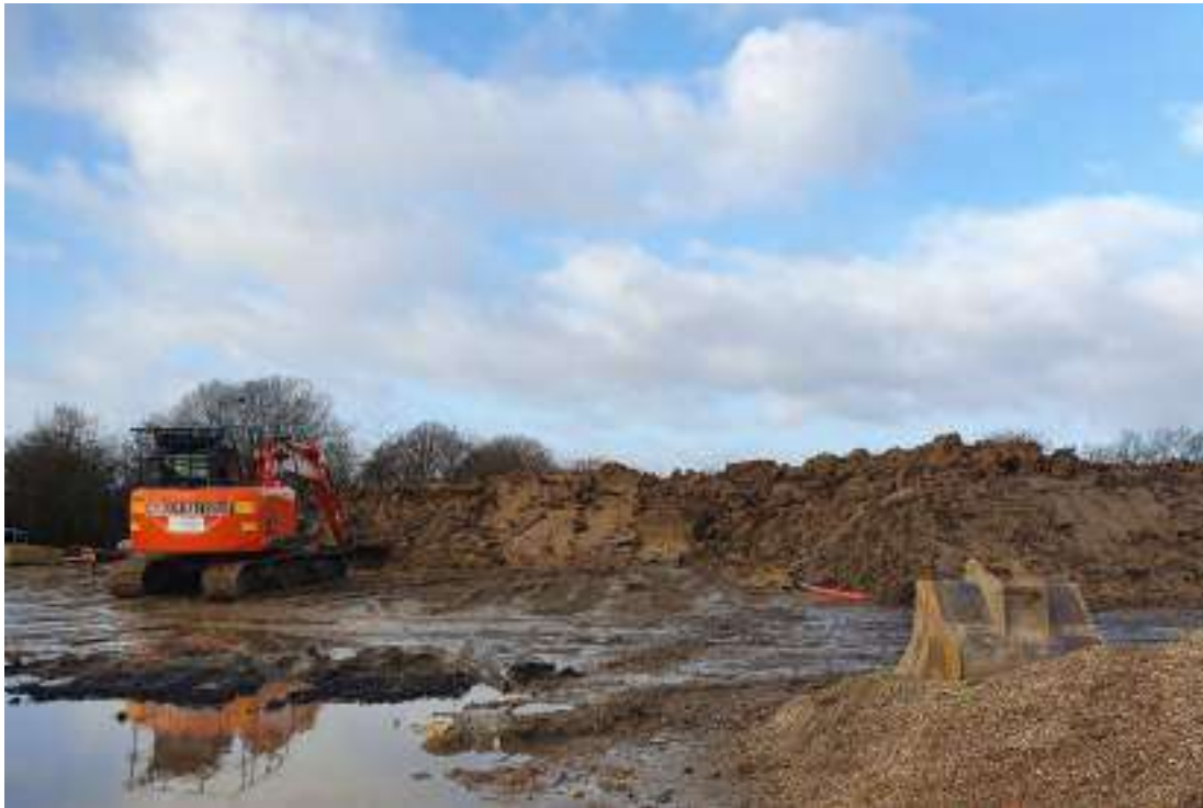
Photograph 1: Looking west towards ongoing stockpiling of soil from Burr ridge Green.
