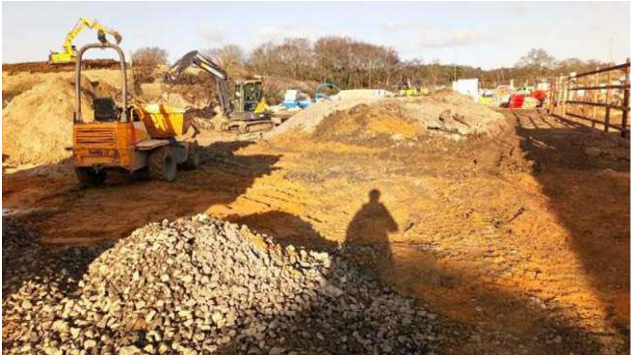
Photograph 7: Stockpiling materials and completion of Taylor Wimpey compound area
