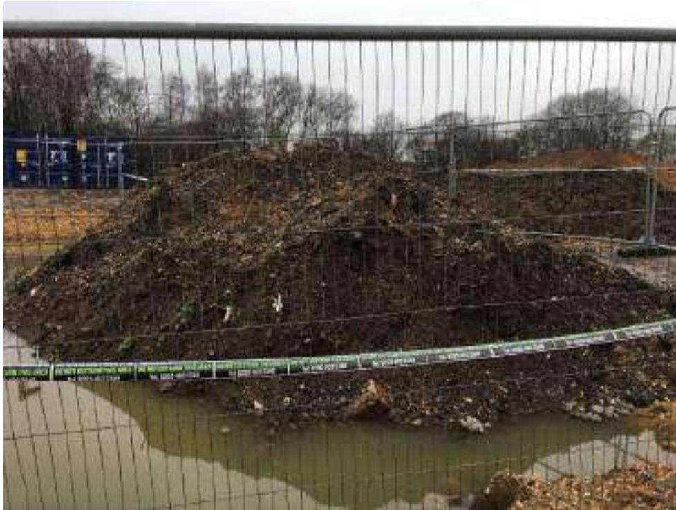
Photograph 7: asbestos impacted soils awaiting disposal off-site
