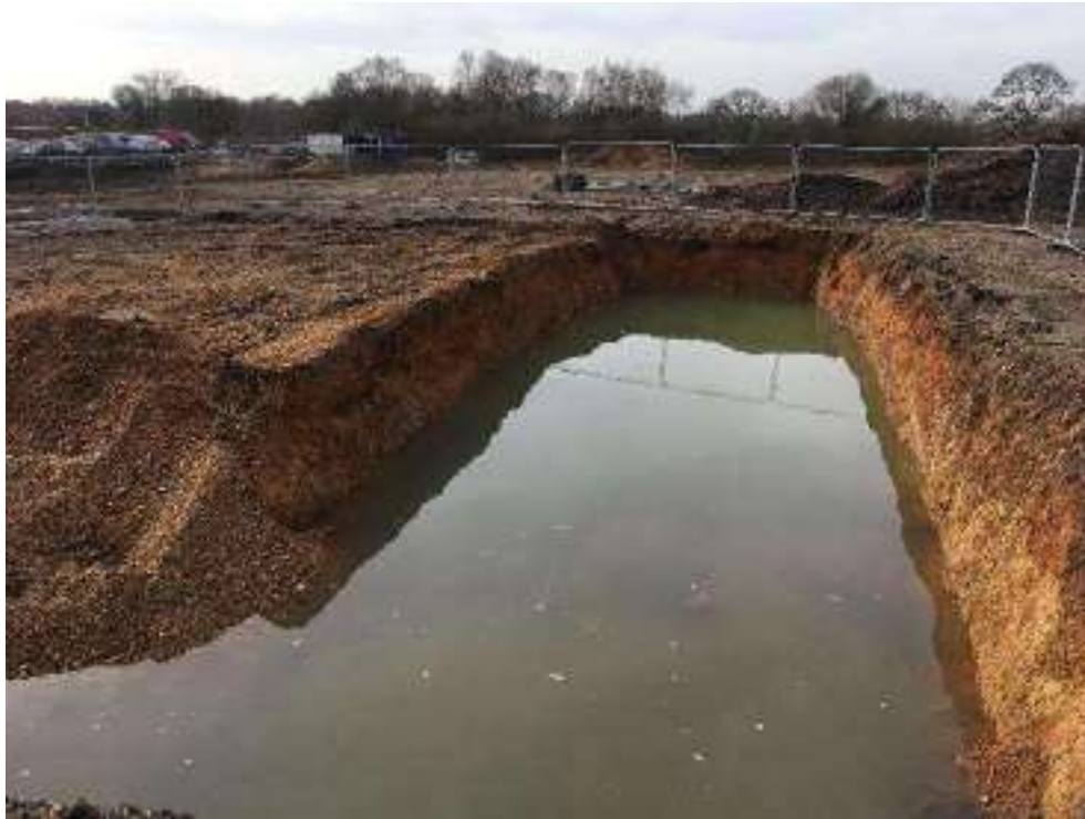
Photograph 5: “borrow pit” excavation
