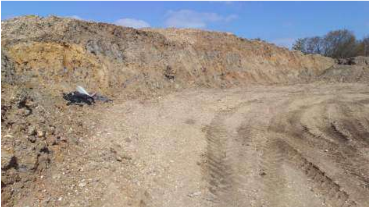
Photograph 7: Stockpiled materials being used. Stockpile at eastern end of stockpile area in north west of the site
