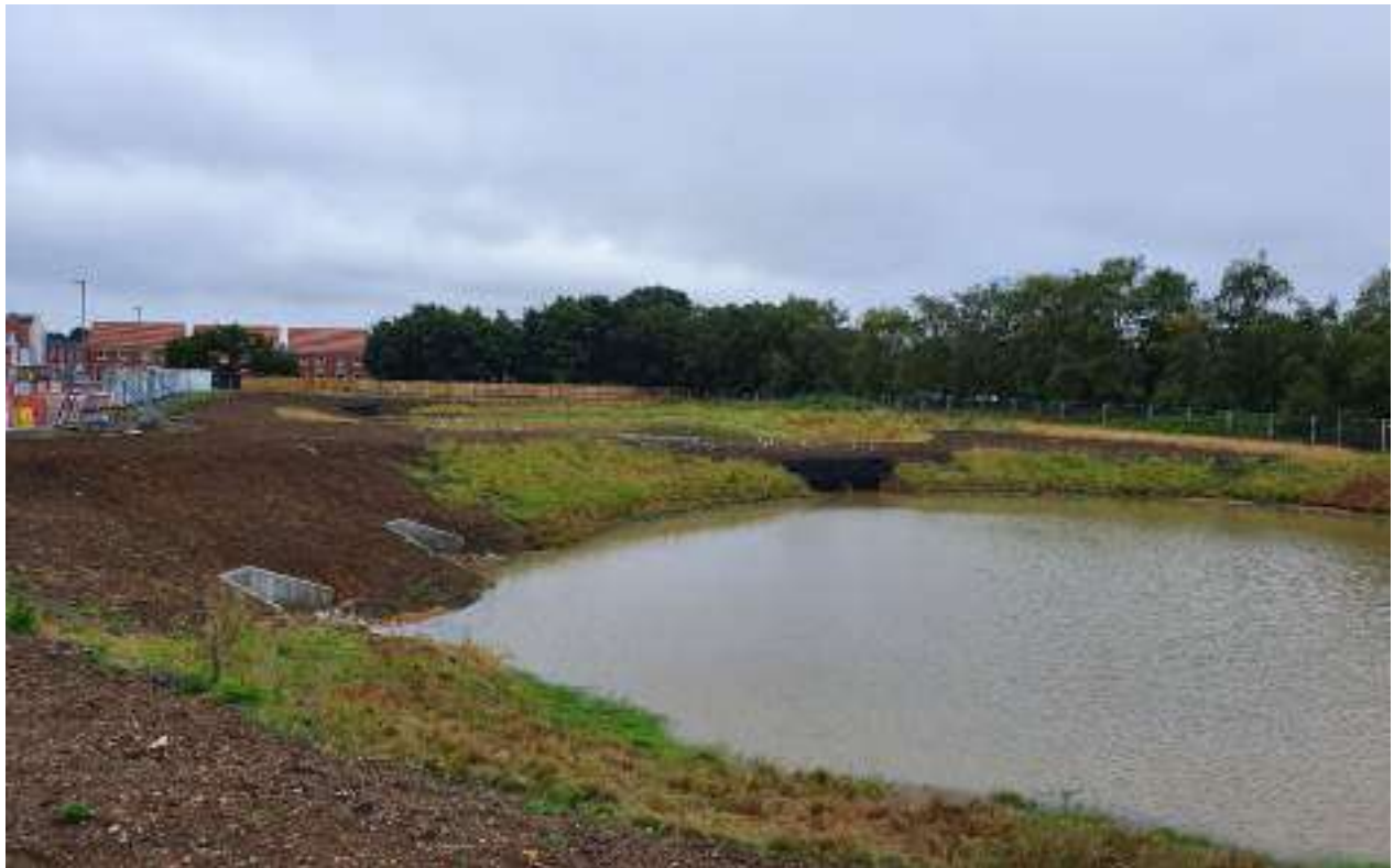
Photograph 5: View of northern most attenuation basin now complete with headworks and Topsoils
