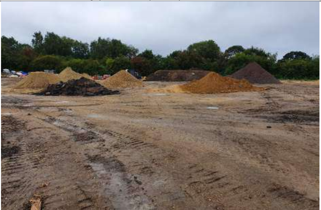
Photograph 4: Various small stockpiles of aggregates to west of TW compound
