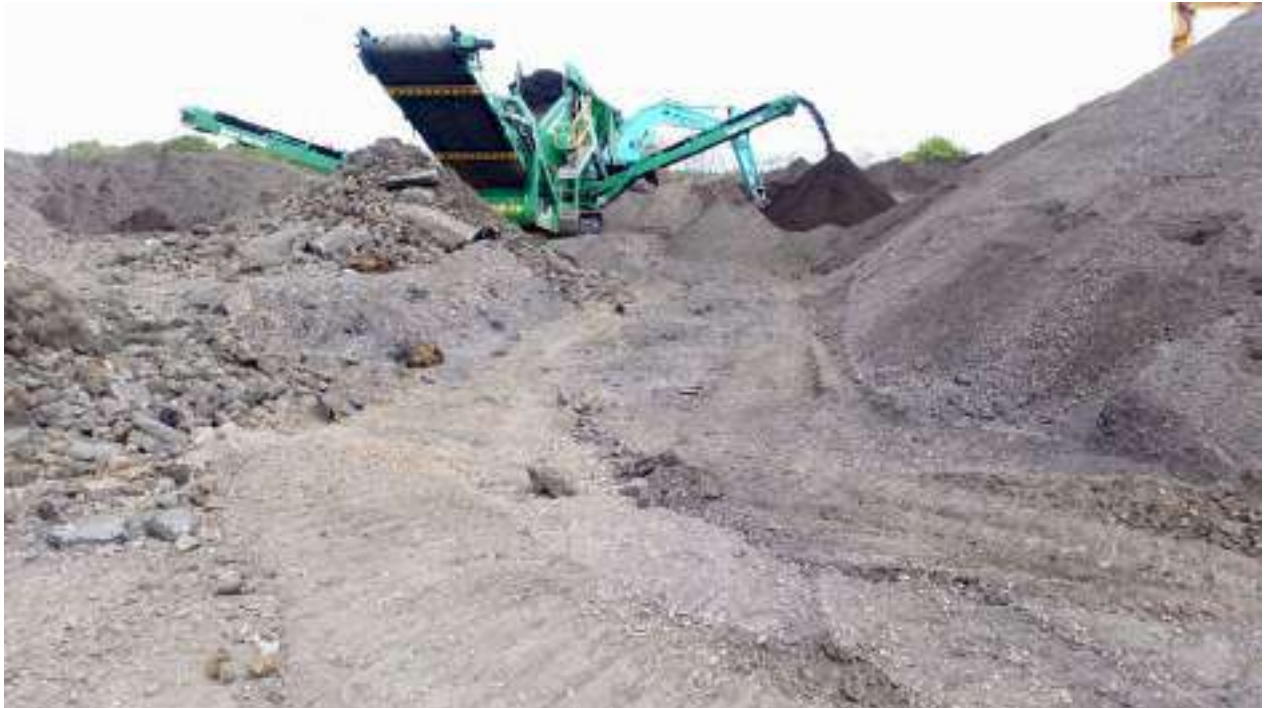
Photograph 1: Ongoing screening of Topsoil stockpiles
