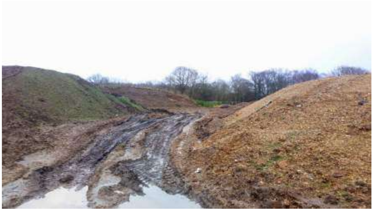
Photograph 3: Topsoil stockpile (left) and mixed materials stockpile (right), facing North.
