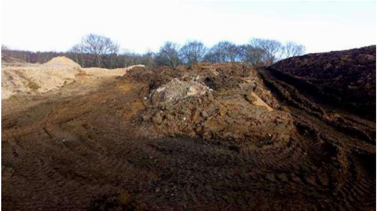
Photograph 5: Ongoing stockpiling of soils with anthropogenic contents
