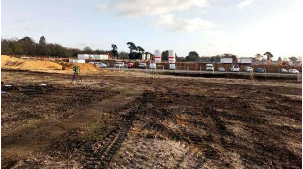
Photograph 3: View toward Taylor Wimpey Compound and parking area
