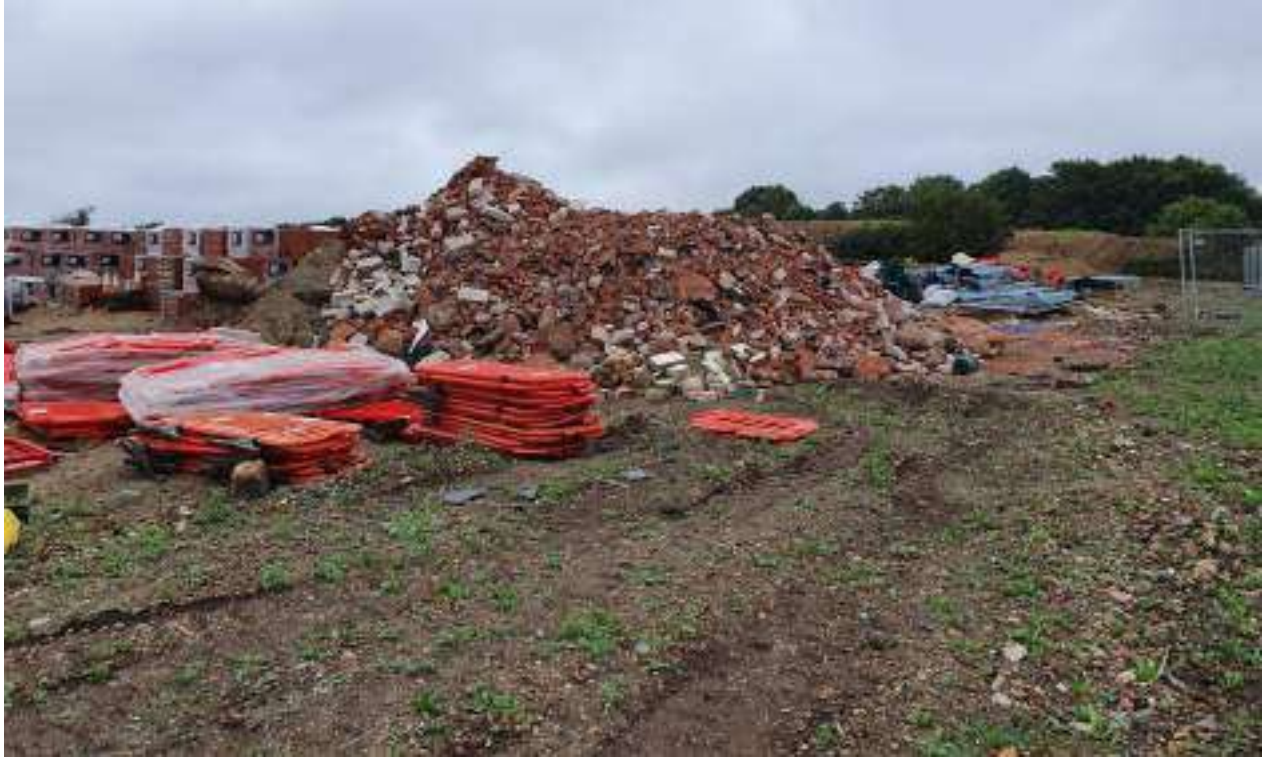
Photograph 1: Brick and block waste stockpile to west of TW compound
