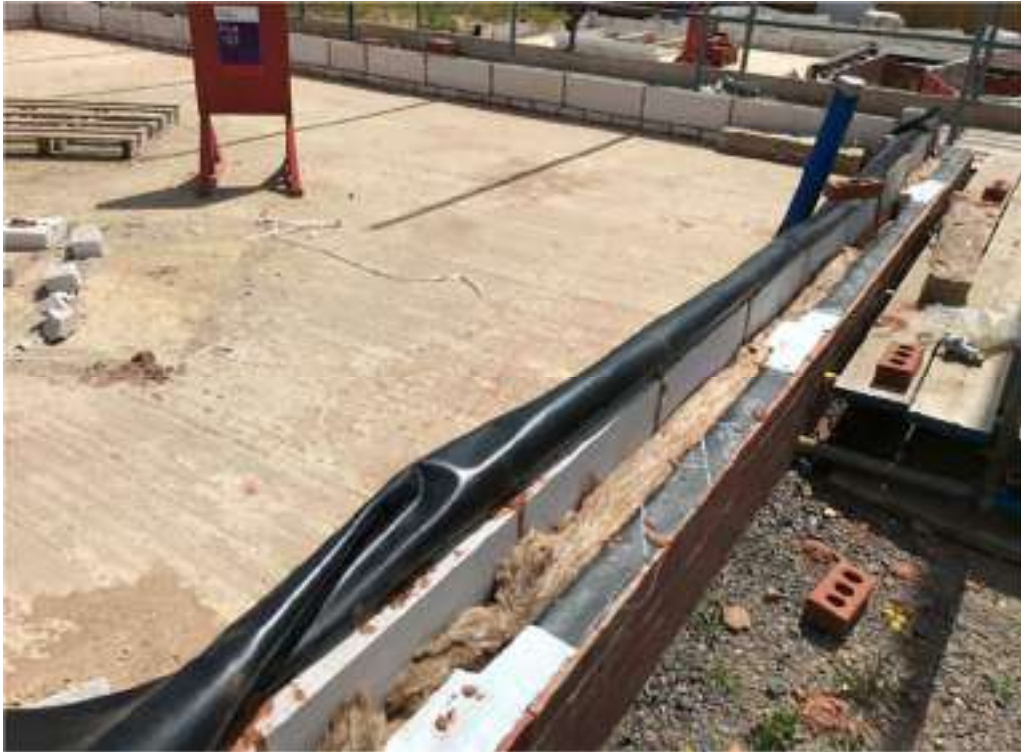
Photograph 5: Re-inspection of gas membranes P183
