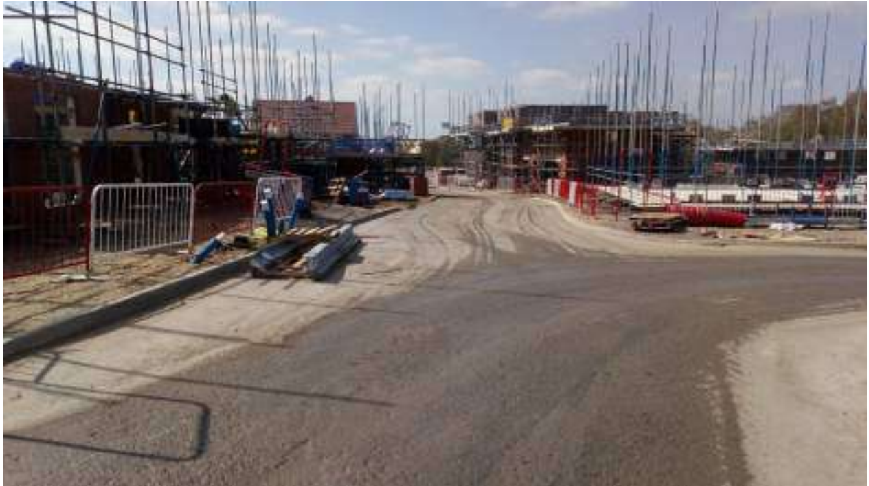
Photograph 1: Ongoing construction of houses, roadways are being wetted/cleaned for dust suppression
