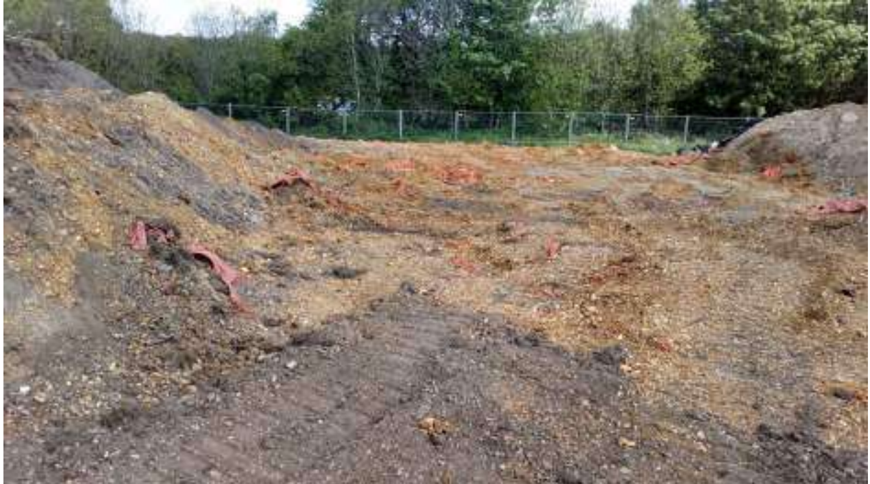
Photograph 3: Membrane evident where natural soil arising stockpiles have been utilised
