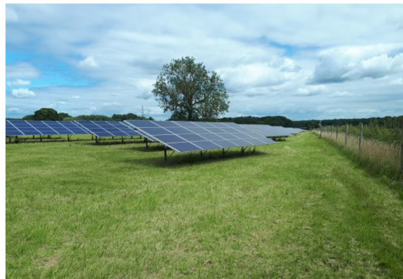
After construction (note this is an example and not the same site)
