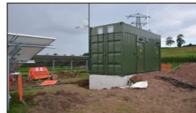
Example Substation Building (shown part way through construction)
