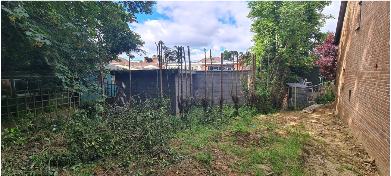
Removed Hedge Line to southern boundary opposite plot 9.
