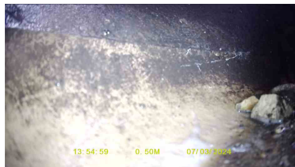
Manhole 3X_3570854f-b8d7-4fc6-a521-be4dba34f3e8_20240320_1037 52_149.jpg, 00:00:19, 0.50 m Finish node, manhole, reference: Manhole 4
