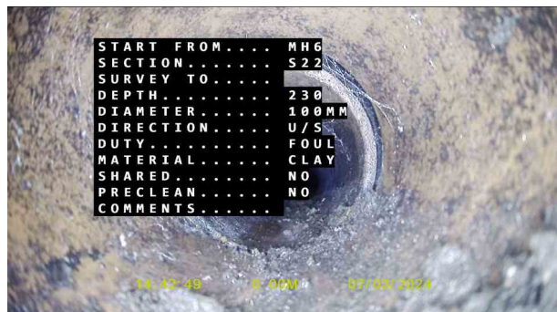
SVP 5X_4b7950ff-f199-43f0-964a-8a229e96175b_20240320_1119 50_060.jpg, 00:00:00, 0.00 m Start node, manhole, reference: Manhole 6
