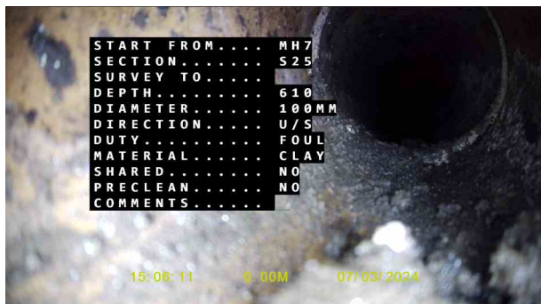
SVP 7X_a17408a8-02ab-4918-a046-8ceaf0dc9c7c_20240320_124 037_263.jpg, 00:00:00, 0.00 m Start node, manhole, reference: Manhole 7
