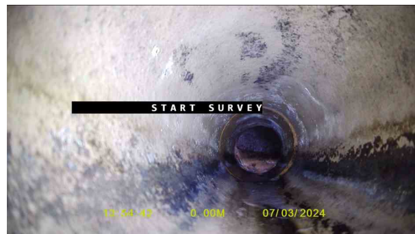
Manhole 3X_44409749-1ceb-407c-a097-f7767082c0fc_20240320_103 639_718.jpg, 00:00:03, 0.00 m Water level, 0% of the vertical dimension
