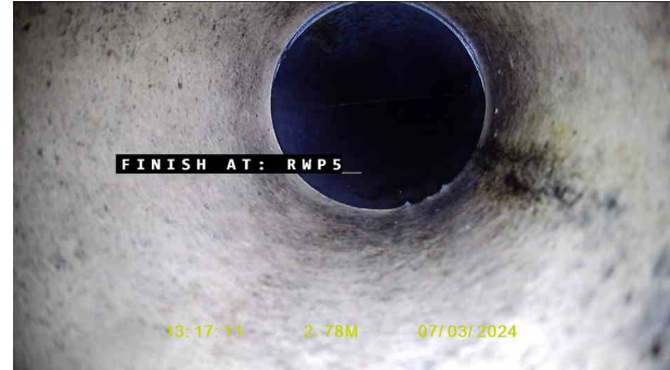
RWDP 5X_86ea2f7b-8100-4b3e-aaf7-ec7c0a68fd1f_20240320_0854 28_006.jpg, 00:01:16, 2.80 m Finish node, major connection without manhole, reference: RWDP 5
