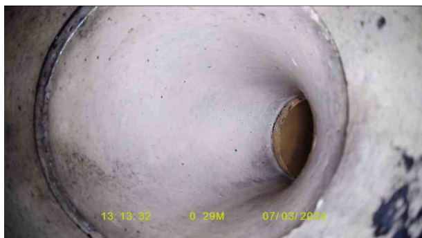
RWDP 4X_d06778ee-4b35-41b7-a975-a2ec3efeab10_20240319_170 954_011.jpg, 00:00:09, 0.29 m Line deviates right
