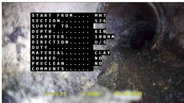
RedundantX_ee872050-97e9-48db-a77a-5383d729ed70_202 40320_124539_411.jpg, 00:00:00, 0.00 m Start node, manhole, reference: Manhole 7
