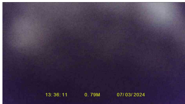
Manhole 2X_0f1934c3-d56a-465a-9667-55d40bfabd3c_20240320_095652_208.jpg, 00:00:20, 0.79 m Loss of vision, camera under water
