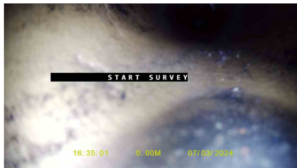
RWDP 7X_ef0e8696-c963-4252-870c-db508bc6ccf6_20240320_132 621_323.jpg, 00:00:03, 0.00 m Water level, 0% of the vertical dimension
