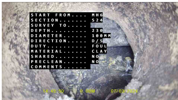
Manhole 6X_0ad92472-5a83-4a4c-a6e6-ca68686a8561_20240320_11 2927_372.jpg, 00:00:00, 0.00 m Start node, manhole, reference: Manhole 6
