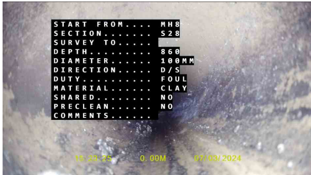
Manhole 8X_8f8dc03c-40bb-4365-b580-9e7de58ee24f_20240320_125 513_763.jpg, 00:00:00, 0.00 m Start node, manhole, reference: Manhole 8
