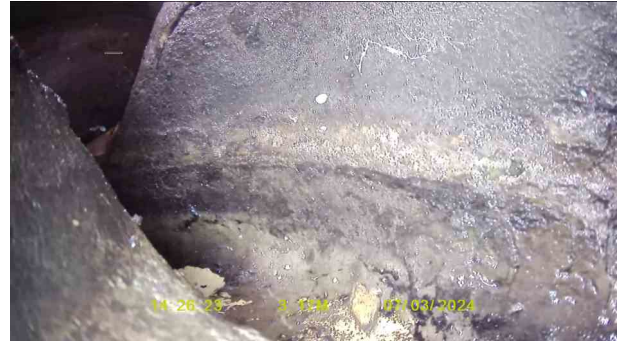
Manhole 4X_4b661bed-236d-4e69-a513-e573027e07ed_20240320_10 4618_877.jpg, 00:00:55, 3.27 m Finish node, manhole, reference: Manhole 5
