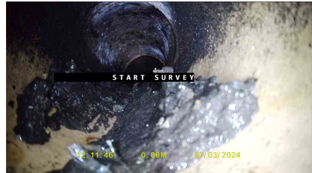
Red.Gully1X_79d8ca3a-42d2-422f-b9a8-e0b8981584cb_20240319_153744_784.jpg, 00:00:10, 0.00 m Water level, 0% of the vertical dimension
