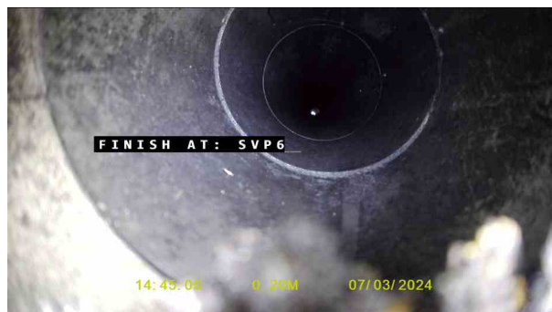
SVP 6X_d5f234bd-8a75-4c53-99d6-562c21560be6_20240320_112 646_198.jpg, 00:00:12, 0.20 m Finish node, major connection without manhole, reference: SVP 6
