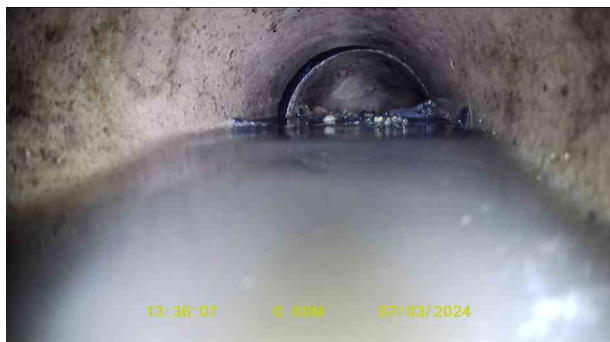
Manhole 2X_e180e7ba-86a9-4a04-bb00-ab7548002c6b_20240320_095628_250.jpg, 00:00:16, 0.69 m Water level, 30% of the vertical dimension
