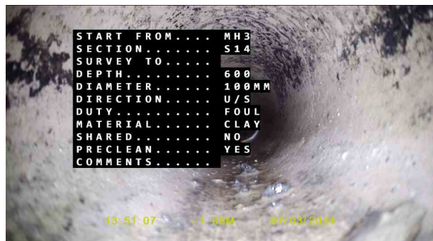
Gully 1X_e1f70322-f45c-41b0-8a61-ce2b02db6a63_20240320_102 231_744.jpg, 00:00:00, 0.00 m Start node, manhole, reference: Manhole 3
