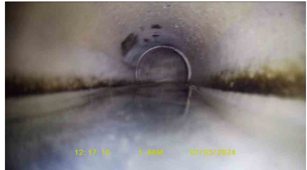
RWDP 2X_9fbec5db-38b8-4e31-b742-2a2926d9441f_20240319_154 949_655.jpg, 00:00:34, 1.88 m Water level, 20% of the vertical dimension
