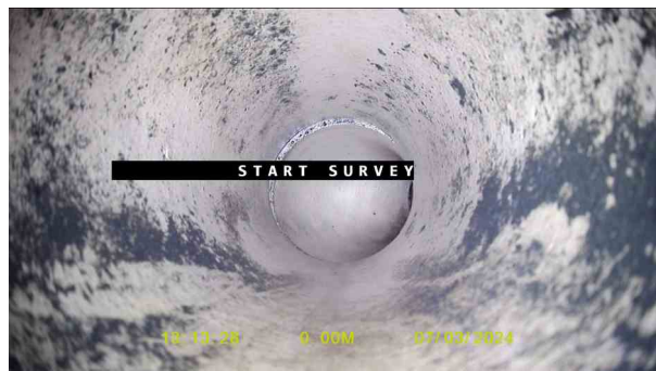
RWDP 4X_cbb82902-734f-49c9-ae6c-0771654dfc24_20240319_170 618_077.jpg, 00:00:04, 0.00 m Water level, 0% of the vertical dimension
