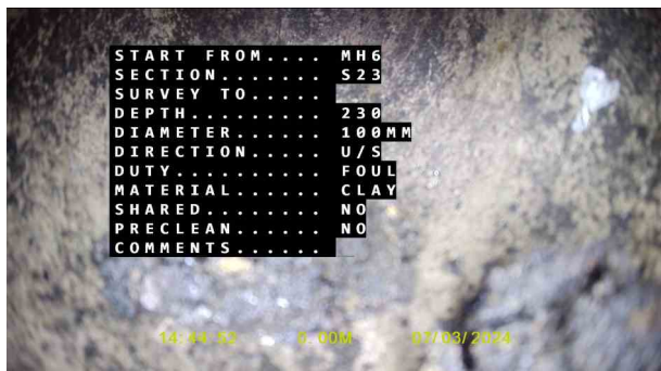
SVP 6X_2b7e16cb-5443-4afb-aa1a-eeed2f8d114c_20240320_112 602_940.jpg, 00:00:00, 0.00 m Start node, manhole, reference: Manhole 6
