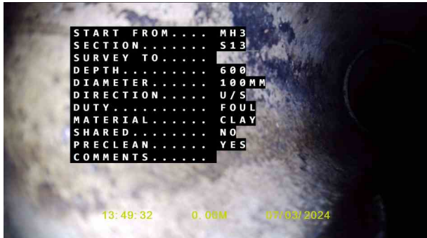
SVP 3X_c527f355-1d31-4274-a555-1137ebc4aaf2_20240320_101 019_569.jpg, 00:00:00, 0.00 m Start node, manhole, reference: Manhole 3
