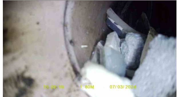
RedundantX_a6a01423-180f-4823-a742-2afe8737d258_2024 0320_124722_821.jpg, 00:00:33, 1.80 m Survey abandoned, Redundant line
