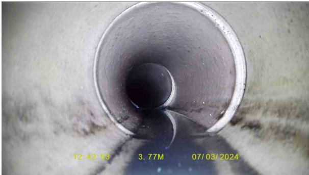
Manhole 1X_5db8b1cc-a2de-418a-80ff-518f9ca7d06b_20240319_1626 23_110.jpg, 00:00:53, 3.77 m Line deviates left
