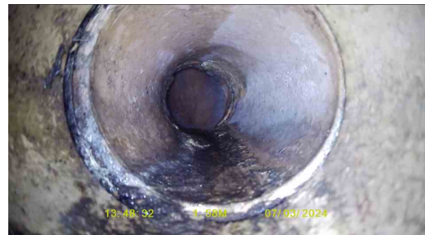
SVP 2X_a88911fc-7bdd-4968-9c5c-85725a0da2c7_20240320_100 809_241.jpg, 00:00:26, 1.49 m Open joint, medium
