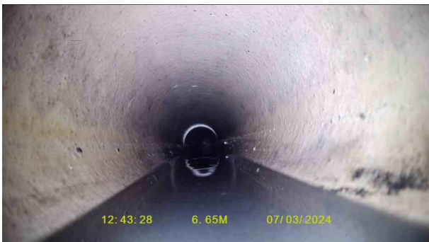
Manhole 1X_ff8504fd-99a1-47a8-8c13-b34a3054bacc_20240319_1629 17_420.jpg, 00:01:28, 6.65 m Water level, 10% of the vertical dimension
