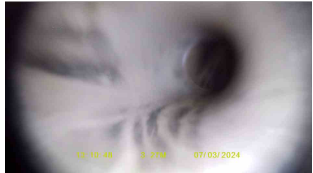
RWDP 3X_2812ae7a-d8dc-45c3-bb21-8c325102e88b_20240319_16 4108_934.jpg, 00:00:44, 3.27 m Line deviates right
