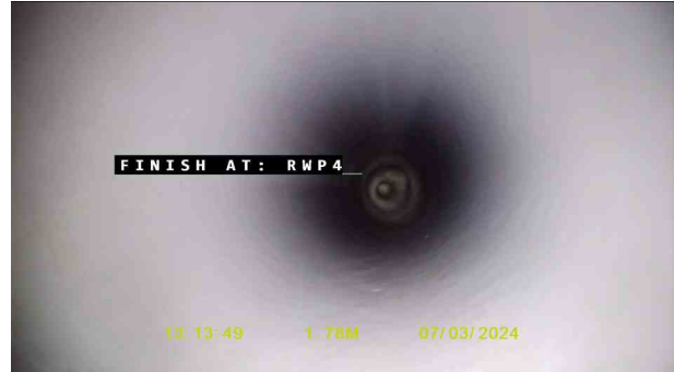
RWDP 4X_16977049-50c2-4ecb-b8d2-55b5d8572f42_20240319_171602_523.jpg, 00:00:26, 1.78 m Finish node, major connection without manhole, reference: RWDP 4
