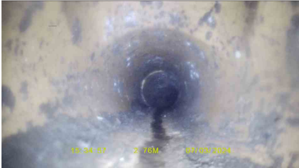
Manhole 9X_385afa2a-6e1e-4242-9b34-913fe13c0d46_20240320_131 543_709.jpg, 00:01:10, 2.76 m Junction at 12 o'clock, diameter: 100mm
