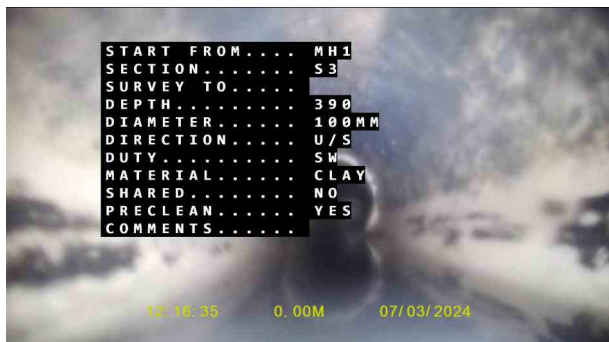
RWDP 2X_82b21668-a75d-4476-8667-1dbbfaa6c5fc_20240319_154 757_806.jpg, 00:00:00, 0.00 m Start node, manhole, reference: Manhole 1
