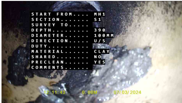
Red.Gully1X_d67abab1-b279-485c-bafa-ddca64df70fe_20240319_153734_321.jpg, 00:00:07, 0.00 m Start node, manhole, reference: Manhole 1
