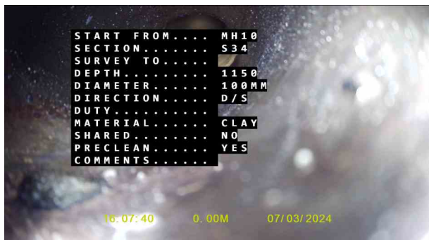
Manhole 10X_a307cee2-fd27-4e30-9867-04a519dffdc_20240320_135 245_772.jpg, 00:00:00, 0.00 m Start node, manhole, reference: Manhole 10
