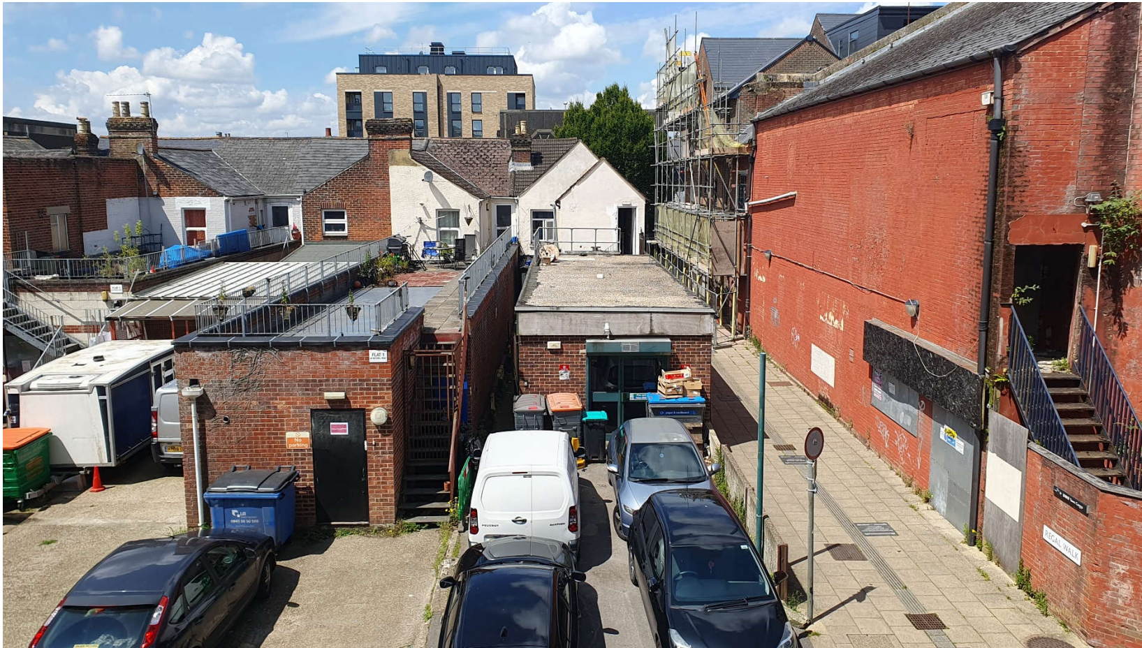
Figure 8 Rear of Oishii showing amenity space and residential use at upper levels
