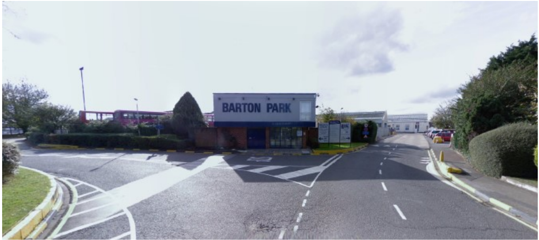
Figure 1 Existing Security Hut
