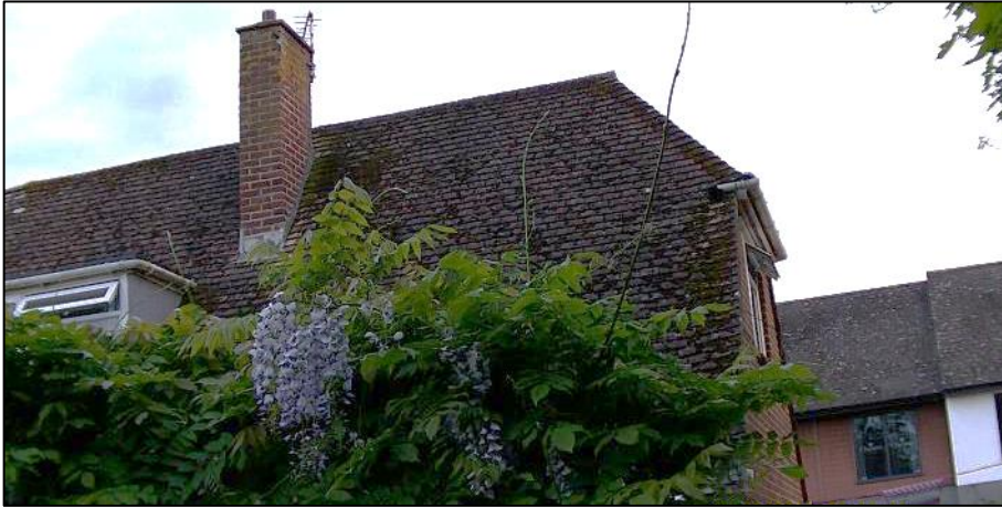
NVA 1 view at the start of the survey (pictured opposite)
