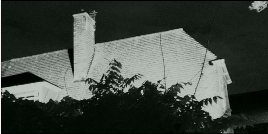
NVA 1 view at the end of the survey (pictured opposite)
