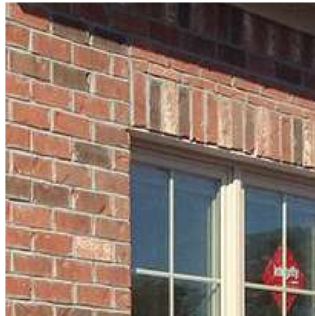
Brickwork window head
