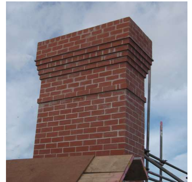
Corbelled Brickwork Chimney Stacks
