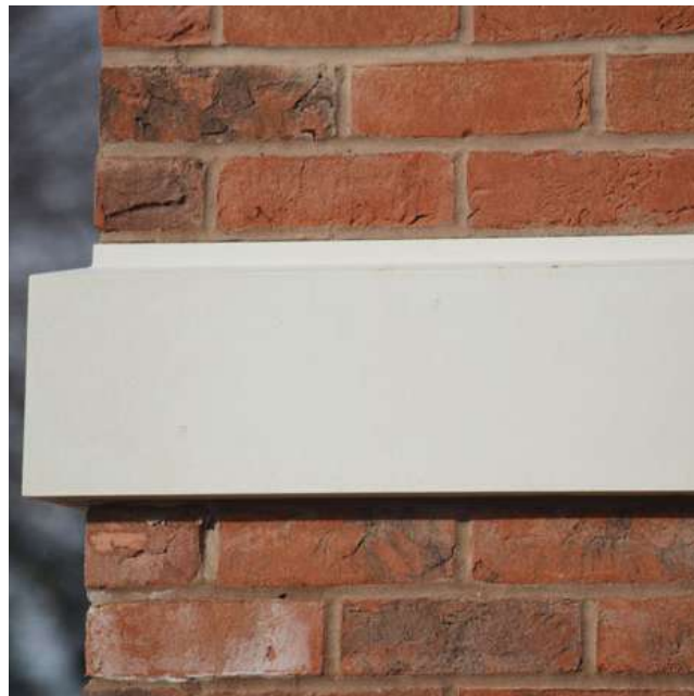
Stonework String Coursing
