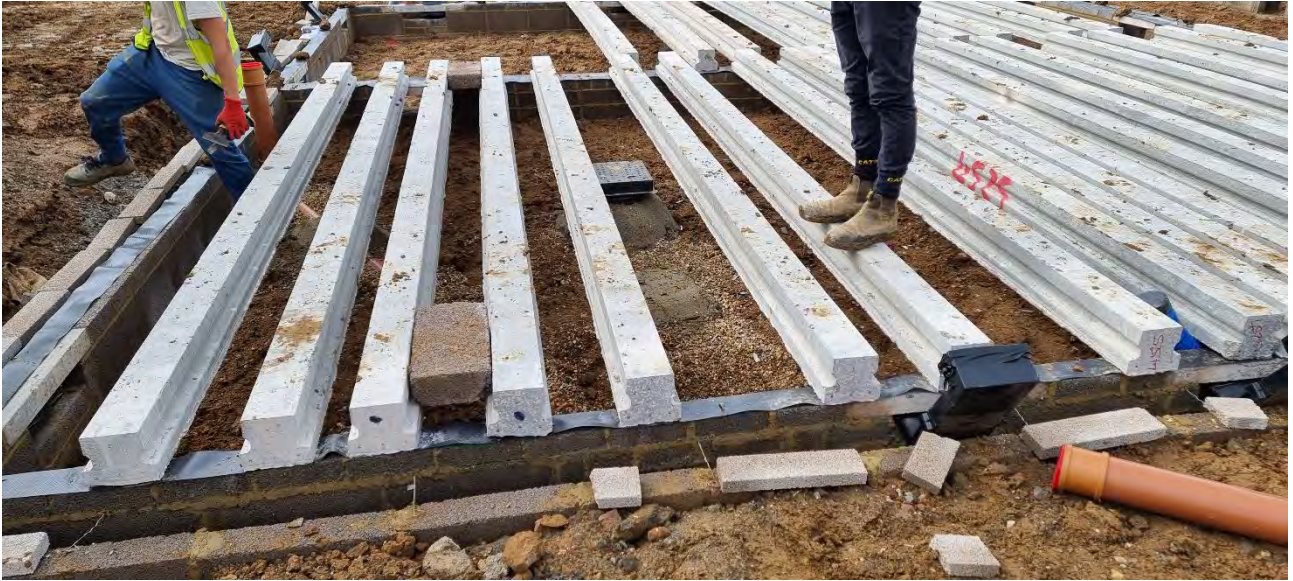
Plate 1 View of sub-floor void construction – Block B
