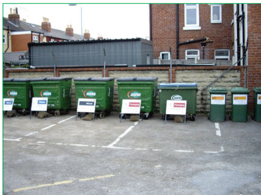
Figure 4.48 Segregated skips (courtesy BAM Nuttall)
