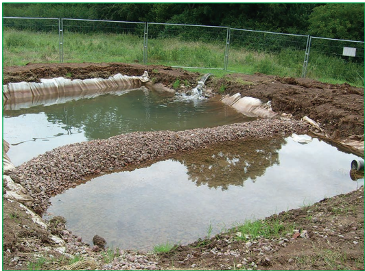
Figure 4.64 Settlement lagoon (courtesy Galliford Try plc)
