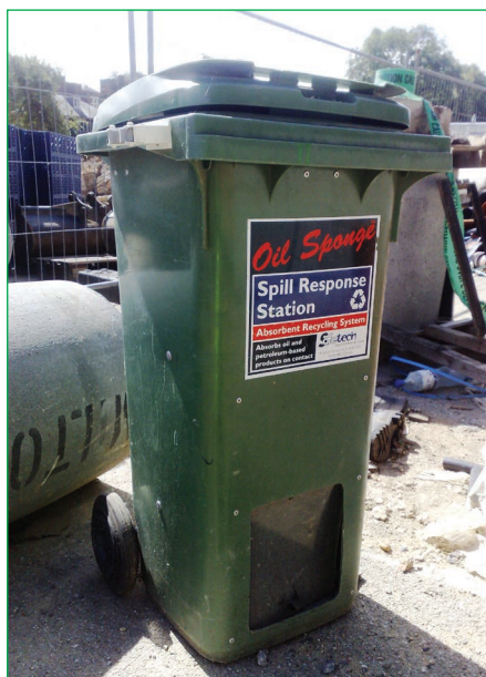
Figure 3.12 Spill response station (courtesy BAM Nuttall)
