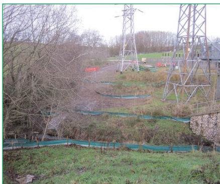
Figure 4.59 Silt fencing
