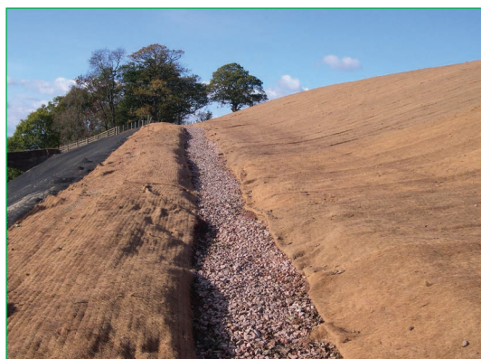
Figure 4.56 Drainage installation and silt management (courtesy BAM Nuttall)
