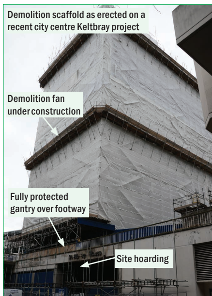
Figure 4.30 Noise and dust mitigation (courtesy Brookfield Multiplex and Keltbray)
