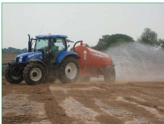
Figure 4.29 Dust suppression (courtesy Galliford Try plc)
