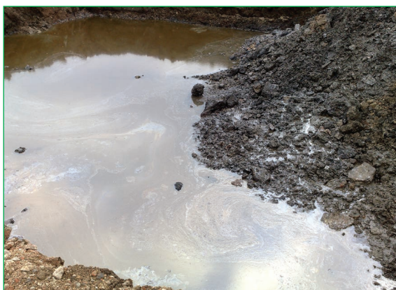
Figure 4.26 Discovery of contaminated land (courtesy BAM Nuttall)
