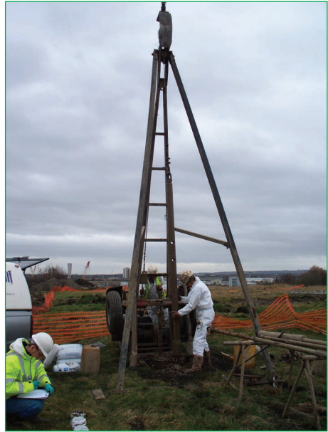
Figure 4.25 Soil testing being undertaken (courtesy Parsons Brinckerhoff)
