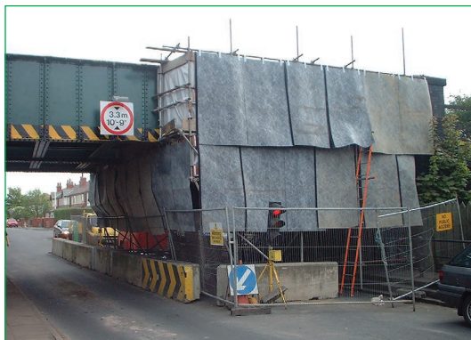
Figure 4.32 Acoustic screening (courtesy BAM Nuttall)
