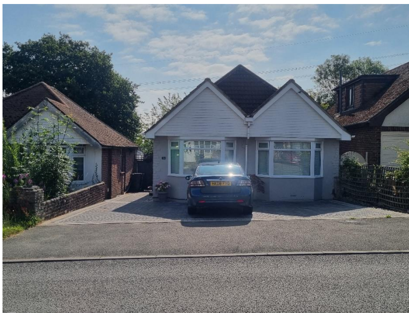
31 Belmont Road, single storey rear & roof extension Raised roof, Raised bay gable height, roof pitch change. Planning Reference: Z/39519/000/00 (2003)
