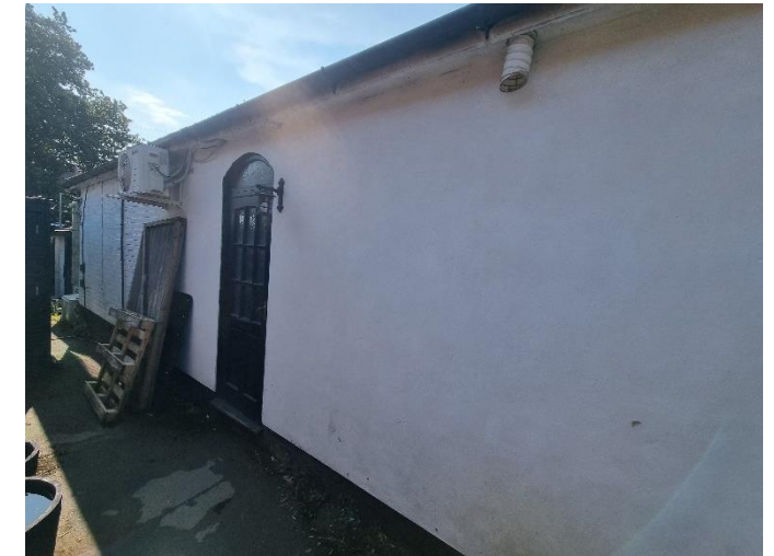
Side façade of 29 Belmont Road facing North
