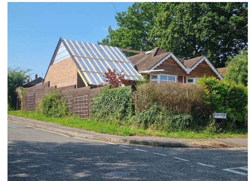
Corner of Belmont Rd & Cox Row, single storey side & rear extension Large gable end extension, with scope to convert the roof void. Planning Reference: F/14/74551 (2014)
