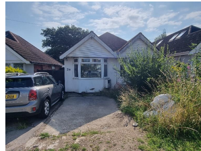
Front façade of 29 Belmont Road facing West
