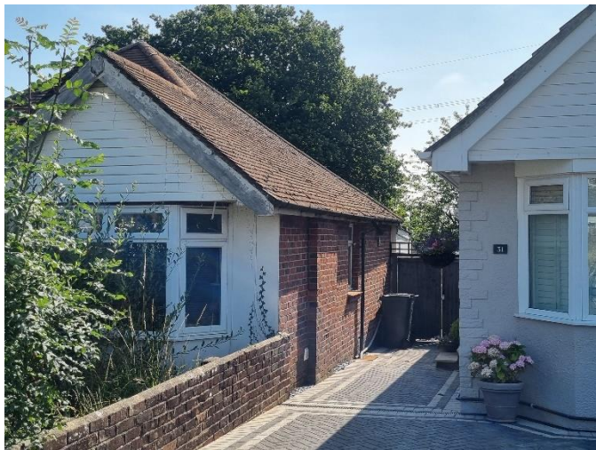
Side façade of 29 Belmont Road facing South
