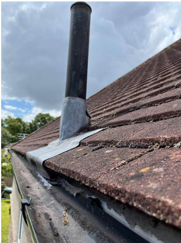
Figure 6 - Close up of roof
