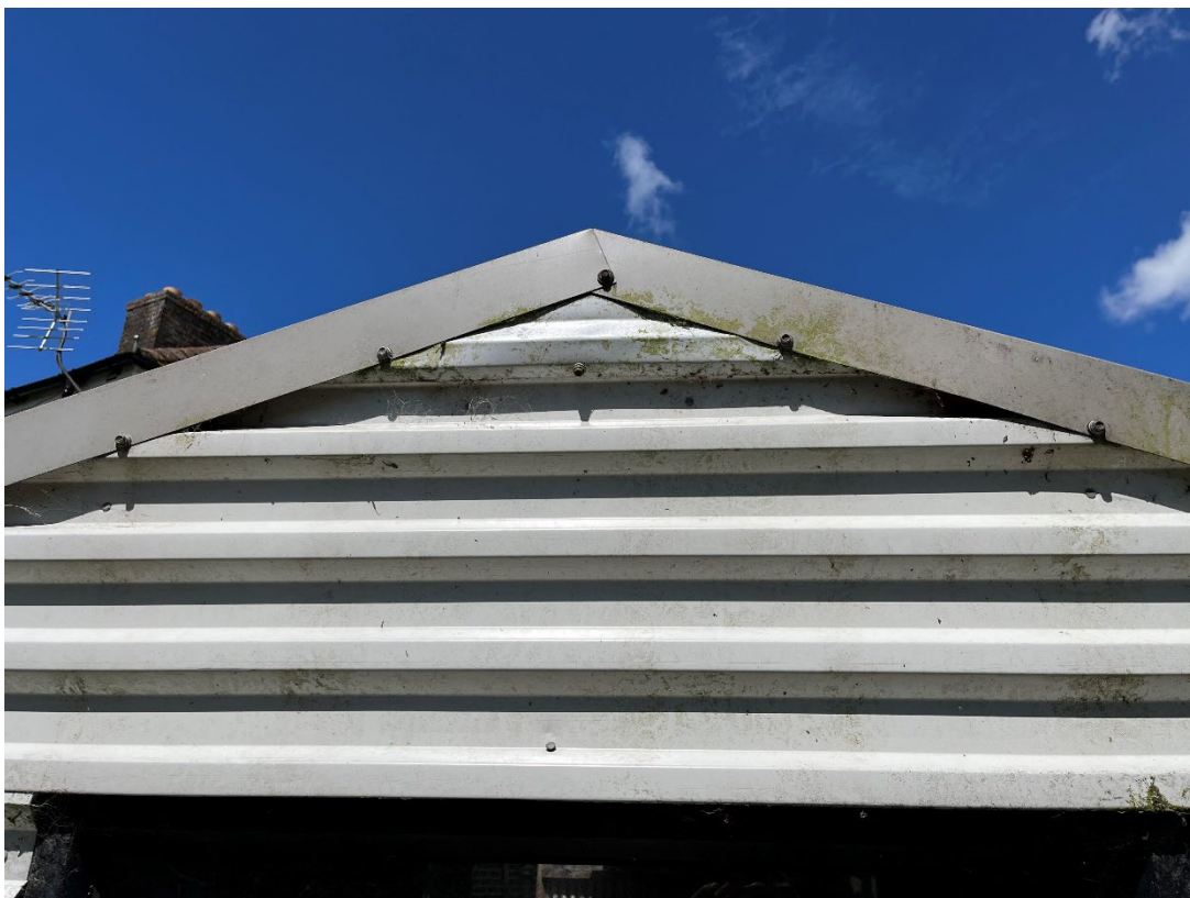
Figure 8 - Close up of garage outbuilding roof
