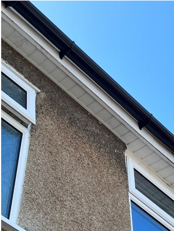
Figure 5 - Front soffit and fascia
