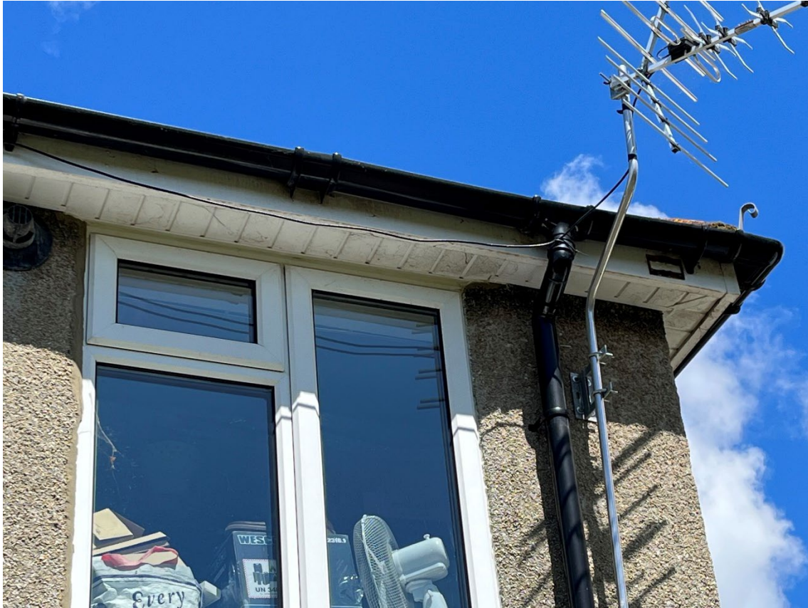
Figure 2 - Rear soffit and fascia
