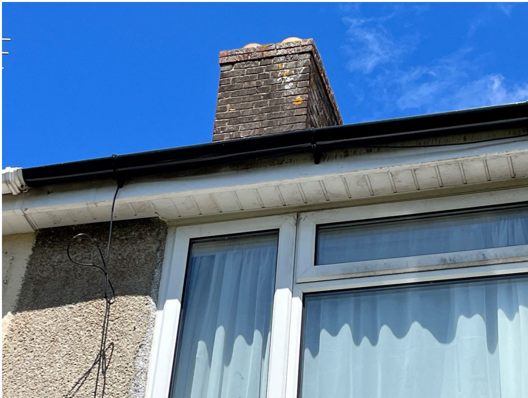
Figure 1 - Rear soffit and fascia
