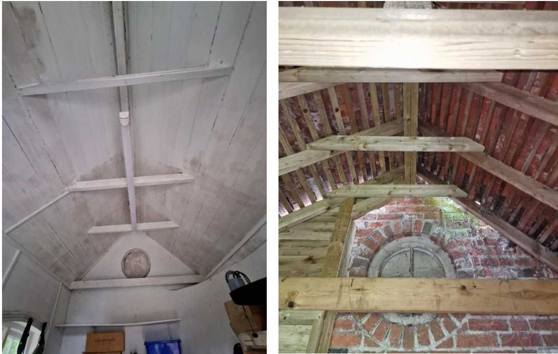
Photo 2: Internal views of the roof of each half of the outbuilding
