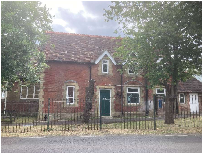
Fig. 1 – Photograph showing the north-west elevation of the building with the entrance door to the first-floor office.
