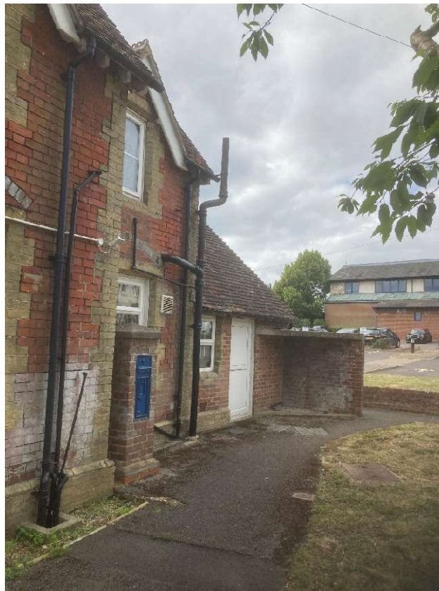
Fig. 2 – Photograph showing the proposed bin storage area on the north-west elevation of the building close to the entrance door to the first-floor office.
