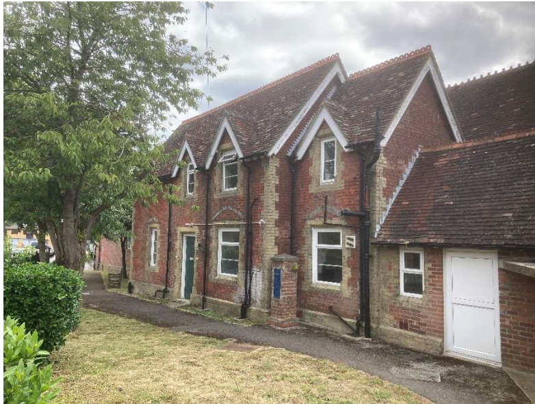
Fig. 3 – Photograph showing the north-west elevation of the building with the entrance door to the first-floor office and proposed bin storage (far right).
