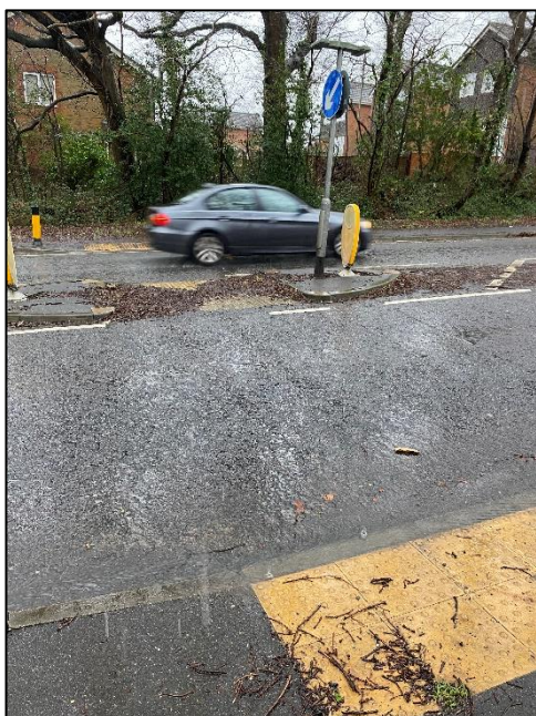
Photograph 3: Existing pedestrian infrastructure along Providence Hill
