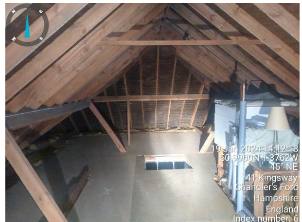
Photograph 24: View within bungalows loft looking north.
