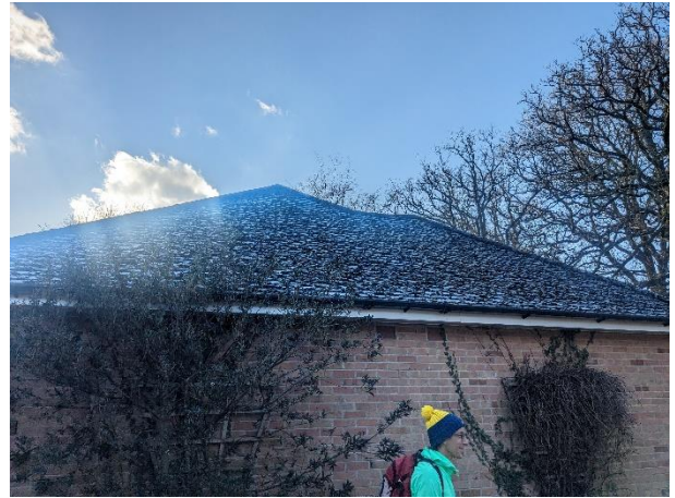
Photograph 2: View of the north-west elevation roof.
