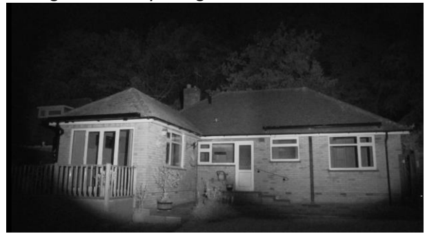
Photograph 36: View of the rear of the property on 18/06/2024 at the end of the dusk emergence survey using NVAs.
