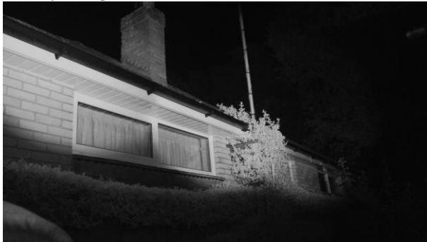
Photograph 33: View of the side of the property on 27/05/2024 at the end of the dusk emergence survey using NVAs.
