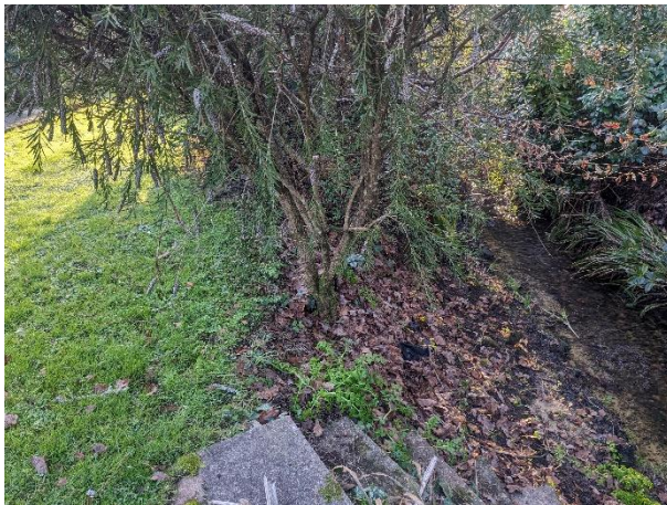
Photograph 9: View of the wet ditches eastern flank embankment
