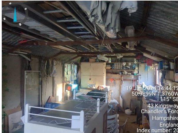
Photograph 19: View of the interior of the garage.
