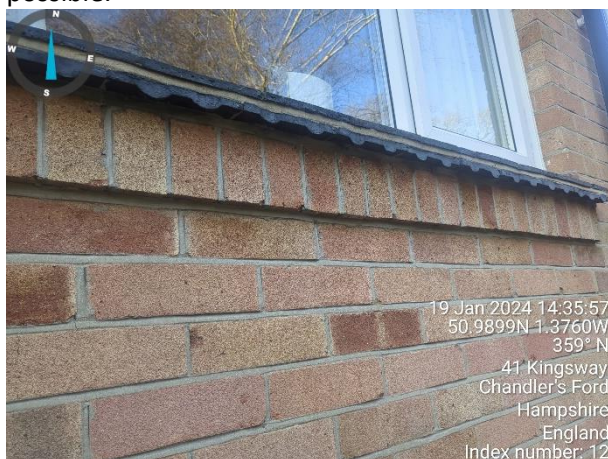
Photograph 15: Example view beneath a window frame of no missing mortar and no gaps for bats to access a cavity.
