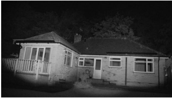
Photograph 31: View of the rear of the property on 27/05/2024 at the end of the dusk emergence survey using NVAs.
