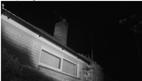
Photograph 35: View of the side of the property on 18/06/2024 at the end of the dusk emergence survey using NVAs.
