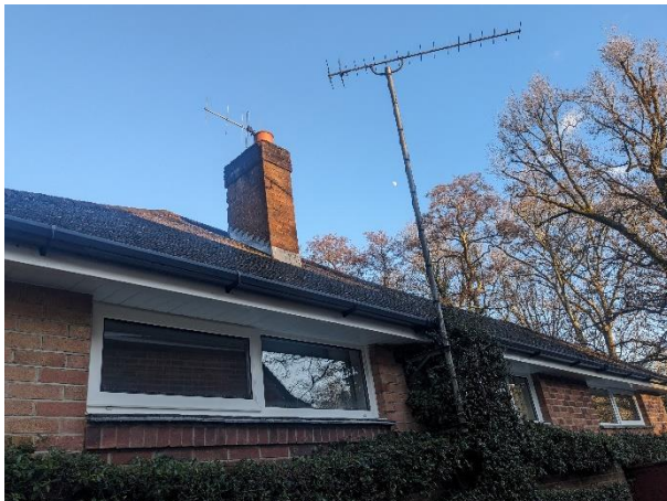
Photograph 11: View of the south-west roof elevation, within the only spot within the plot where it is visible.
