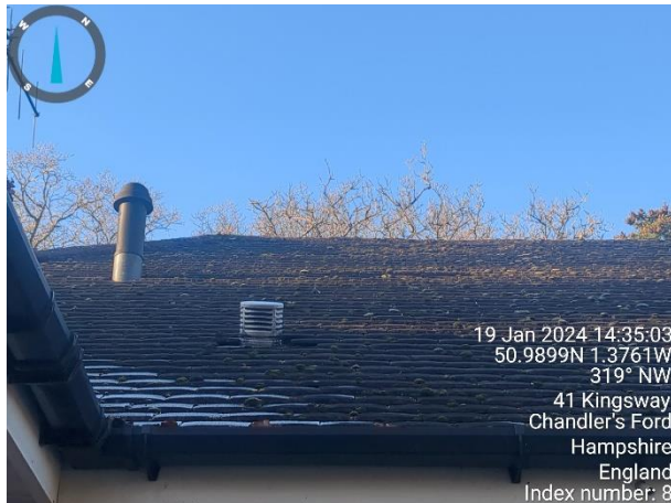
Photograph 13: View of the flues where bat access to the loft from underneath surrounding tiles is possible.
