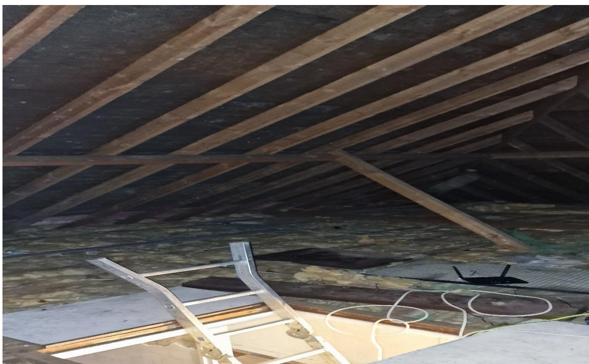
Picture 4: Showing the internal structure of the roof and the bitumen felt..
