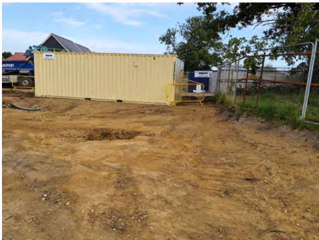
Description Area C reduced dig
