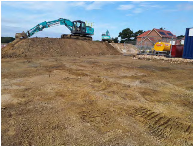
Description Reduced dig Area C
