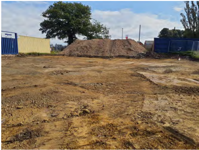
Description Reduced dig Area C
