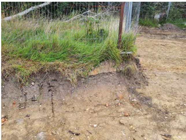
Description Area C reduced dig
