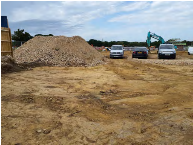
Description Area C reduced dig
