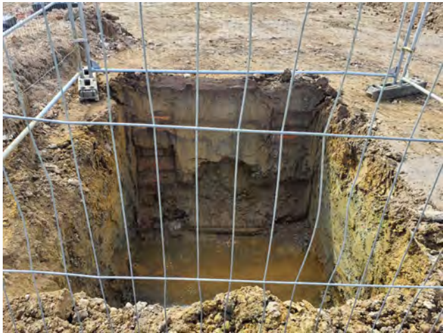
Description Area C tank
