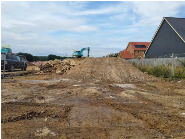
Description Reduced dig Area D
