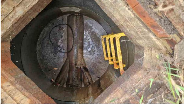
S23A__TANK 4 (A)_12.jpg, 00:00:00, 0.00 m Start node, manhole, reference: S23A
